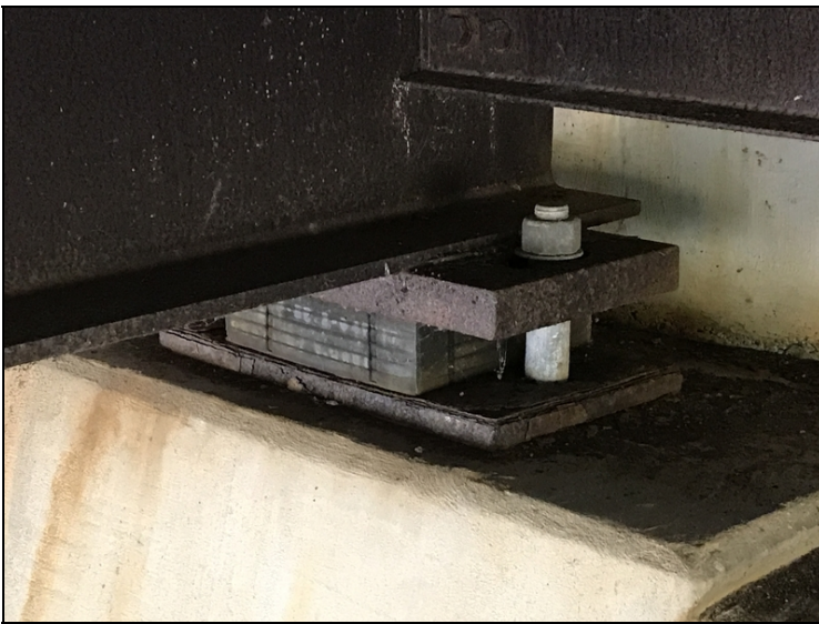
Typical corrosion with laminations on abutment #1 bearings
