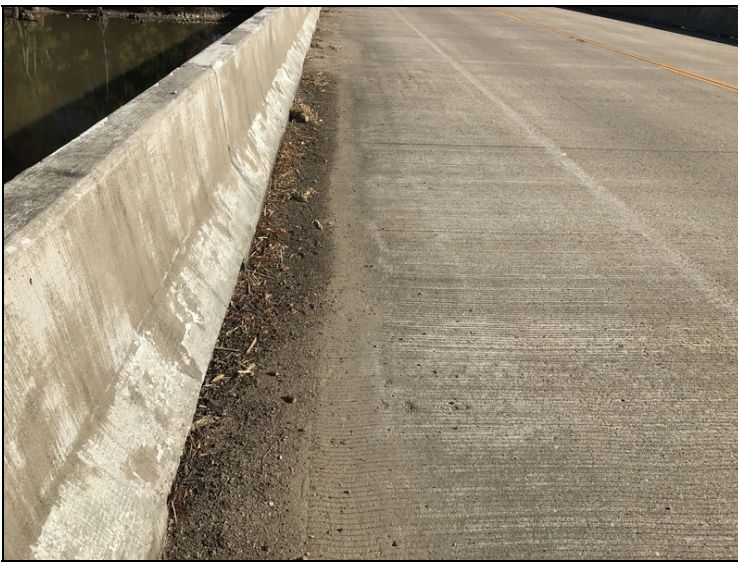
Dirt and debris in gutters
