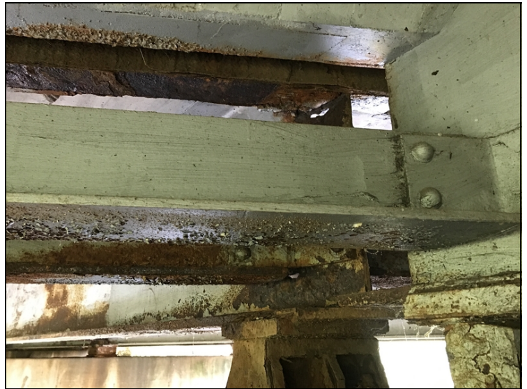
Bent #2 span #2 girder #2 corrosion at haunch and diaphragm connections with a two inch hole at diaphragm and a three inch hole at haunch.
