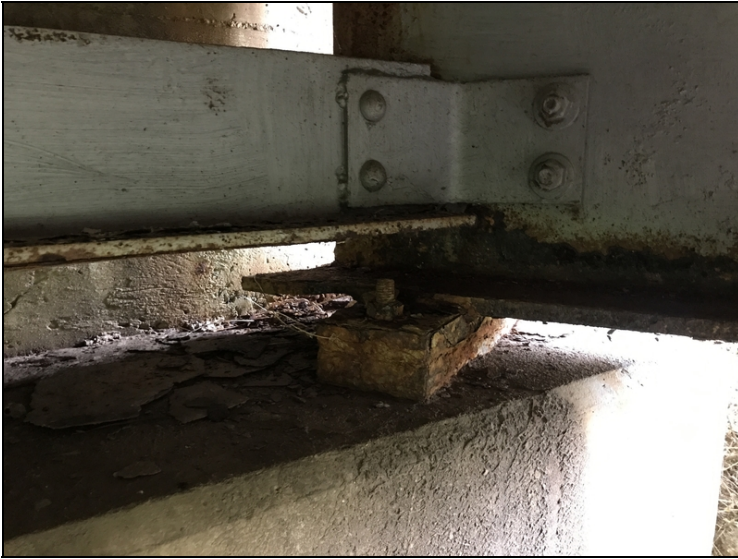
Abutment #2 girder #4 bottom flange has 25% section loss last one foot.
