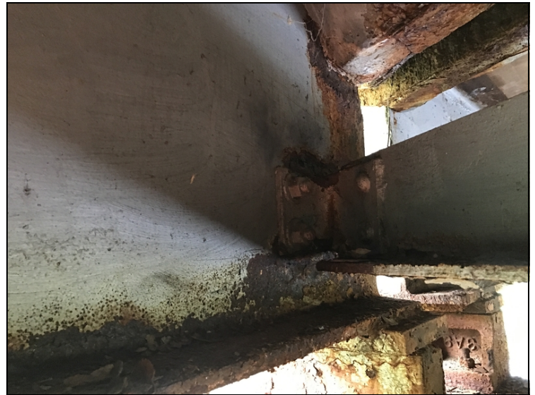
Bent #2 girder #1 span #1 corrosion at haunch and diaphragm connections with 70% sect. loss.
