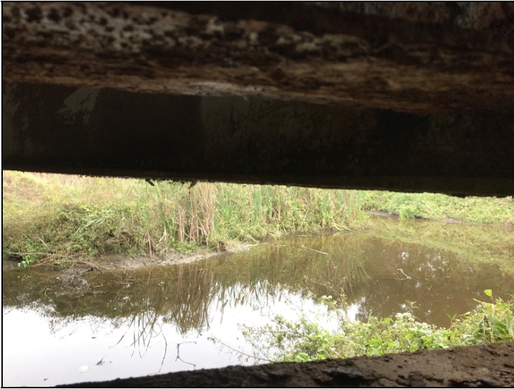
Bent #2 span #2 girder #4 has first 2' long area bottom flange inside with up to 50% section loss.
