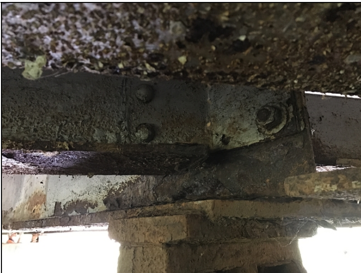
Bent #2 span #2 girder #3 corrosion at haunch and diaphragm connections with a small hole under diaphragm.
