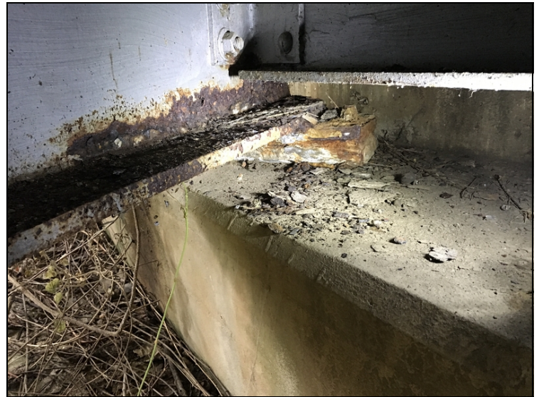
Abutment #1 girder #4 lower flange and lower web at lower flange has corrosion with laminations and section loss up to 25% for two feet.
