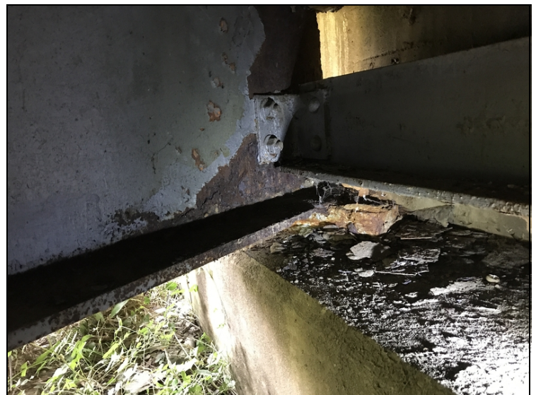
Abutment #2 girder #1 bottom flange into the lower web has up to 75% section loss for first foot of girder both sides.
