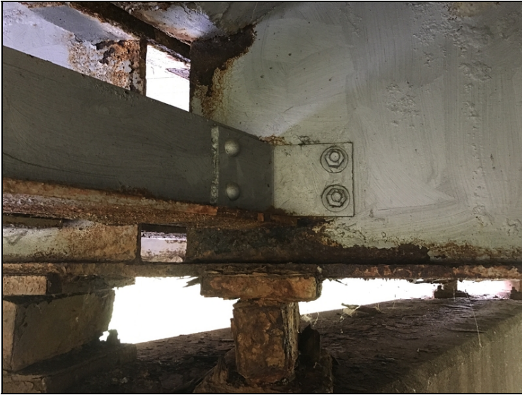
Bent #3 span #3 girder #2 corrosion at haunch and diaphragm connections with 70% sect. loss.
