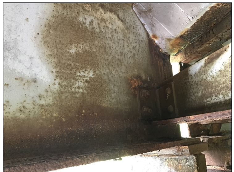
Bent #3 girder #1 span #2 corrosion at haunch and diaphragm connections with 60% sect. loss.
