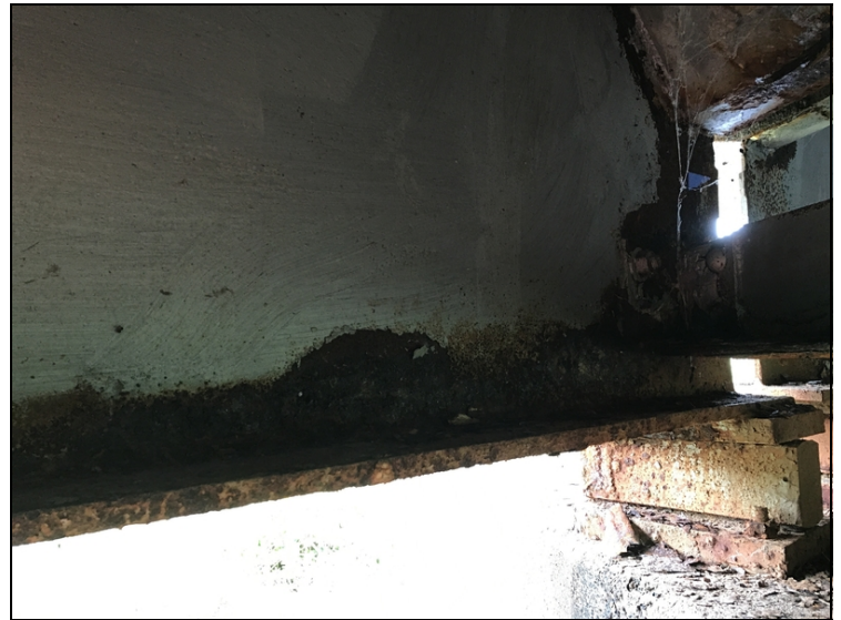
Bent #3 span #3 girder #4 corrosion at haunch and diaphragm connections with 70% sect. loss.
