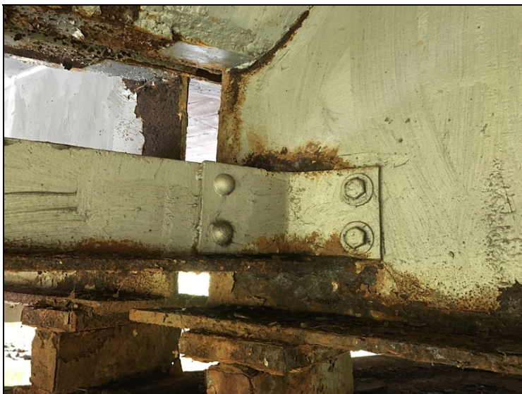
Bent #3 span #3 girder #3 corrosion at haunch and diaphragm connections with 70% sect. loss.
