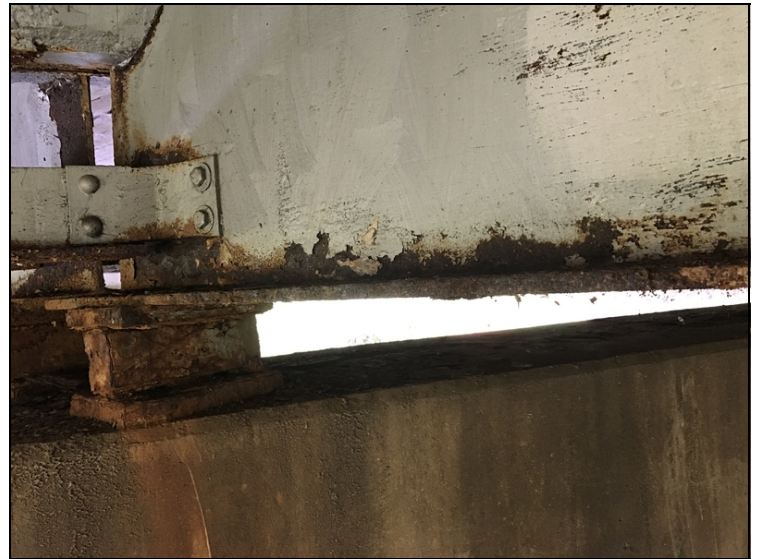
Bent #3 span #3 girder #3 lower flange first 2' corroded & laminated with section loss up to 20%.
