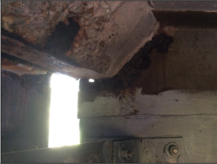
Bent 3 girder 1 span 3 has section loss up to 80% around haunch with small hole.
