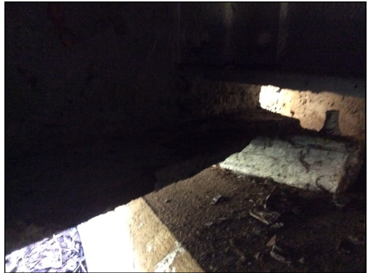
ABUTMENT # 2 GIRDER #1 LOWER FLANGE FOR FIRST 2' HAS SECTION LOSS UP TO 75% GROWING INTO WEB.
