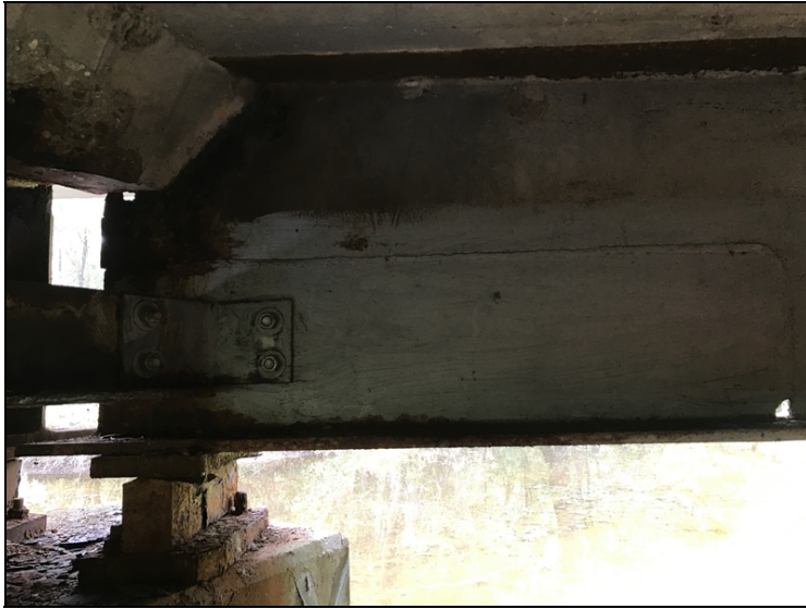
Bent #3 girder #1 span #3 has section loss up to 80% around haunch with small hole. Girder has been t-spliced for one foot tall three feet long.
