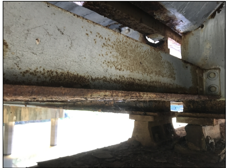
Span #3 bent #3 girder #2 has hole in web six inches long at haunch and up to 50% section loss in web around diaphragm.
