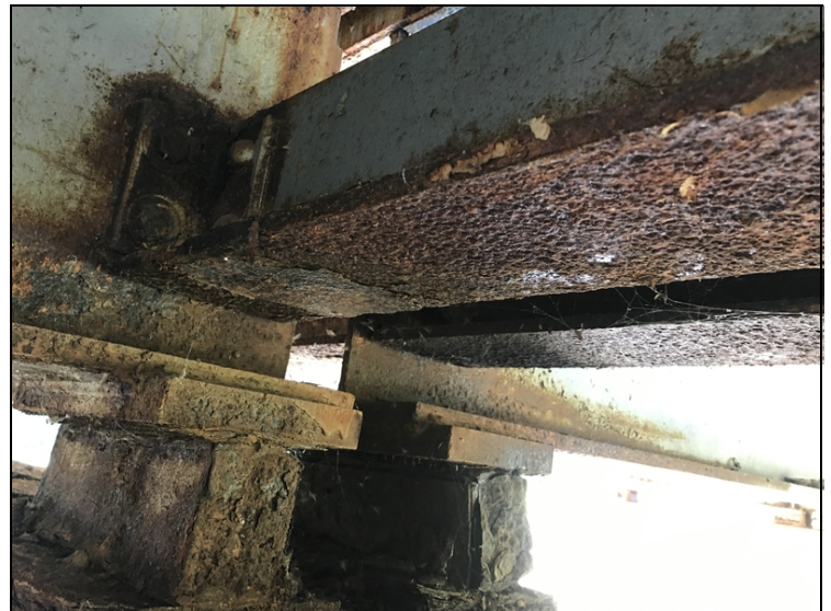
Span #4 bent #5 bearing #2 is rocked forward.
