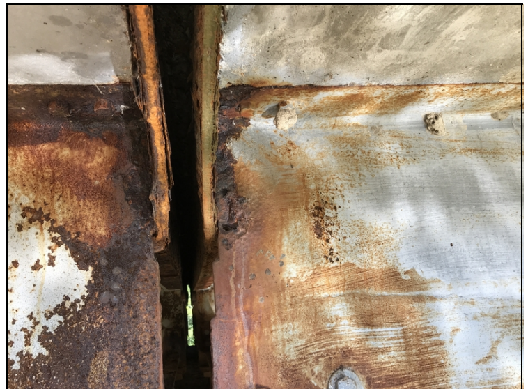
Span #4 bent #4 girder #4 has a one inch hole in web at haunch with rest of web at haunch with up to 75% section loss.
