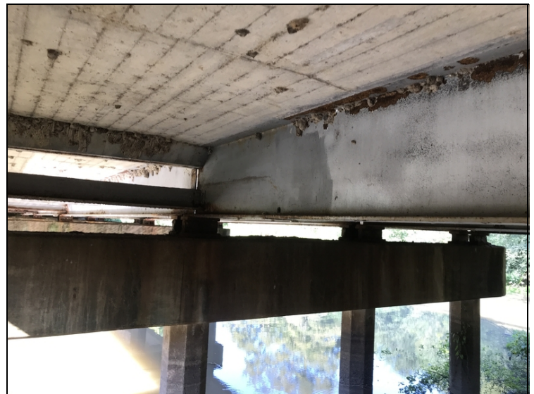
Typical paint condition inside girder.
