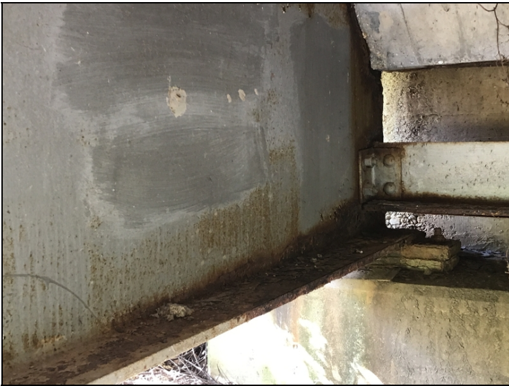
Typical outside girder condition.
