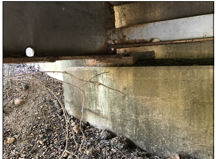
Typical abutment bearing
