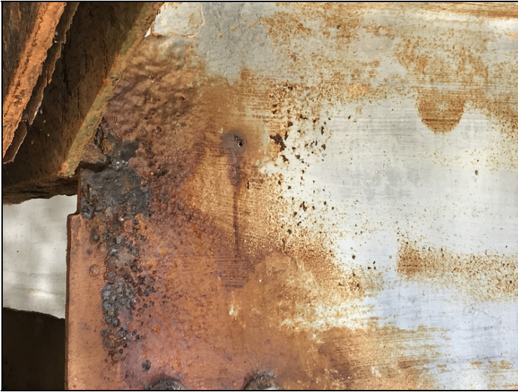
Span #3 bent #3 girder #4 has section loss with small pin hole and one inch hole at haunch.
