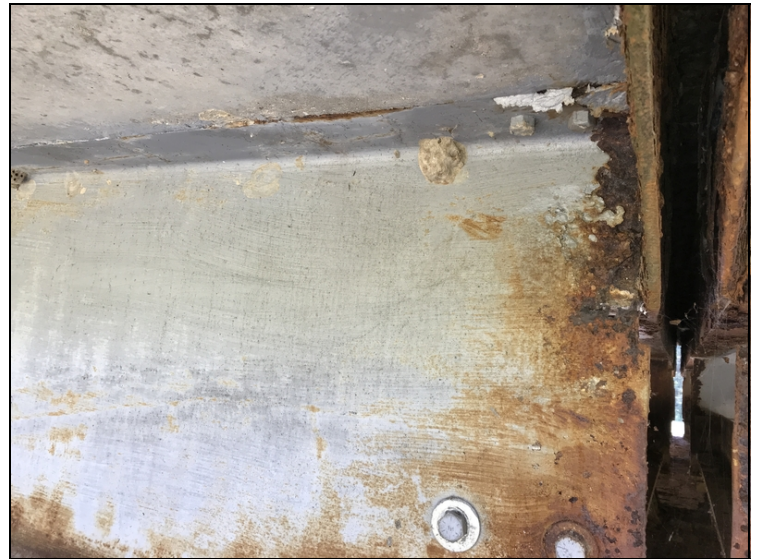
Span #4 bent #4 girder #1 has a one inch long hole in web at haunch rest of web around haunch has section loss up to 75%.
