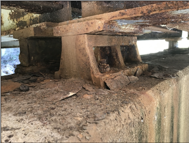
Typical fixed bearing condition.
