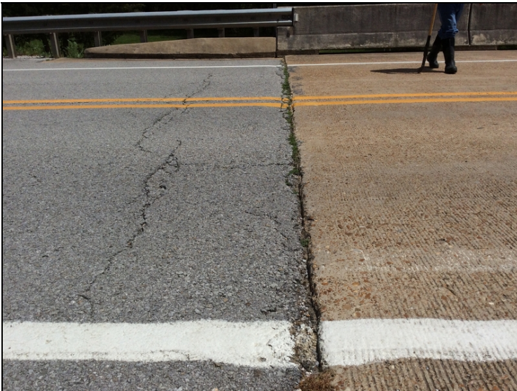
Approach roadway settlement @ Abutment 1.
