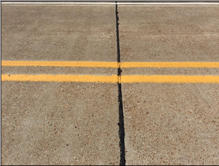
Pourable joint seal over Bent 2.
