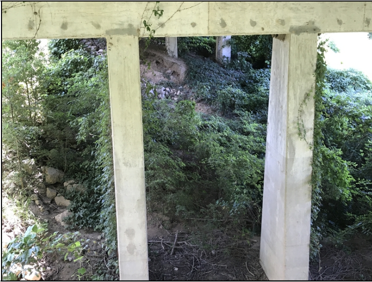
Span #2 erosion
