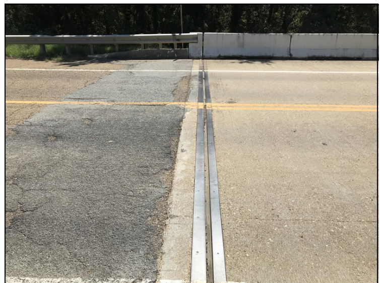
Abutment #2 seal has two one inch holes in the right lane and shoulder.
