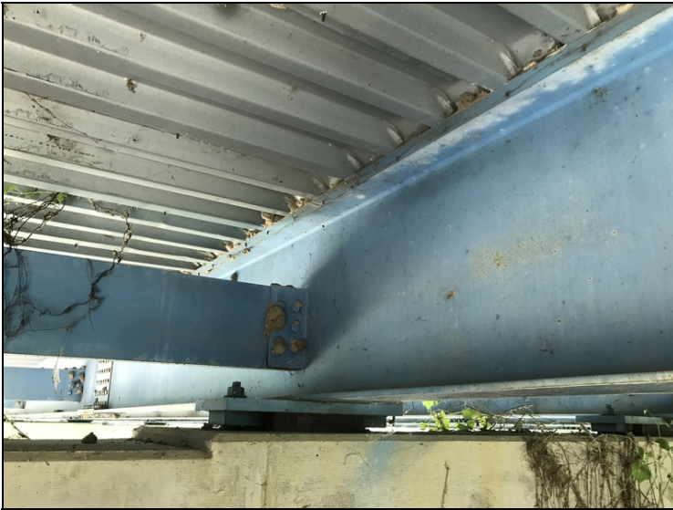
Typical interior girder paint condition
