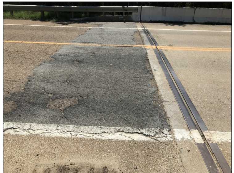
Abutment #2 approach roadway has been repaired since last inspection.
