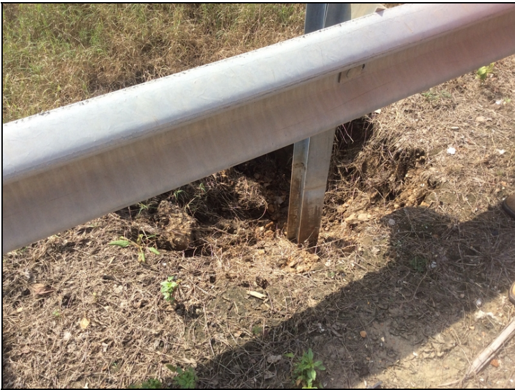
Abutment #2 approach rail right side fourth feet from bridge end has three foot deep hole around rail post.
