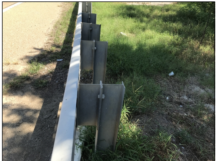
Abutment #2 right approach rail hole around post has been filled in since last inspection.
