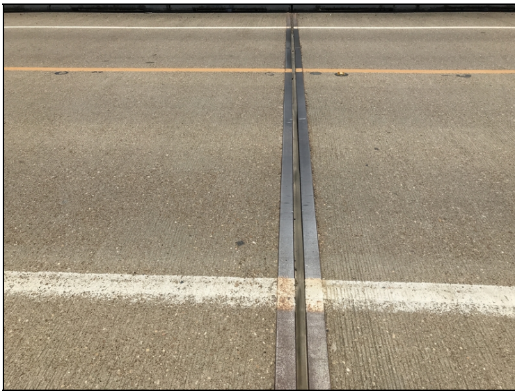
Bent #5 seal has lost adhesion for one foot in left lane.
