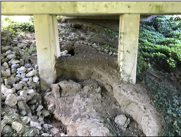
Span #1 slope erosion
