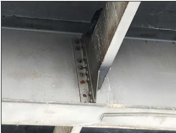
Typical diaphragm nuts missing
