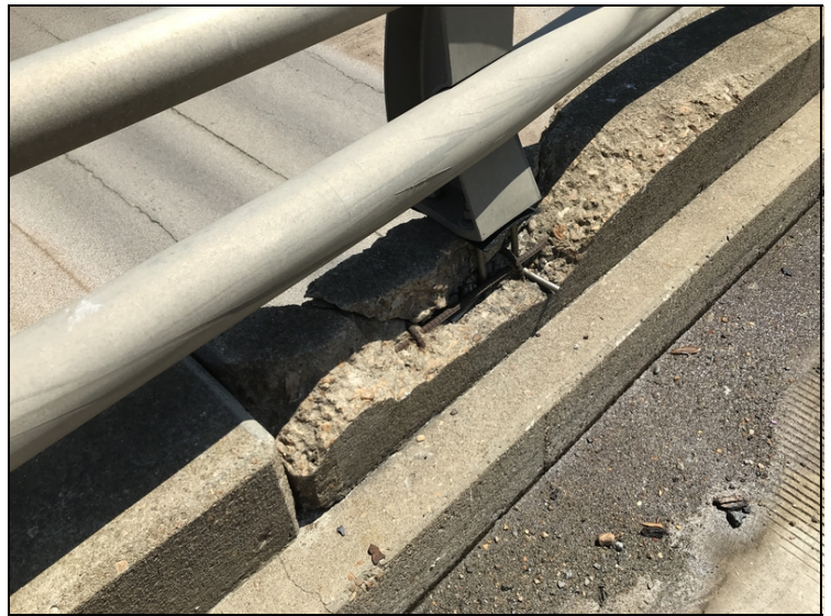
Span #4 right side concrete bridge rail has 2' spall exposed rebar due to collision damage.
