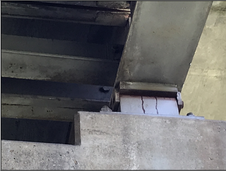
Typical missing girder to bearing bolt.
