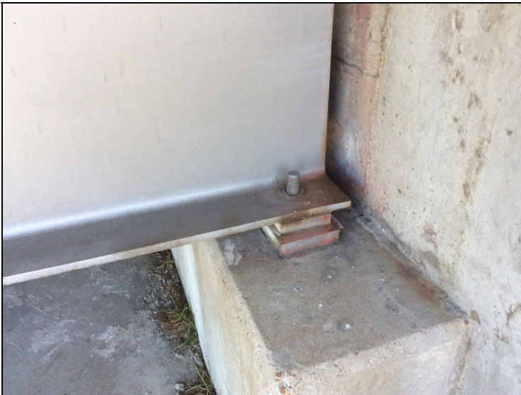
Typical bearing nut missing.
