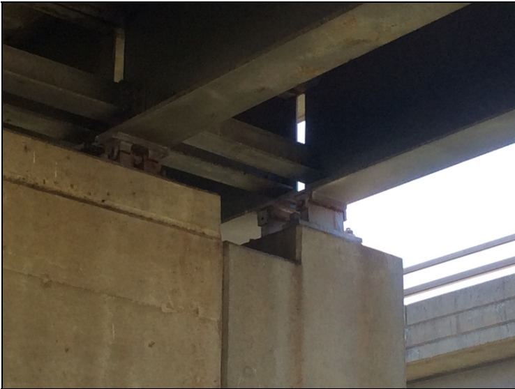
Typical bearing to girder bolt missing.
