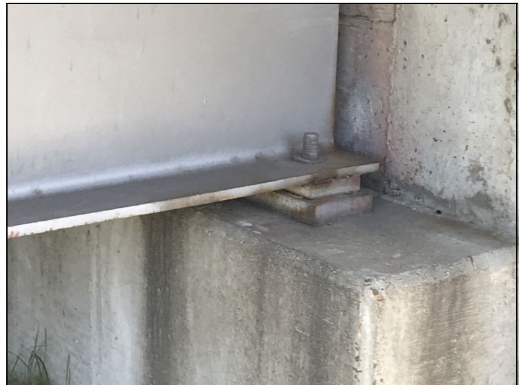
Typical abutment bearing nut missing.
