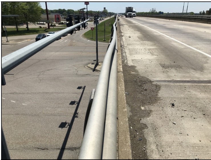
Right aluminum bridge rail has collision damage in spans #4,5,6.
