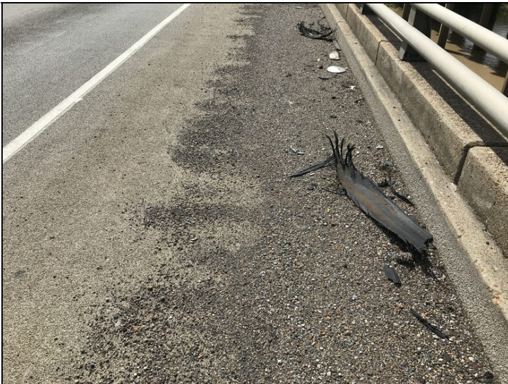
Typical deck debris in gutters
