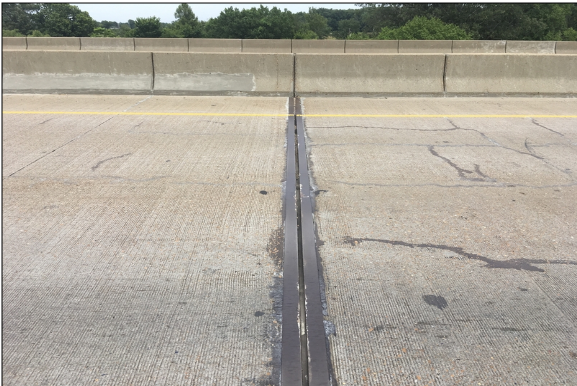
Span 4, Pourable Joint: Sag with minor leakage
