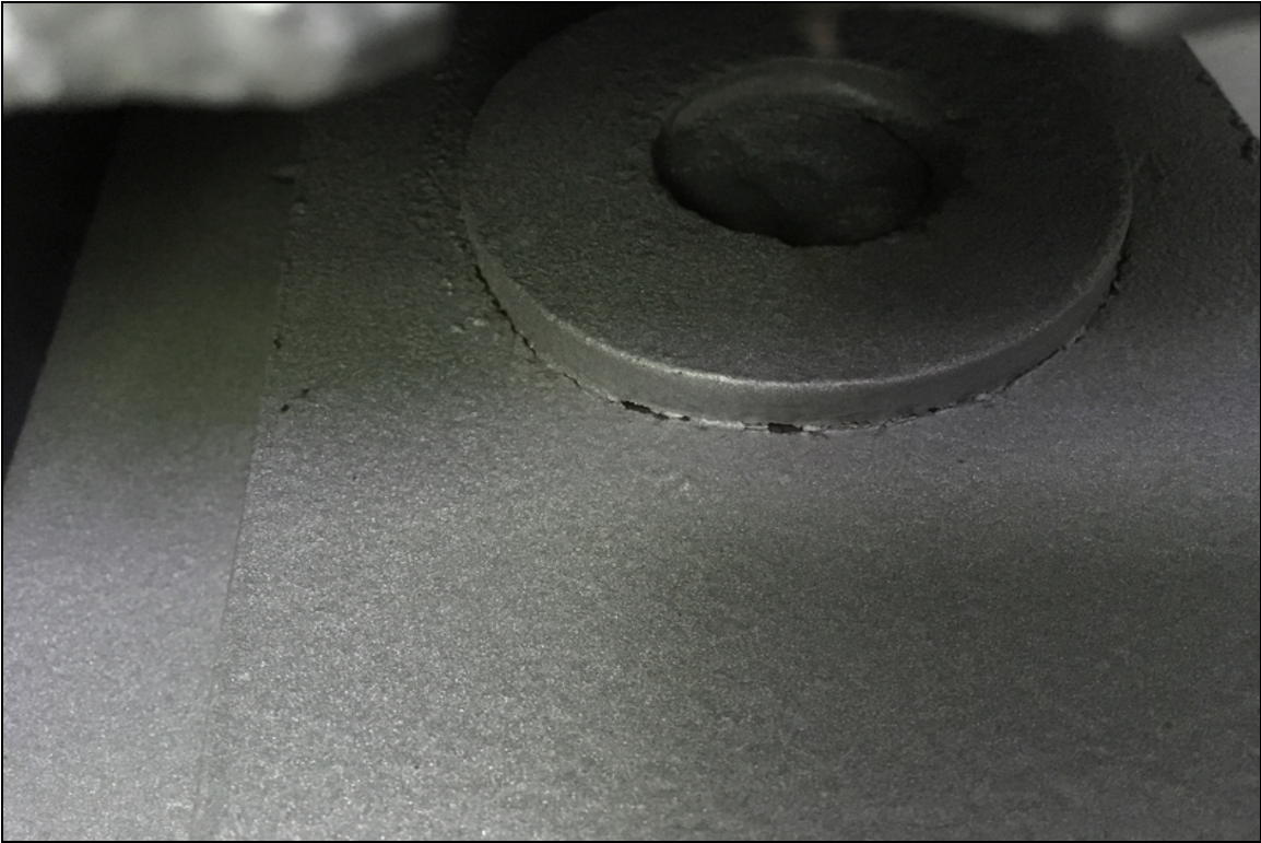
Span 14, Girder 2, Top Pin: Retaining washer weld fractured.
