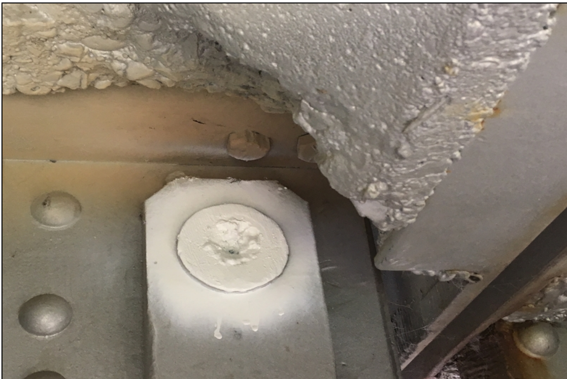
Span 6, Girder 2, Top Pin: Repaired.
