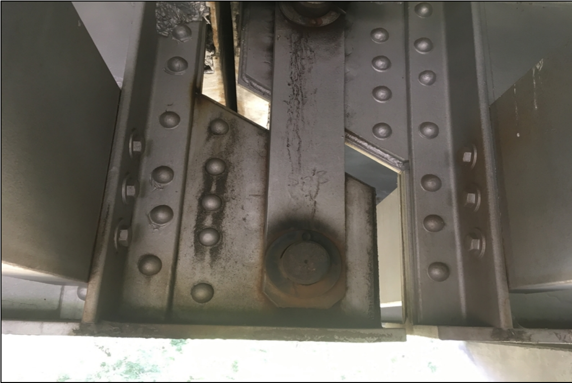
Span 8, Girder 3, Pin & Hanger: Floating.
