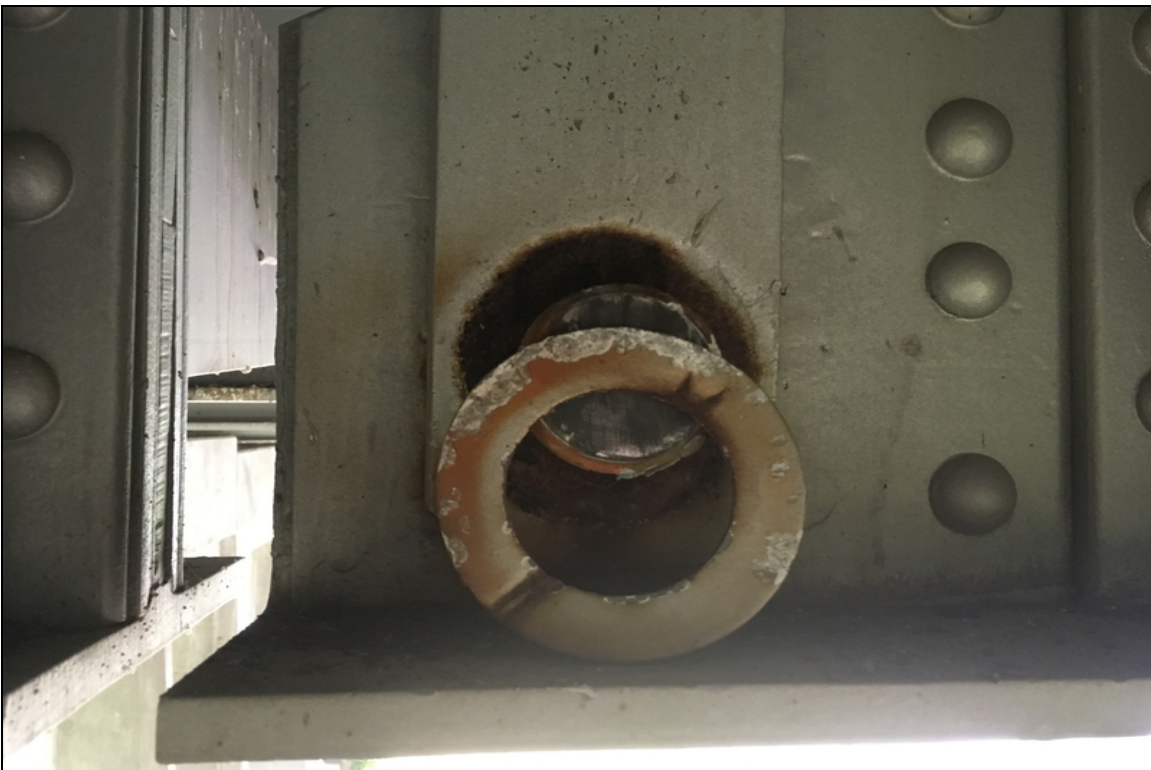
Span 10, Girder 6, Bottom Pin: Keeper missing. Washer loose.
