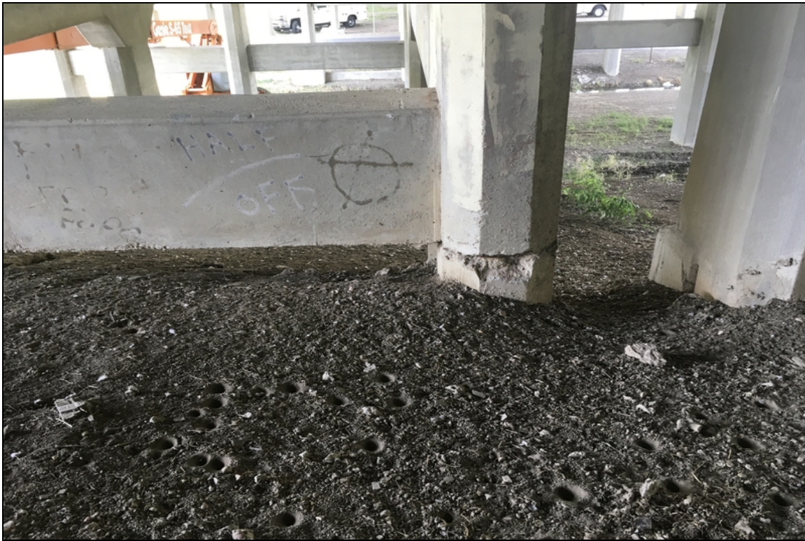
Bent 2, Column 4: Spalling with exposed reinforcing steel.
