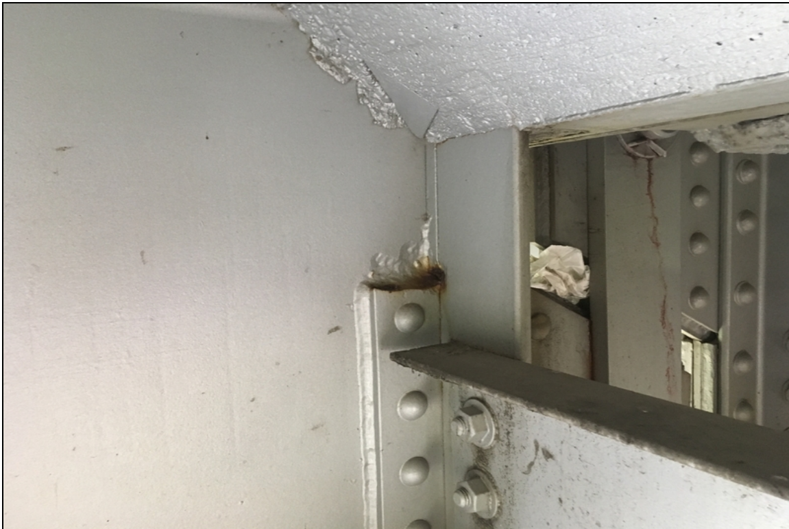
Typical section loss to the diaphragm connections.
