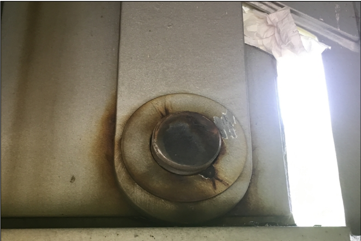
Span 6, Girder 1, Bottom Pin: Keeper missing.
