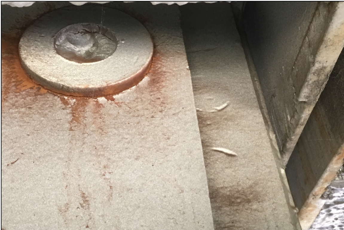
Span 8, Girder 3, Top Pin: Retaining washer weld fractured.
