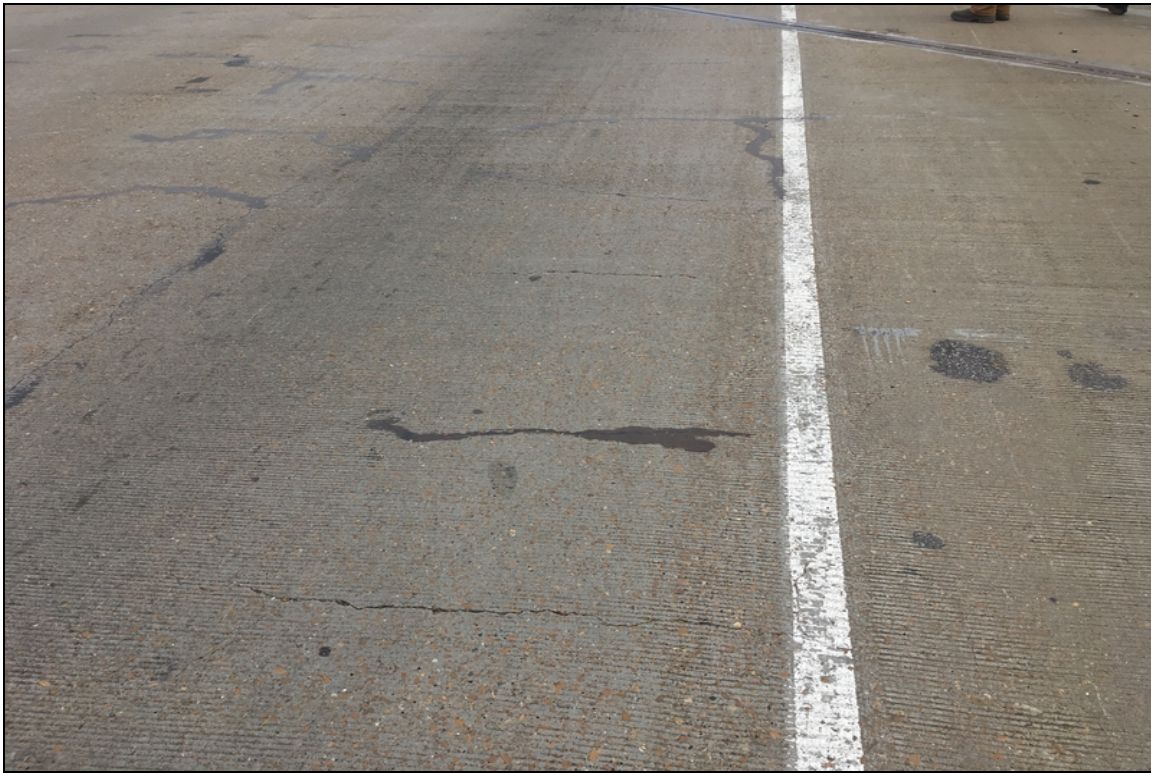
Sealable deck cracking.
