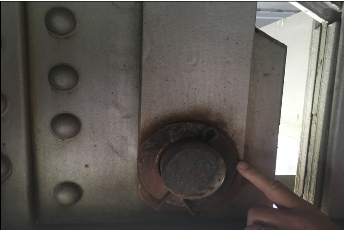
Span 9, Girder 3, Pin & Hanger: Floating.
