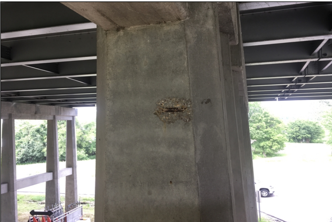
Bent 5, Column 4: Spalling with exposed reinforcing steel.
