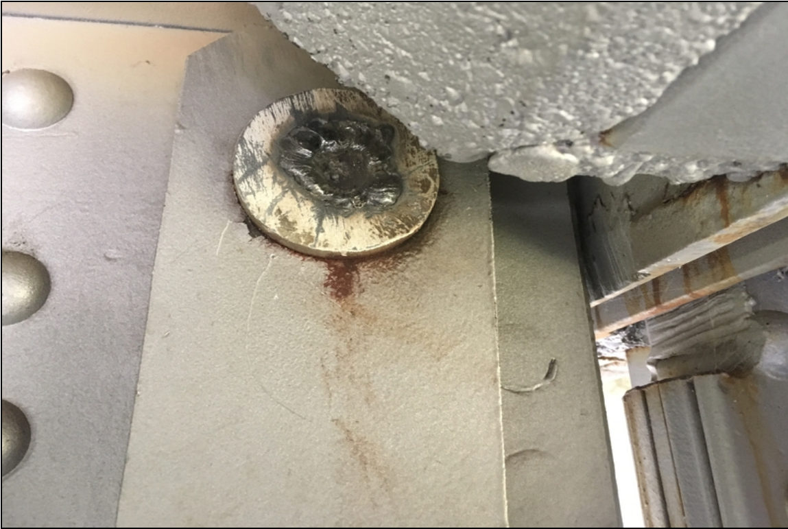
Span 4, Girder 3, Top Pin: Repaired.
