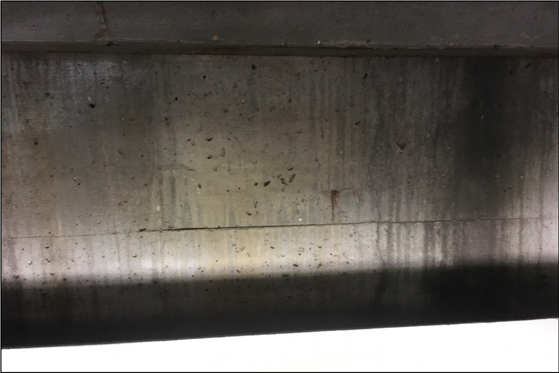
Bent 1, Back Wall: Typical cracking.
