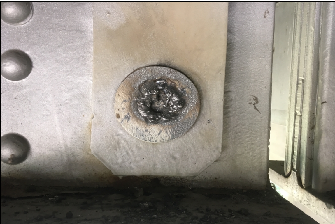
Span 11, Girder 6, Bottom Pin: Repaired.
