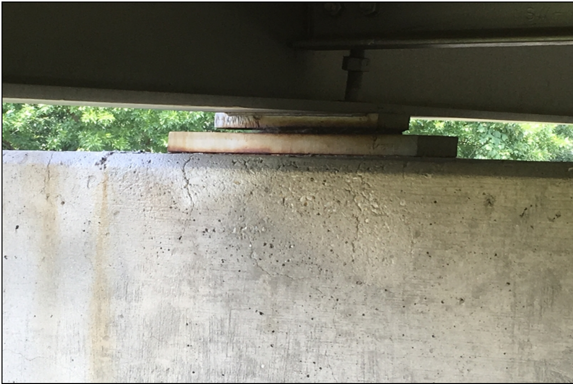
Bent 2, Girder 1, Bearing: Active corrosion and floating
