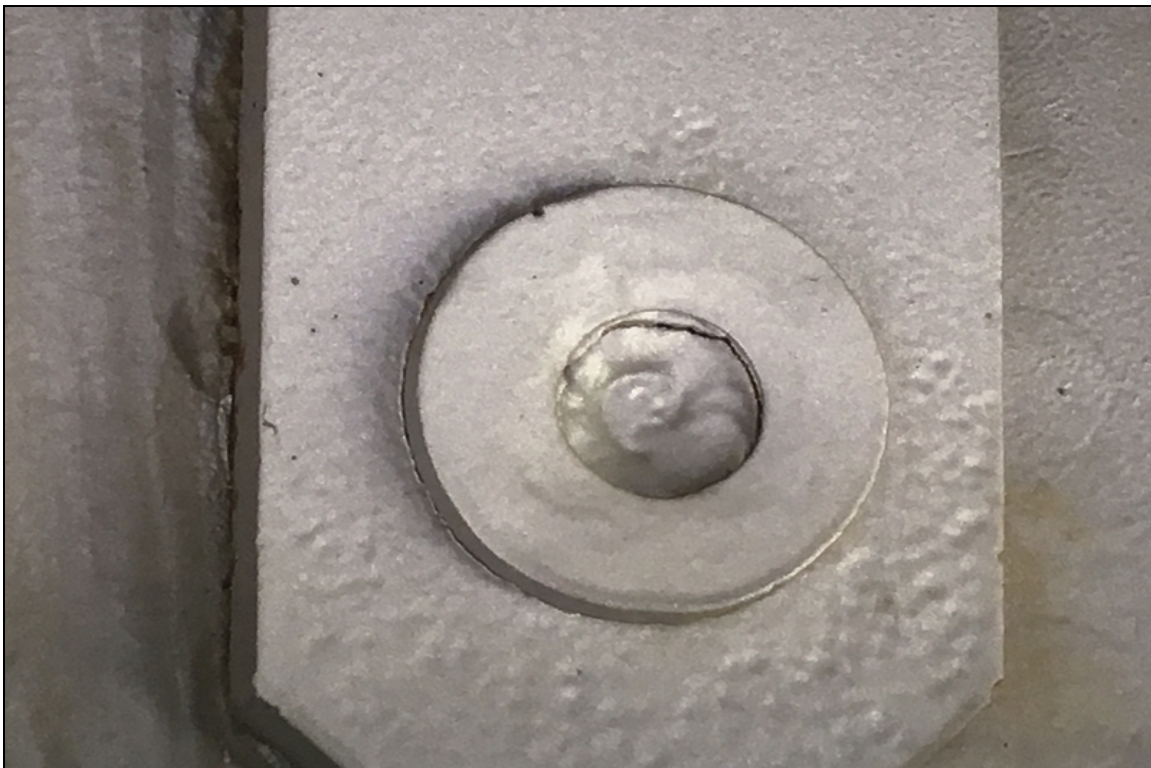
Span 4, Girder 2, Bottom Pin: Retaining washer weld fractured.
