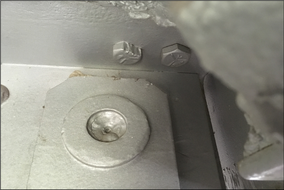
Span 6, Girder 2, Top Pin: Retaining washer weld fractured.
