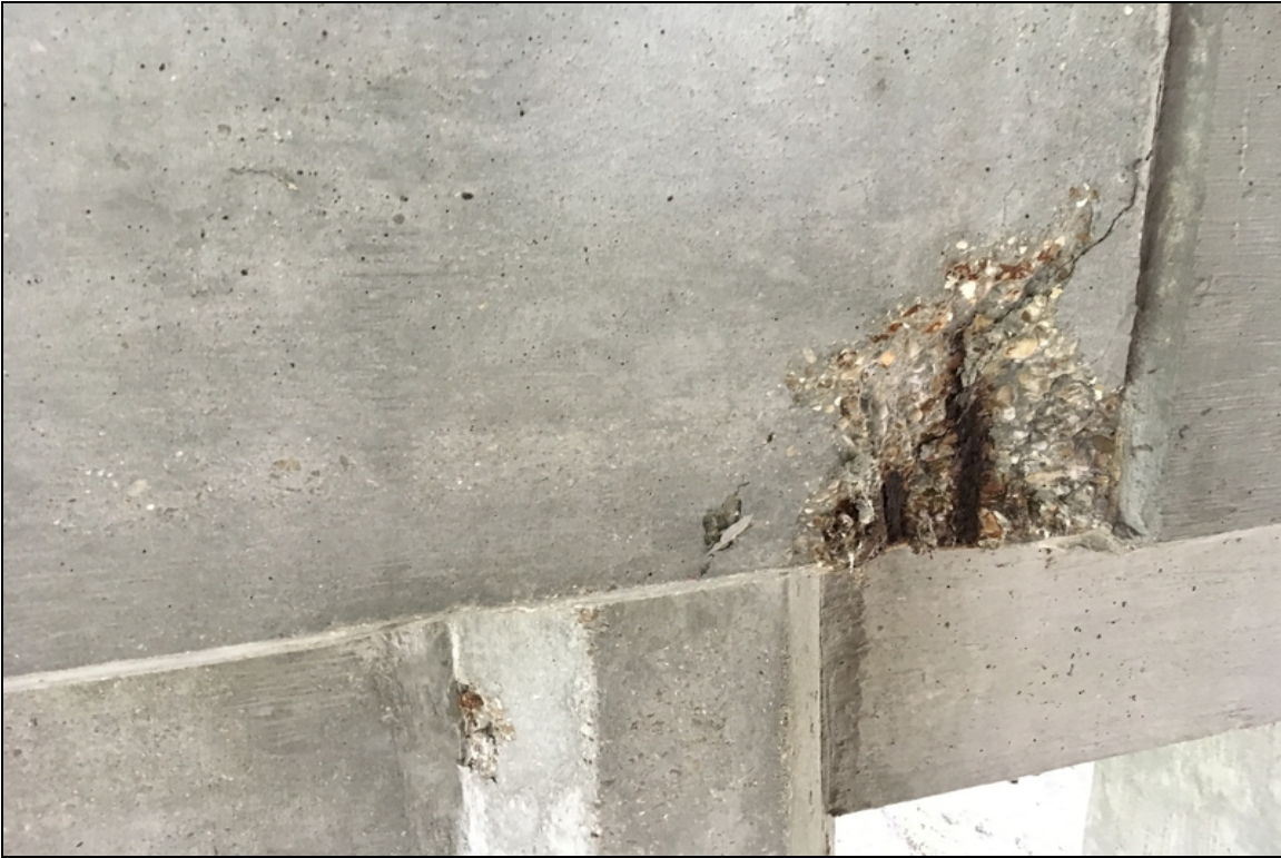
Bent 15, Girder 6, Cap: Spalling.
