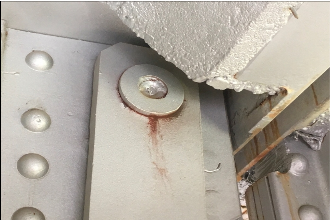
Span 4, Girder 3, Top Pin: Retaining washer weld fractured.
