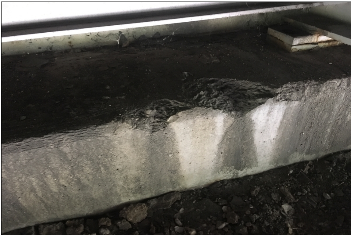
Bent 1: Spalling.
