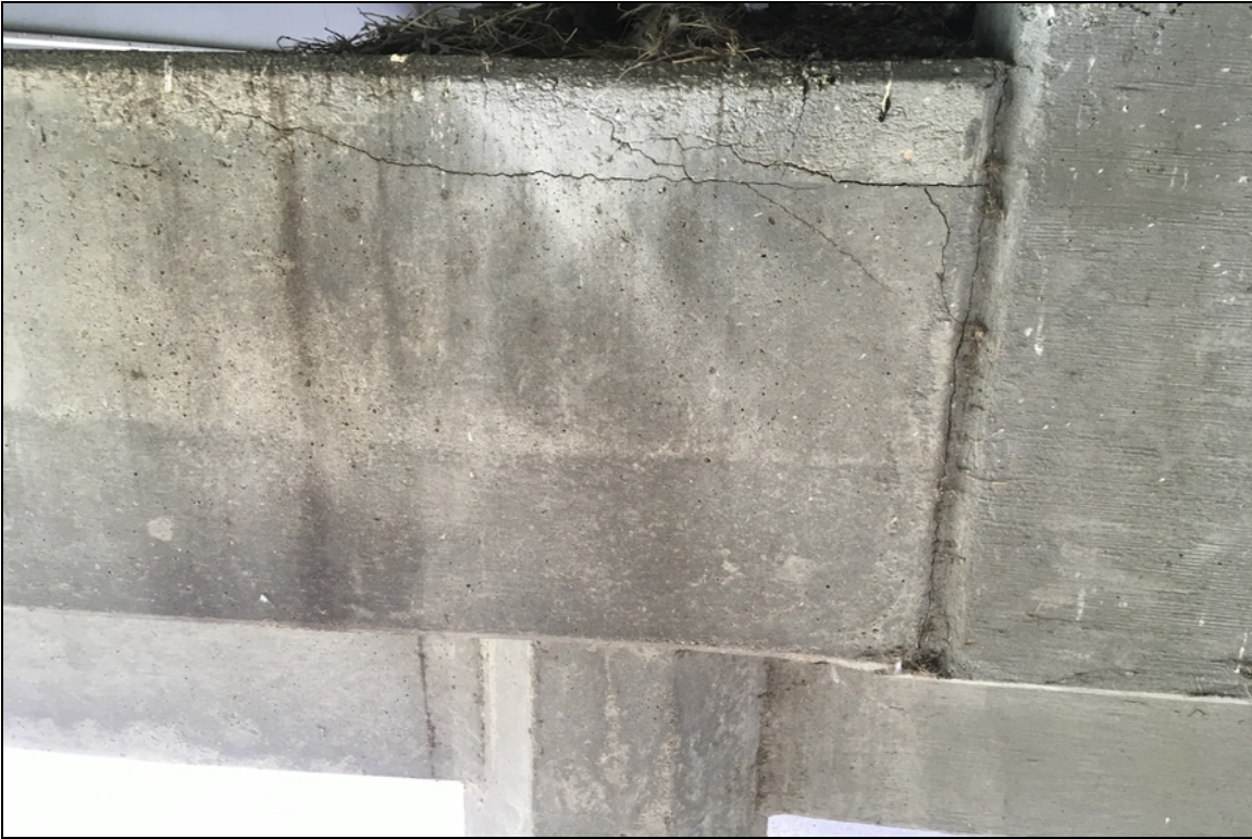
Bent 5, Column 4, Cap: Cracking.
