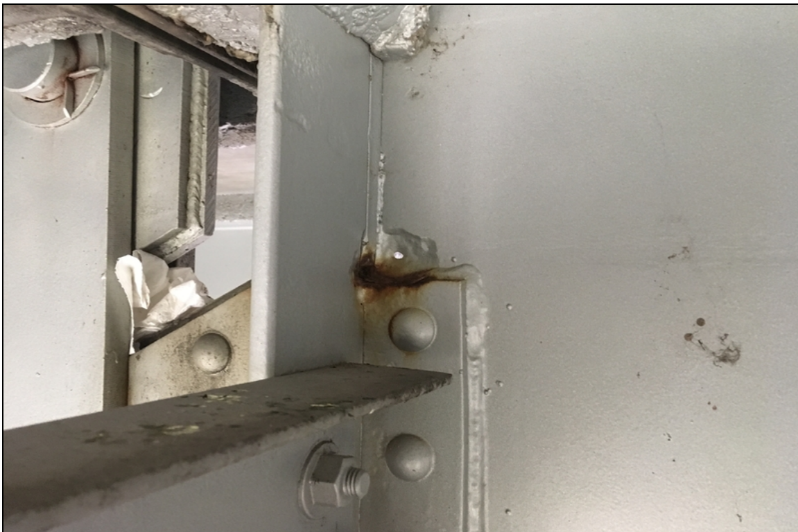
Span 9, Girder 4: Hole through web.
