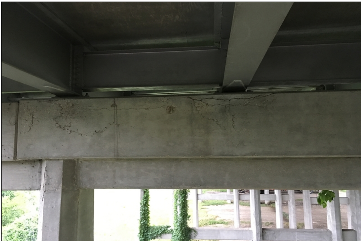
Bent 15, Girder 3, Cap: Cracking.
