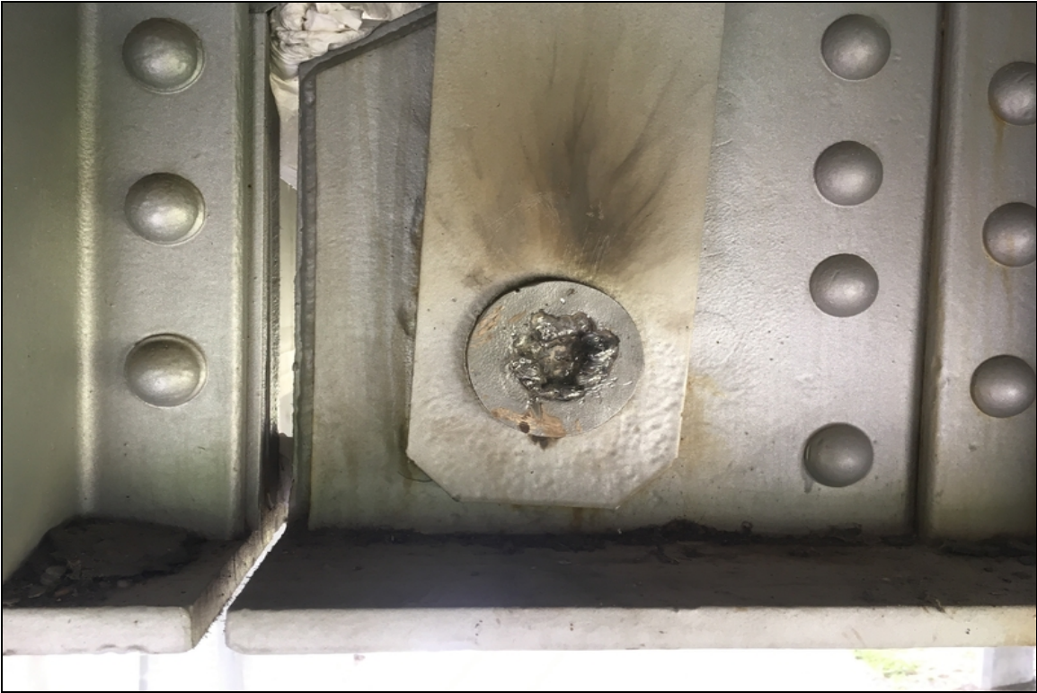
Span 4, Girder 2, Bottom Pin: Repaired.
