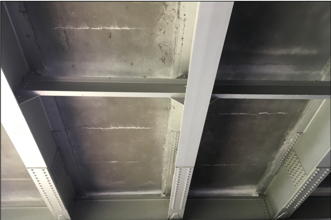
Typical efflorescence in the undersurface.
