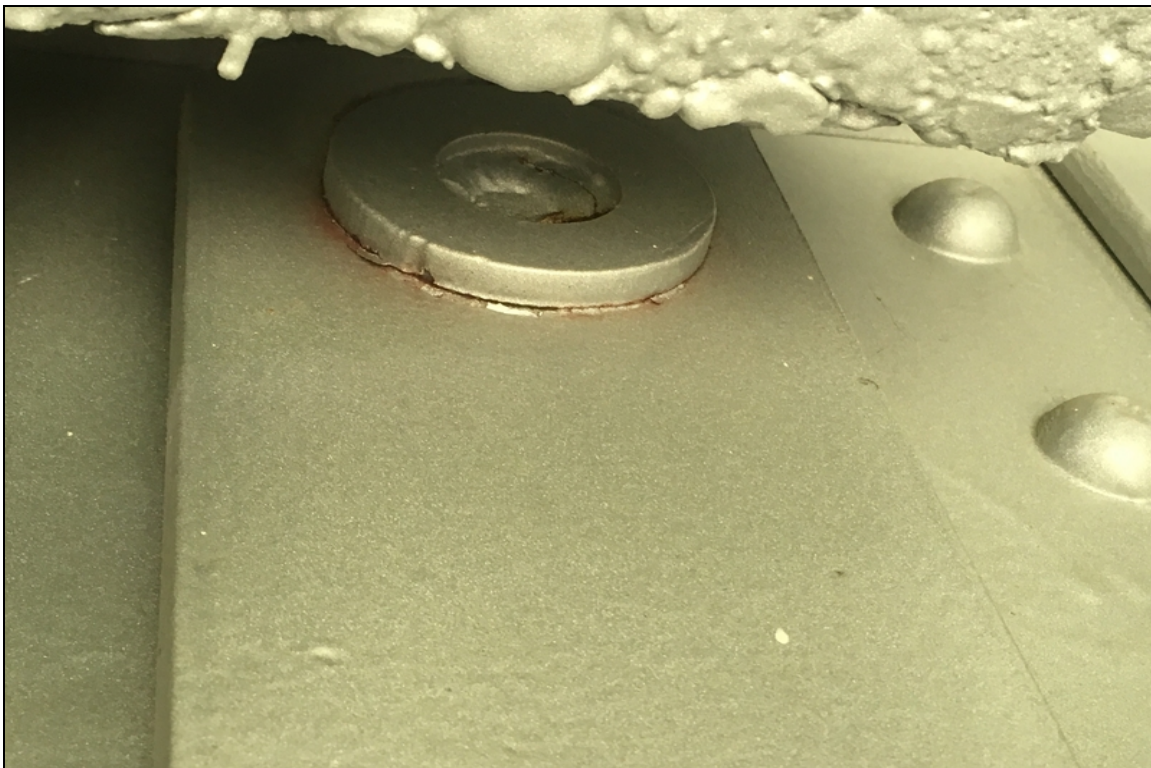
Span 17, Girder 2, Top Pin: Retaining washer weld fractured.
