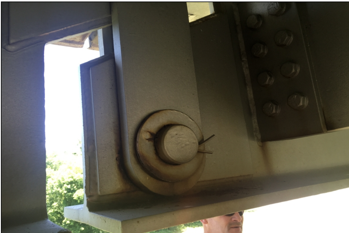
Span 18, Girder 1: Fractured cotter key.
