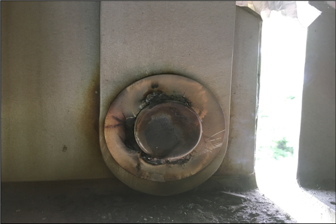
Span 6, Girder 1, Bottom Pin: Repaired.
