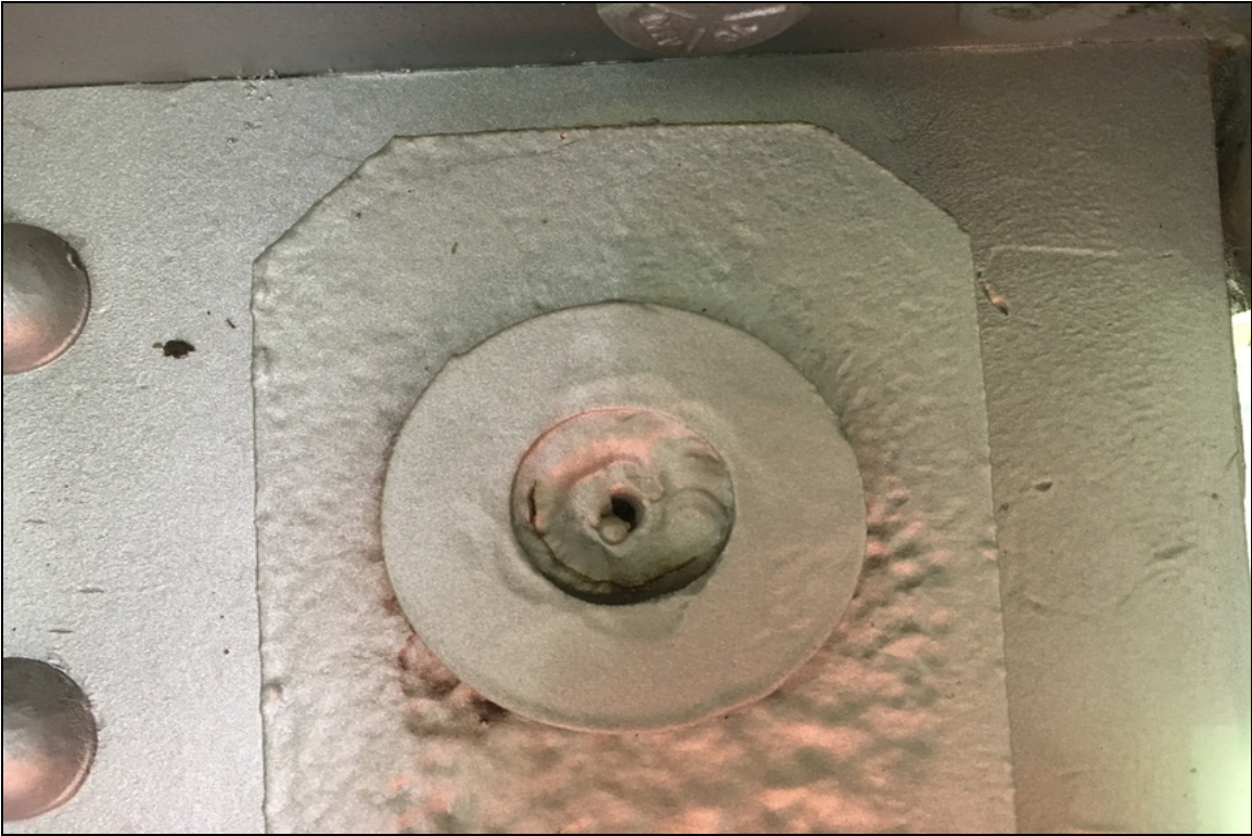
Span 20, Girder 6, Top Pin: Retaining washer weld fractured.
