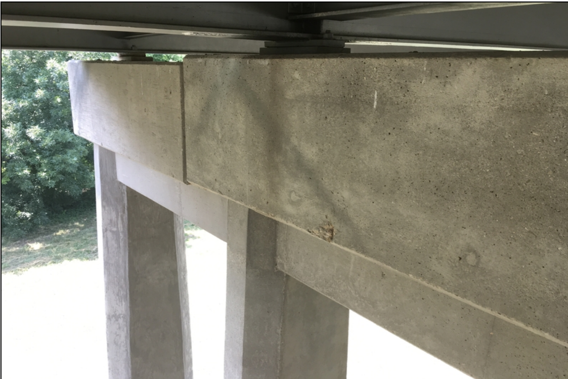
Bent 8, Cap: Minor spalling with exposed reinforcing steel.
