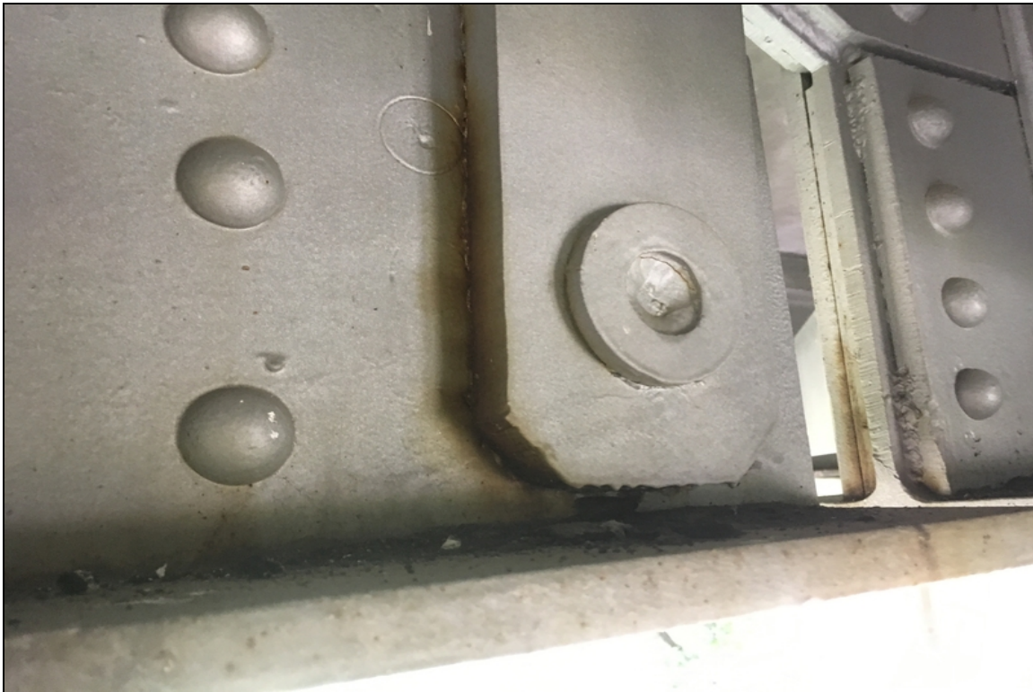
Span 12, Girder 6, Bottom Pin: Retaining washer weld fractured.
