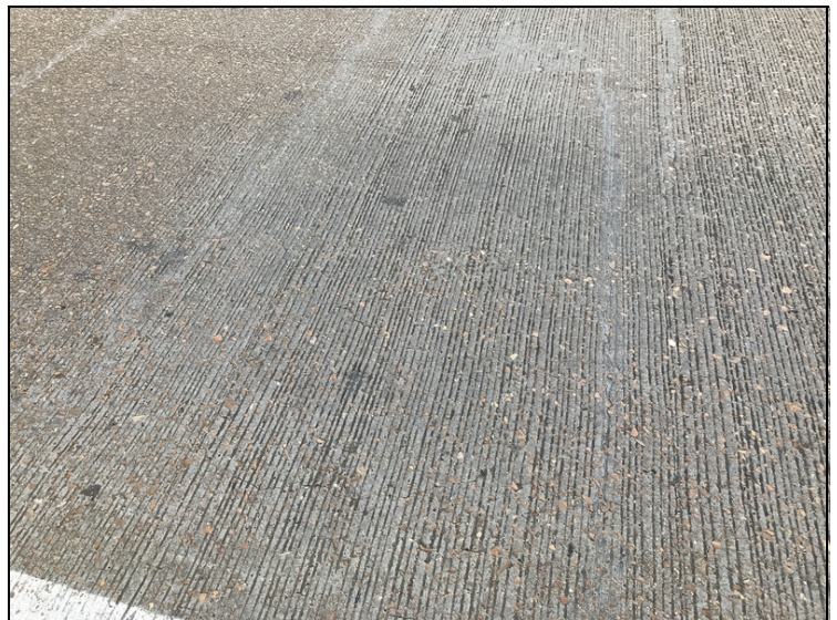
Transverse and longitudinal cracking every 2' - 3' up to 1/32" wide.
