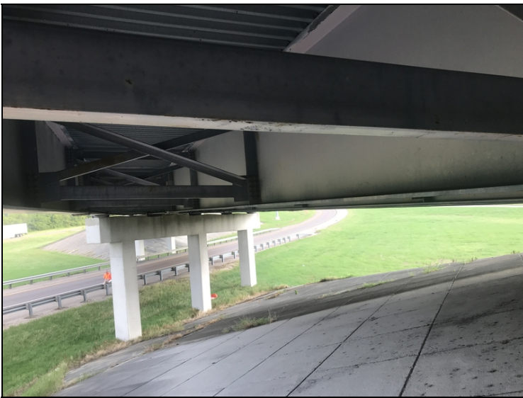
Typical paint condition interior girder
