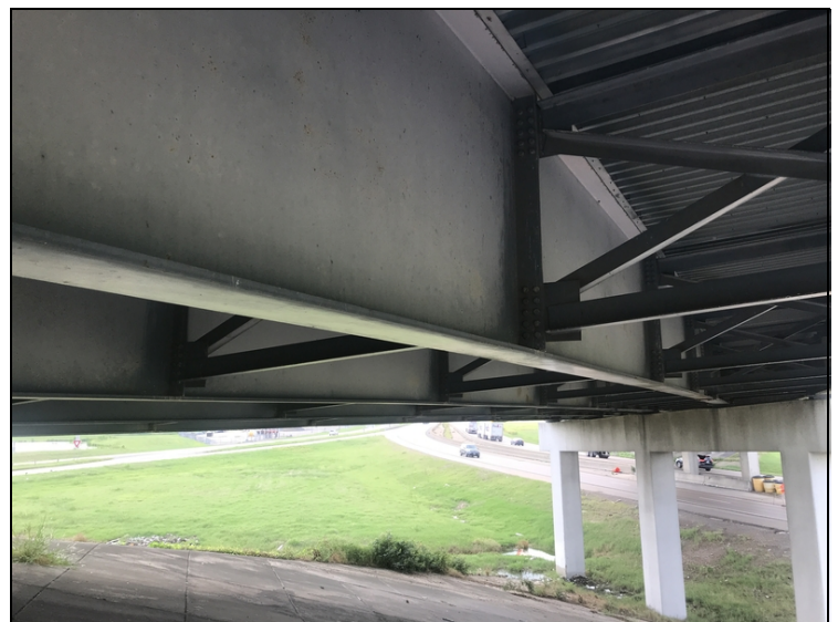
Typical paint condition interior girder
