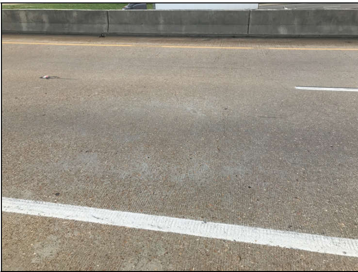
Typical deck cracks
