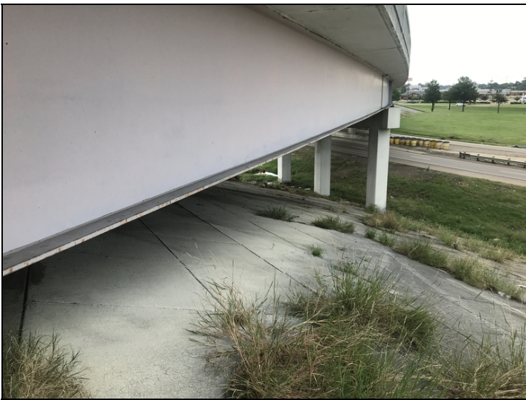
Typical outside girder paint condition.
