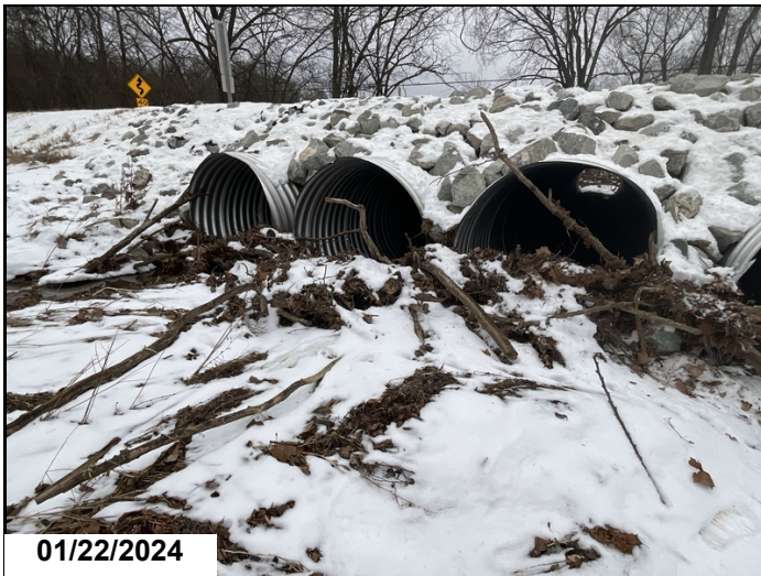
Pipes 1-3 have minor drift buildup
