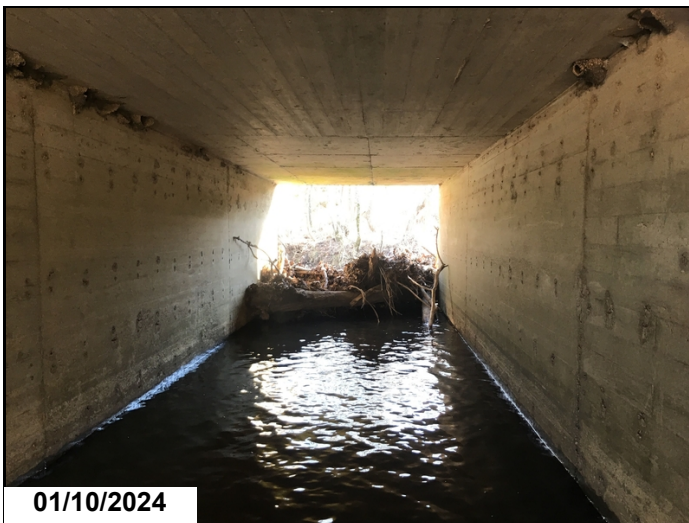
Drift in barrel 2
