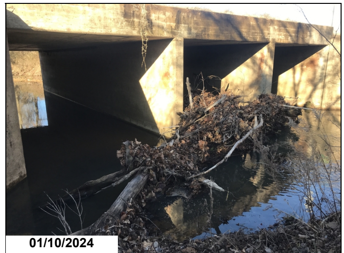
Drift on inlet, right end
