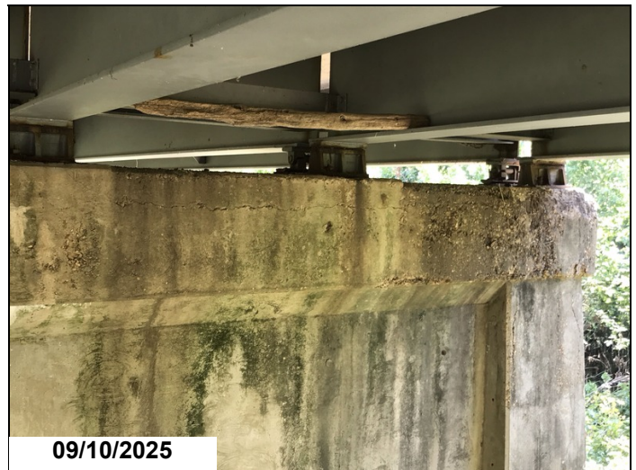
Bent 14 cap ahead face has 8' horizontal cracking CS3.
