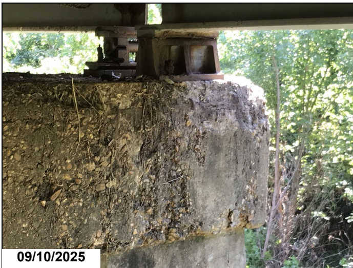
Bent 14 cap ahead right end has 3' spall with exposed rebar CS3
