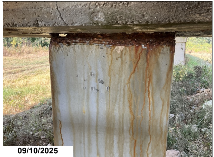
Bent 7 Pile 4 back flange has a 1" x 1/2" hole CS3
