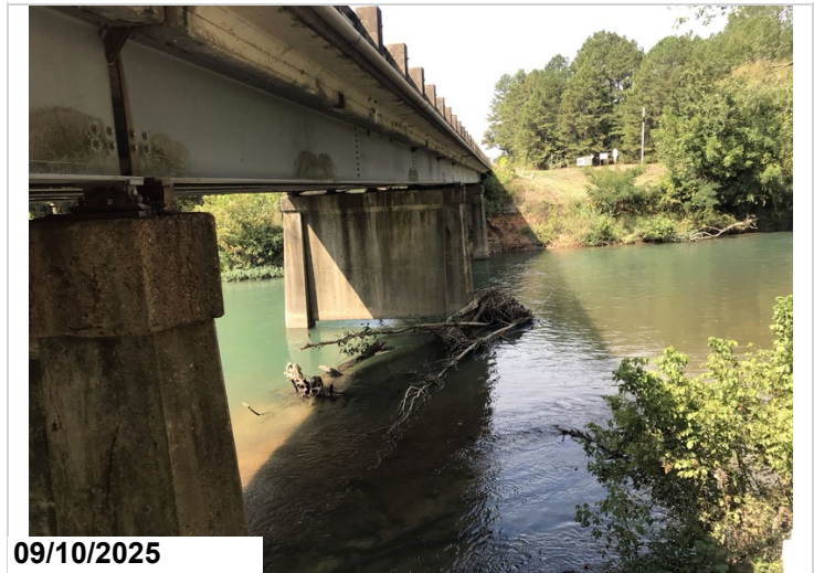
Bent 17 right side drift
