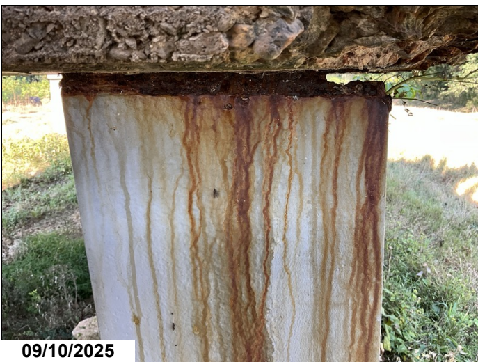
Bent 7 Pile 5 back flange has a 3" x 1/2" hole CS3
