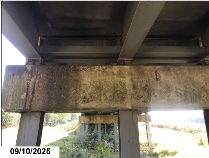
Span 4 bent 4 cap from mid to right end has 6' cracking CS2 and 3' spalls with exposed rebar CS3.
