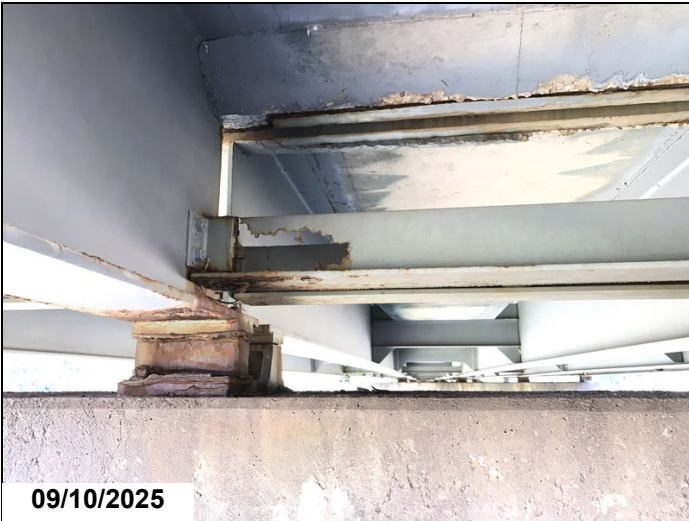
Span 4 bent 5 bay 2 10" x 5" hole in diaphragm
