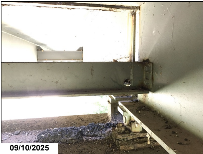
Span 14 bent 15 bay 3 diaphragm has a 2" diameter hole
