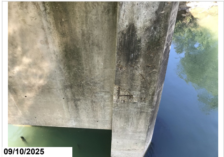
Bent 11 right and left columns have spalls with exposed rebar CS3.
