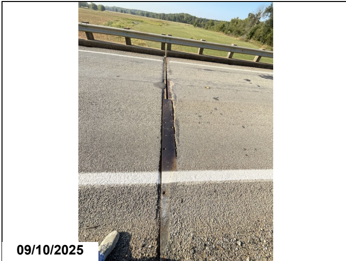
Bent 3 joint slide plate loose
