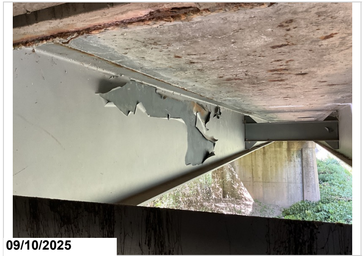
Span 14 Bent 14 Girder 4 Right side paint peeling. CS2 and CS3
