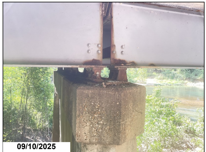
Span 15 bent 15 girder 5 corrosion CS2 and CS3
