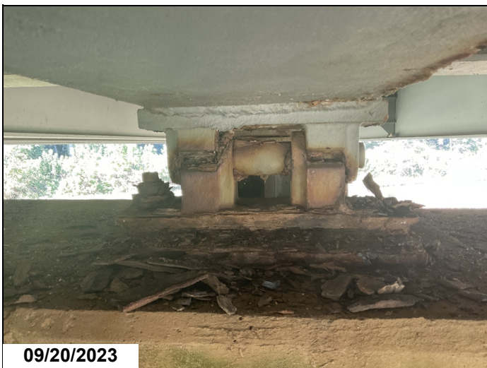
Span 8 bent 9 bearing 4
