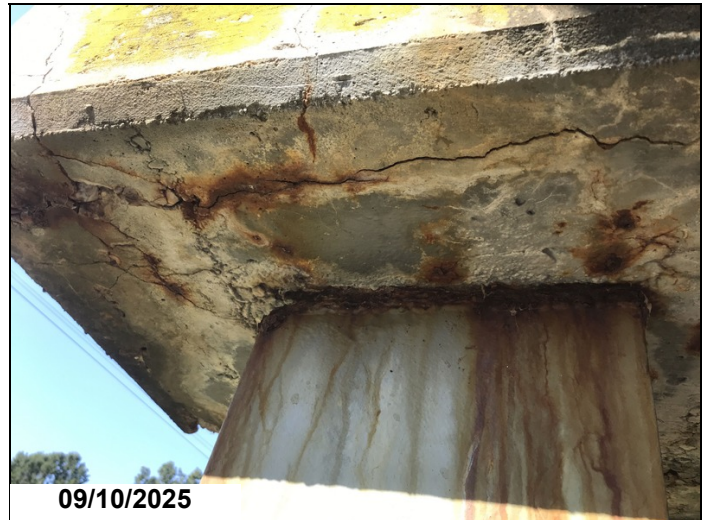
Span 4 bent 5 left end has 1' spall with exposed rebar CS3, and 4' cracking with rust staining CS3.
