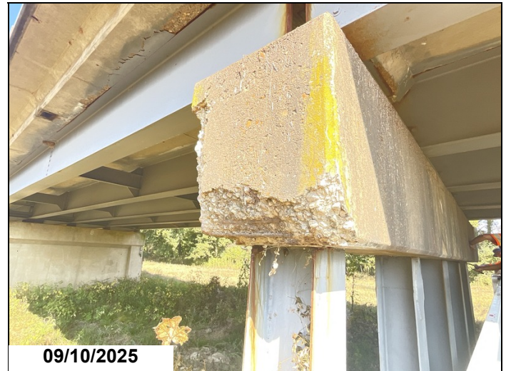
Bent 7 Lt spall/rebar CS3
