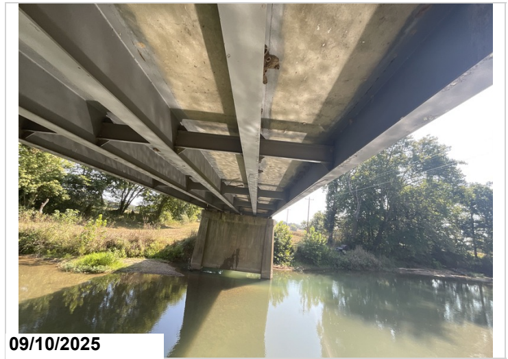
Main undersurface bay 1 efflorescence
