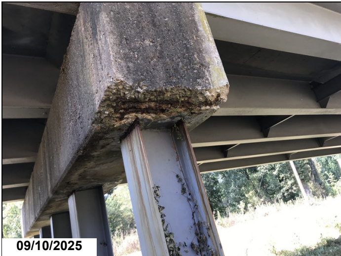
bent 7 cap right end has 1' spall with exposed rebar CS3, over piles 2 and 3 has 4' cracking CS3, 3' spall with exposed rebar CS3.
