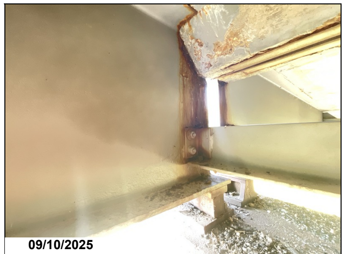
Span 2 bent 3 girder 1 section loss at haunch CS3
