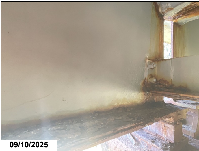
Span 4 bent 5 girder 1 corrosion with areas of section loss
