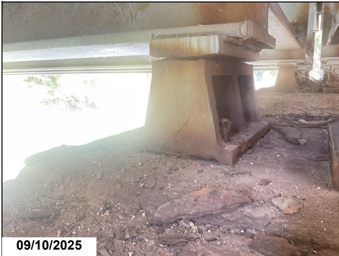
Bent 16 and 17 ahead bearing 2 pushed back with 1/4 gap on ahead side
