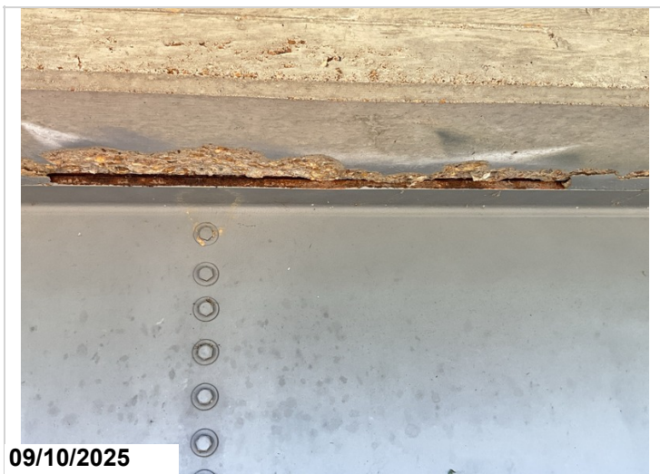
Span 7 Girder 5 Right side top flange is separating from deck
