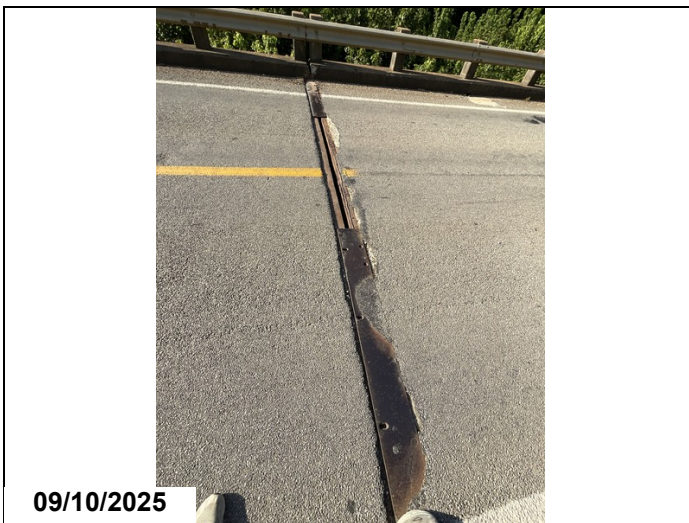
Bent 13 6 missing, 8' loose
