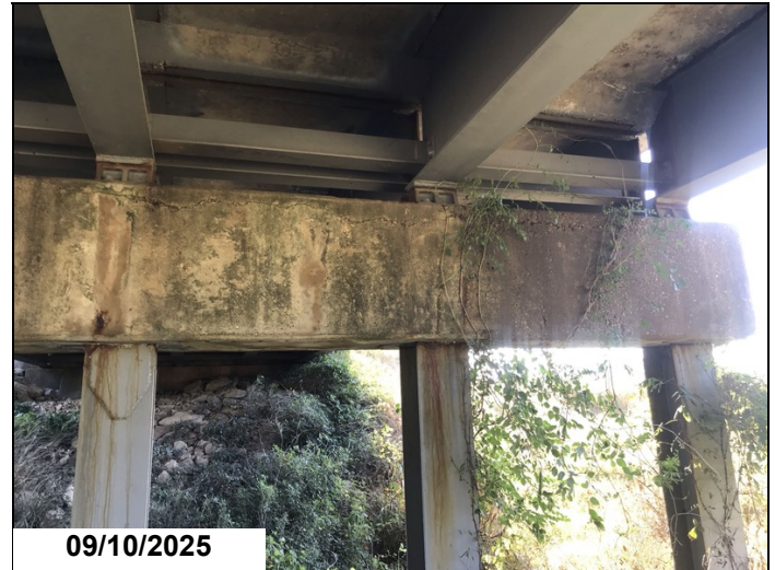
Span 2 bent 2 mid to left end top of cap has an 10' delaminated area CS3.
