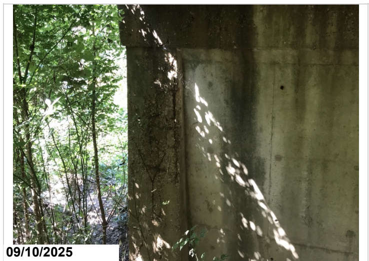
Bent 15 left column has large spall with exposed rebar CS3. Right has spall with exposed rebar CS3.
