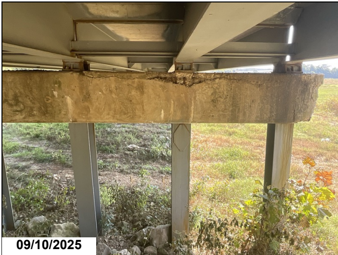
Bent 7 ahead spall/rebar CS3
