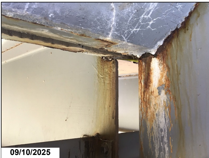
Span 18 bent 18 girder 3 has a 4" x 1" hole below haunch CS3
