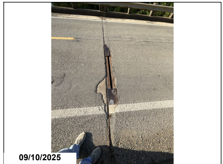
Bent 11 4' missing rest loose
