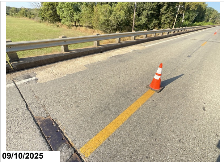
Span 5 Lt gutter typical of several patched areas
