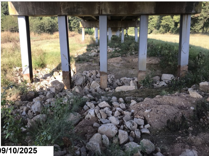
Bent 3 piles past washouts filled with rip rap
