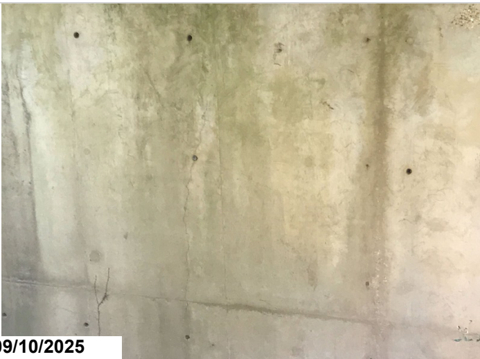
Bent 13 pier wall near mid vertical crack CS3.
