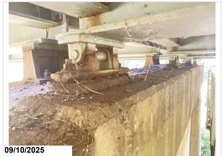
Bent 15 bearings corrosion and pack rust CS3
