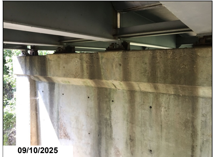
Bent 13 cap has full length horizontal cracking CS3 1' is spall with exposed rebar CS3.
