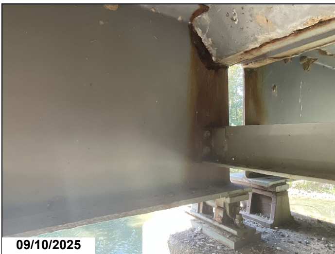
Span 9 bent 10 girder 1 moderate loss CS3
