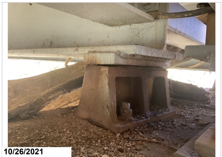
Span 12 bent 12 bearing 4 pack rust CS3
