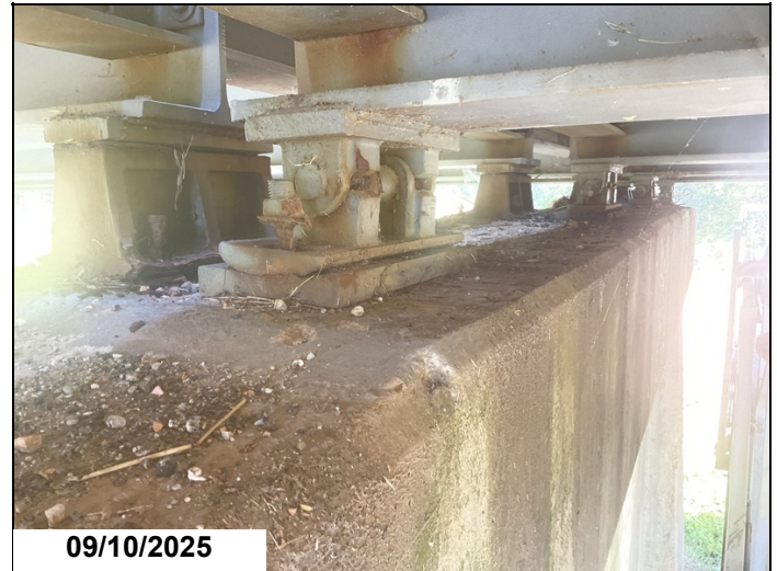
Main span typical bearings
