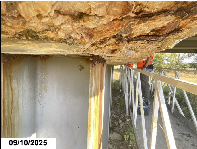
Bent 4 pile 1 Lt back flange 1/8" deep section loss CS3
