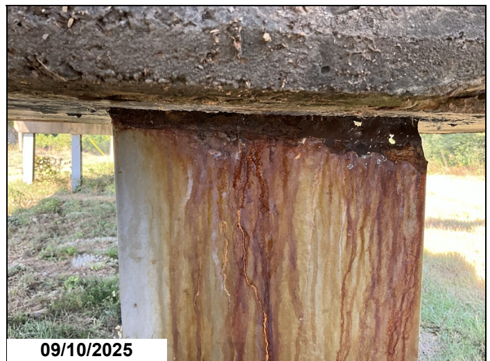
Bent 6 Pile 5 back flange has a 2" x 1/2" hole CS3
