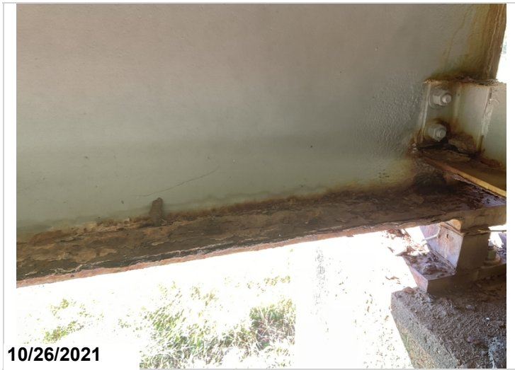
Span 4 bent 5 girder 1 active corrosion CS2
