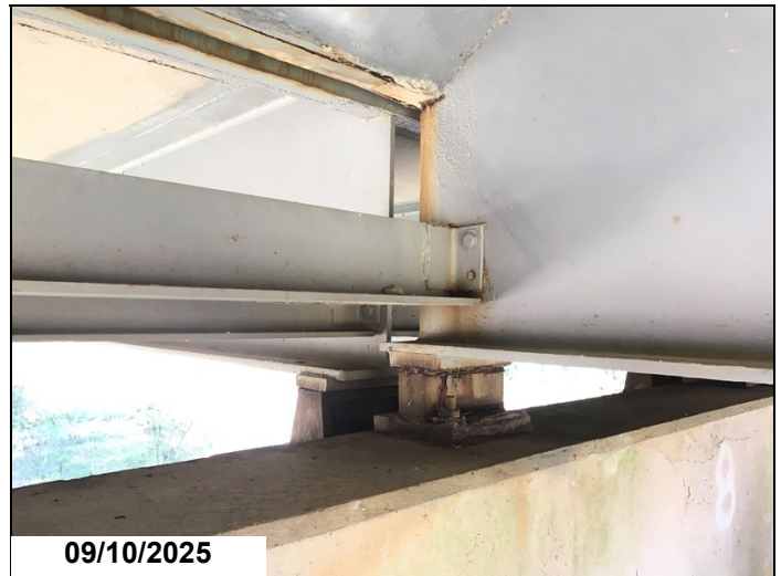
Span 7 bent 8 bay 2 girder 3 diaphragm bolt head is sheared off
