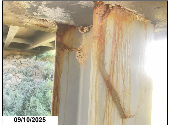
Bent 2 pile 3 back Rt flange knife edged at connection to cap CS3
