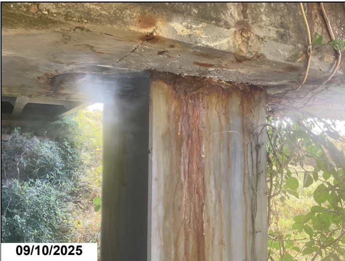
Bent 2 pile 2 ahead corrosion CS3
