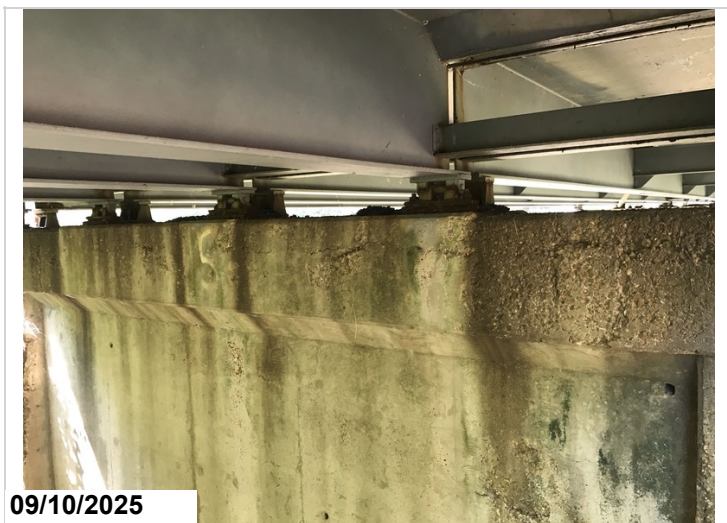
Bent 15 cap back right end has 12' horizontal cracking CS3, ahead has 6' horizontal cracking CS3.
