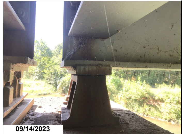
Span 17 bent 17 bearings shifted
