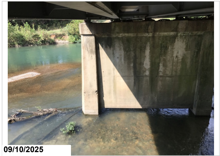
Bent 16 columns have spalls with exposed rebar CS3.
