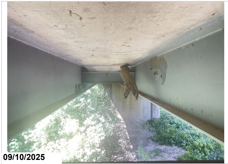
Span 14 paint 60' CS2
