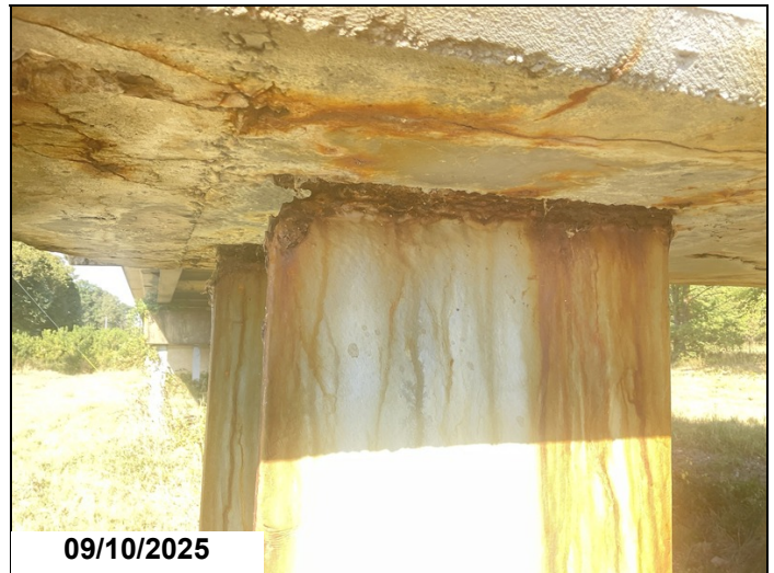
Bent 5 pile 1 has 1" hole on edge of back Lt flange CS3
