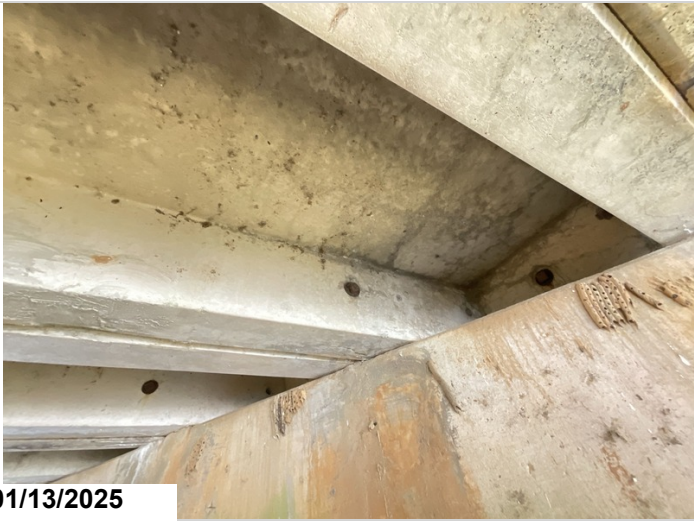
Span 1 bent 2 unit 5 Lt leg 2' patch CS2
