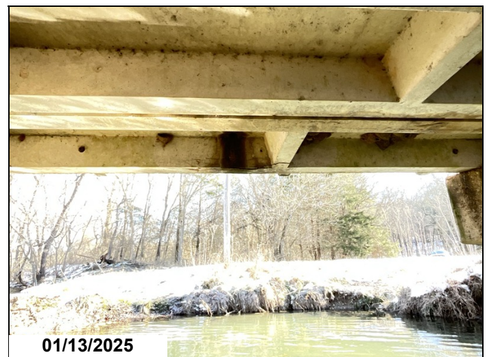
Span 2 unit 7 cracks CS3
