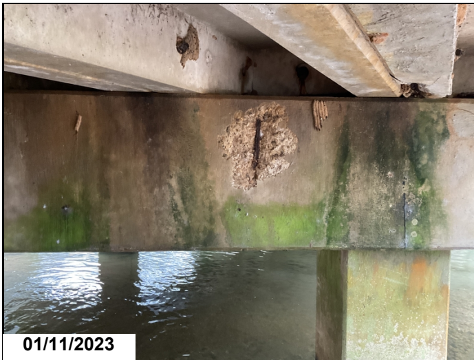
Bent 4 ahead rebar CS3
