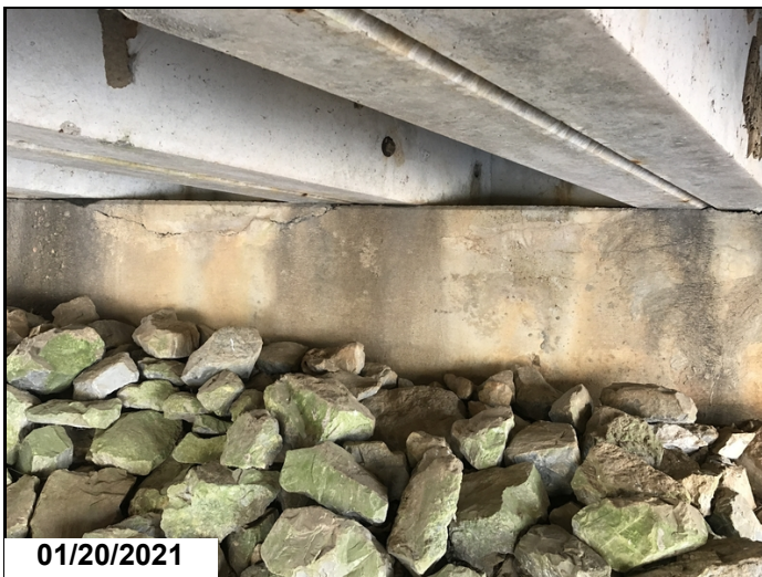
Bent 1 cracks/delam CS3
