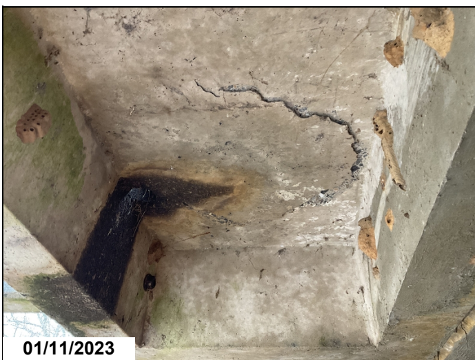
Span 4 unit 1 undersurface delam
