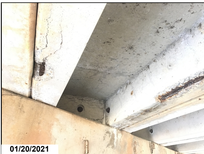
Span 1 unit 3 rebar CS3
