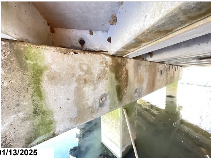
Bent 2 cap typical cracks/delaminated areas
