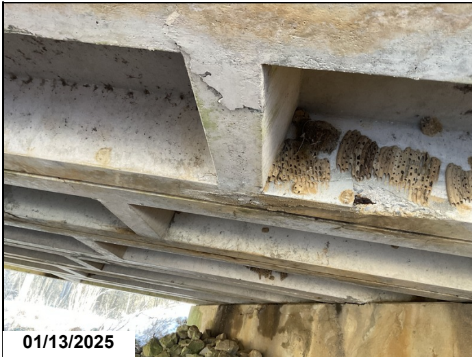
Span 1 unit 2 rebar CS3
