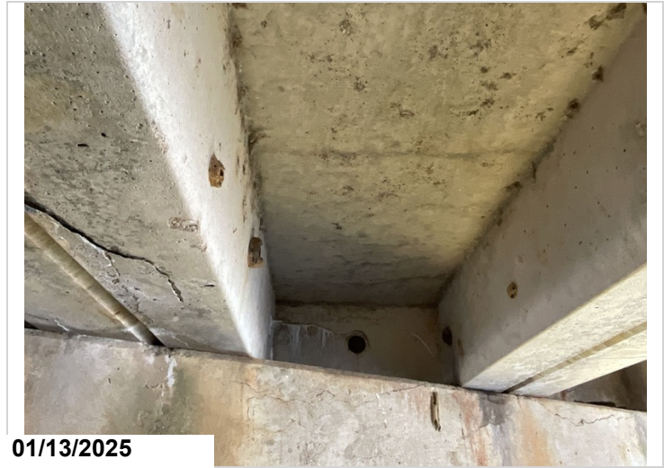
Span 1 bent 2 unit 6 cracks CS2 and 3
