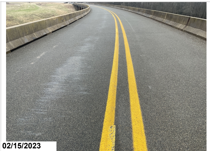
Deck HBM Polymer observed 2-15-2023
