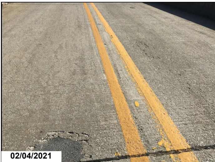
cracks, spalls, abrasion
