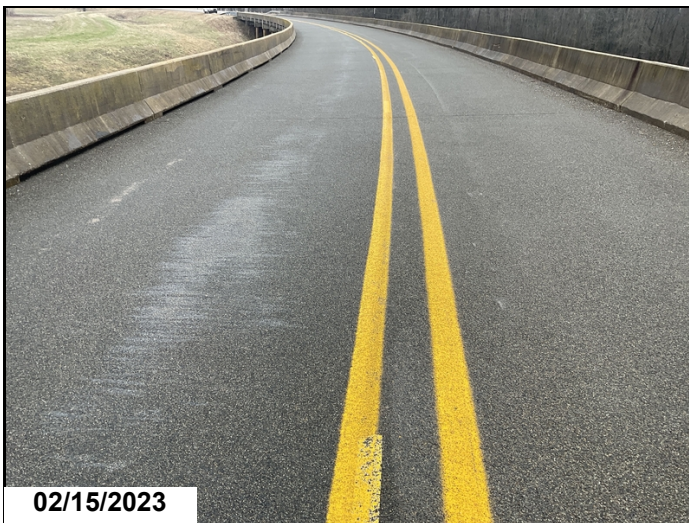
Deck HBM Polymer observed 2-15-2023
