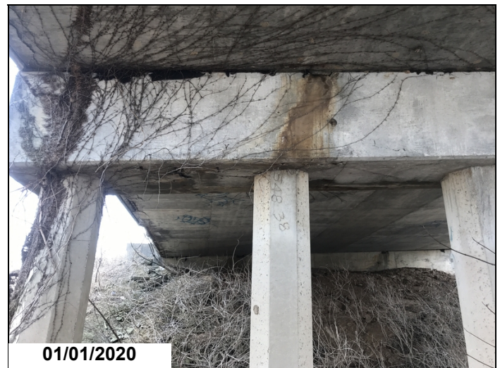
Bent 14 delam
