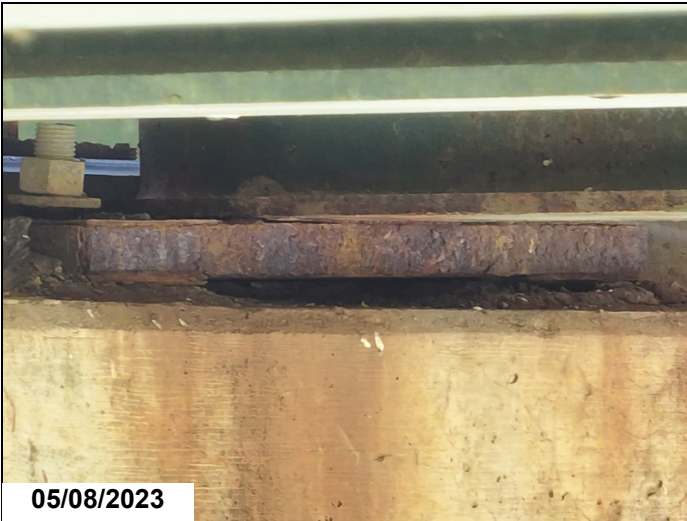
Span 4 bent 4 girder 2 elastomeric bearing pad missing
