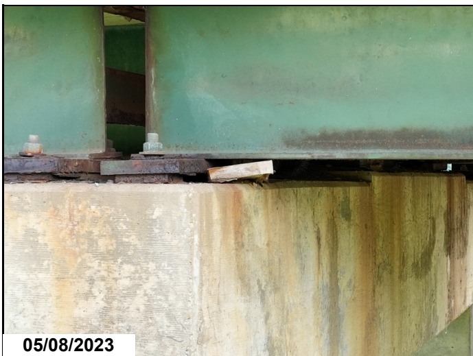
Span 4 bent 4 girder 4 elastomeric bearing pad < 20% remaining in place.
