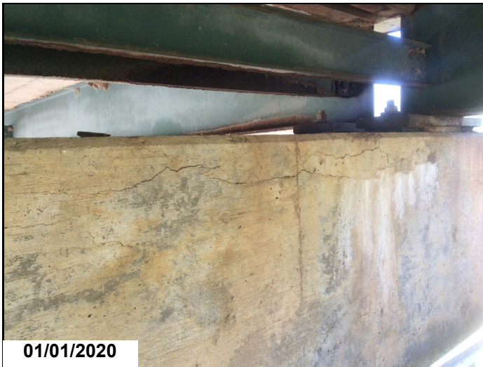
Typical cap cracking and bearings
