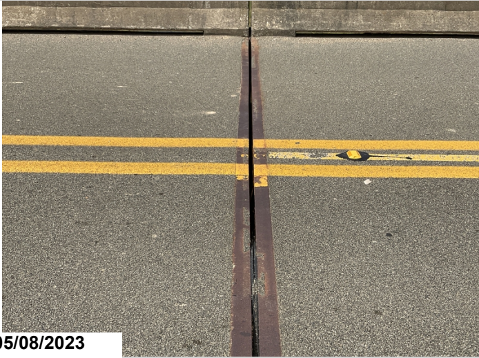
Bent 6 joint seal
