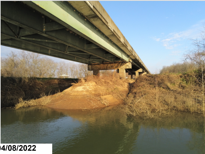
RUNOFF EROSION ON THE WEST BANK UNDER THE BRIDGE
