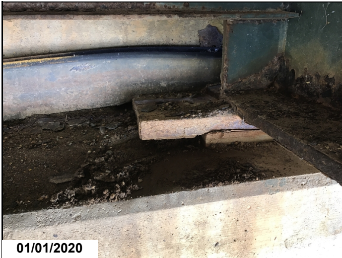
Span 7 Bent 7 Girder 2 missing anchor bolt
