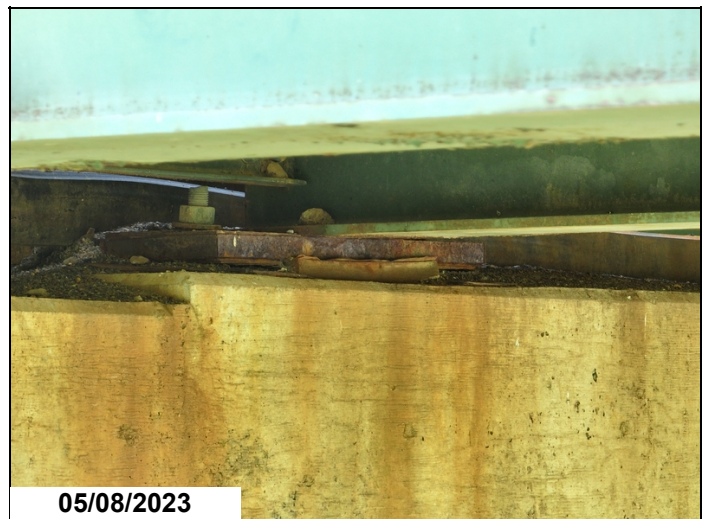
Span 4 bent 4 girder 3 elastomeric bearing pad moving
