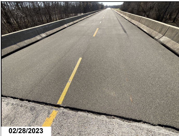
Polymer deck observed repair by statewide crews 2-28-2023
