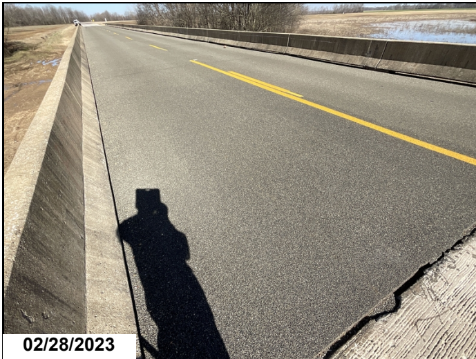
Polymer deck observed repair by statewide crews 2-28-2023
