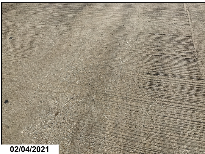
Map cracks in wheel path
