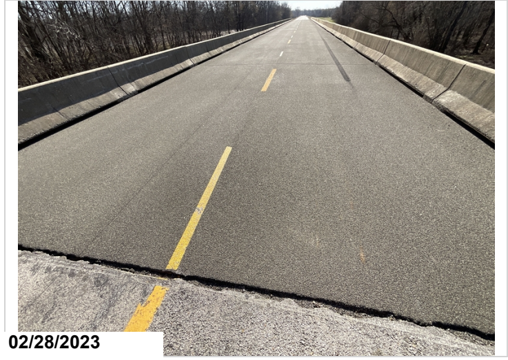
Polymer deck observed repair by statewide crews 2-28-2023
