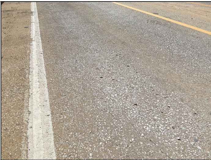
cracks/abrasion with pop outs
