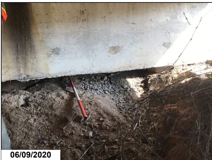
Bent 1 erosion LT SIDE 2019
