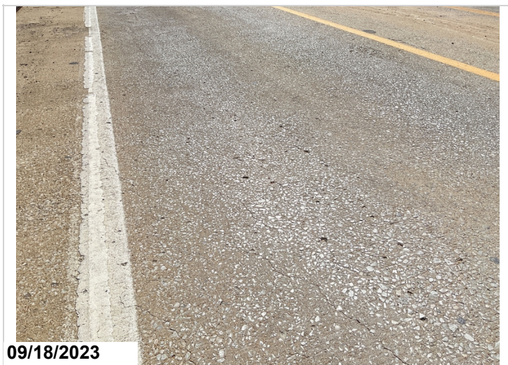
cracks/abrasion with pop outs
