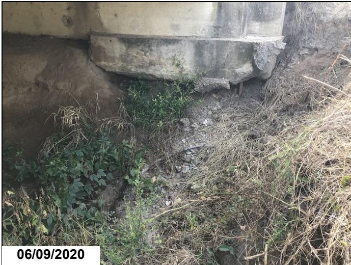
Bent 4 erosion RT SIDE 2019
