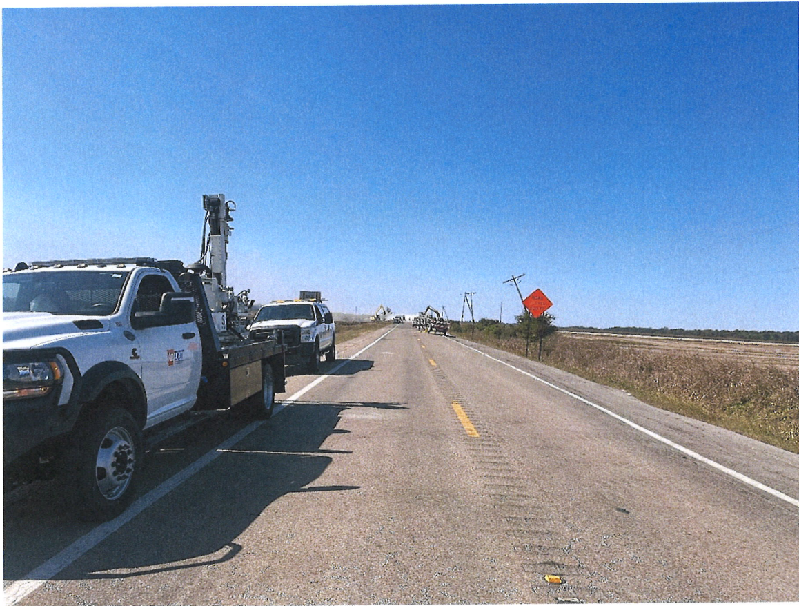
Highway 140 west end of project looking west.
