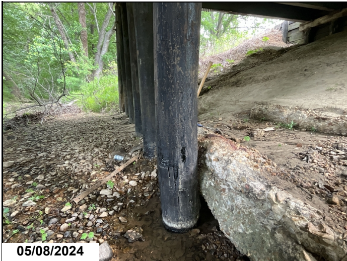
Bent 2, Pile 3: concrete slid against pile. Pile has some outer split and delam on ahead side
