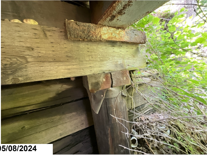
Bent 1, Pile 1: spacer block split
