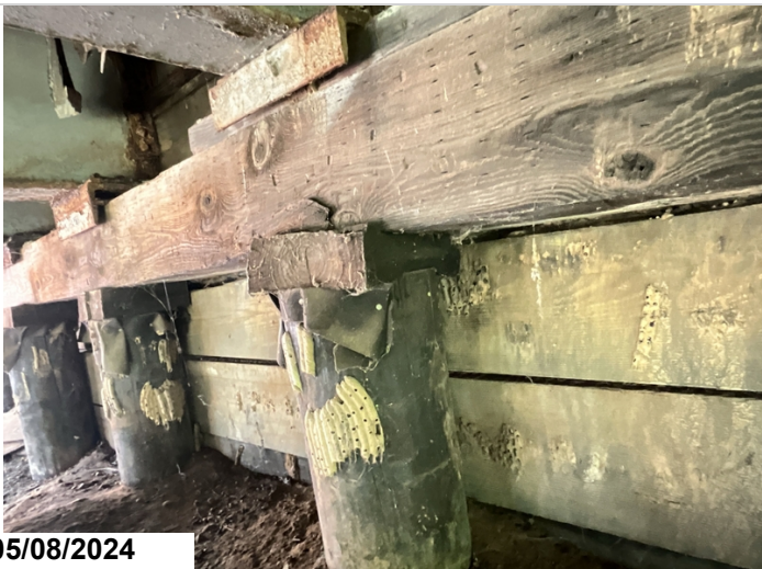
Bent 1, Pile 5: spacer block is decay and crushing
