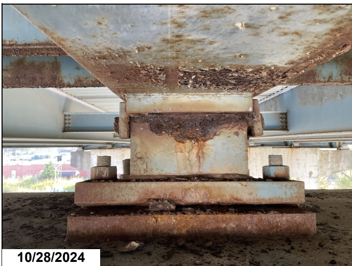
Span 3 bent 4 bearing 4 retainer is bowed from pack rust at cap screw. CS3
