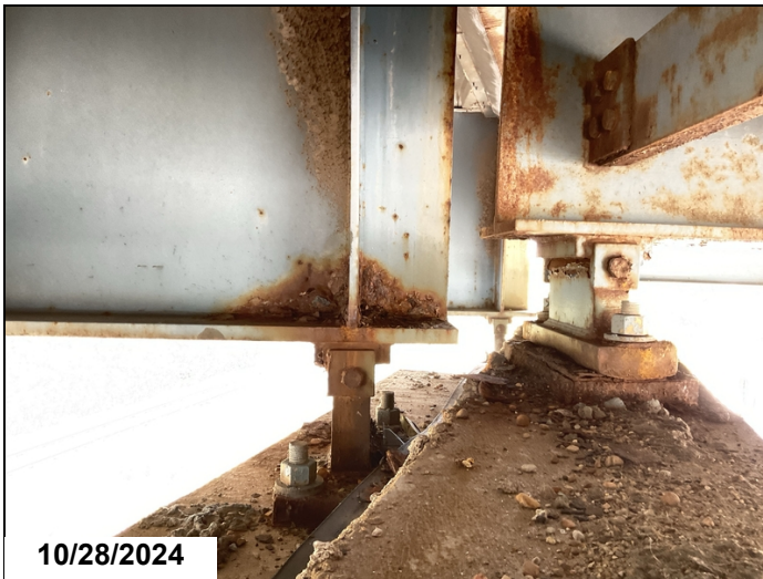
span 5 bent 5 girder 7 CS3
