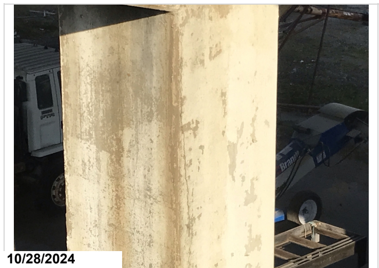
Bent 4 column 3 ahead has a vertical crack CS3
