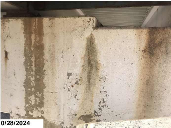
Bent 9 cap has 1' of cracking with rust stains CS3 and 1' of cracking CS2
