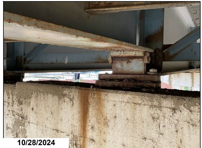
Span 4 bent 5 bearing 3 has 1 anchor bolt sheared off
