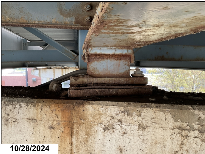
Span 4 bent 5 bearing 4 has 1 anchor bolt sheared off
