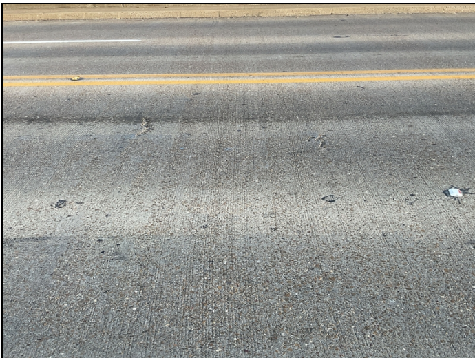
Span 2 East bound delam/shallow spalls
