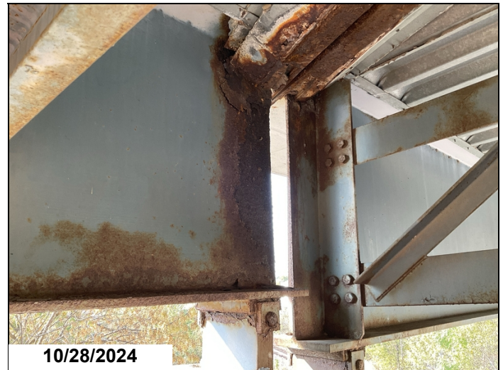
Span 6 bent 6 girder 8 CS3
