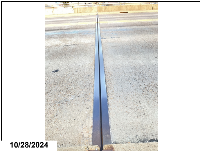
Bent 2, 5 seal missing
