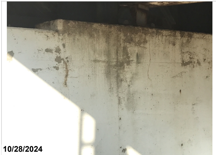
Bent 6 cap has 4' of vertical cracks CS2
