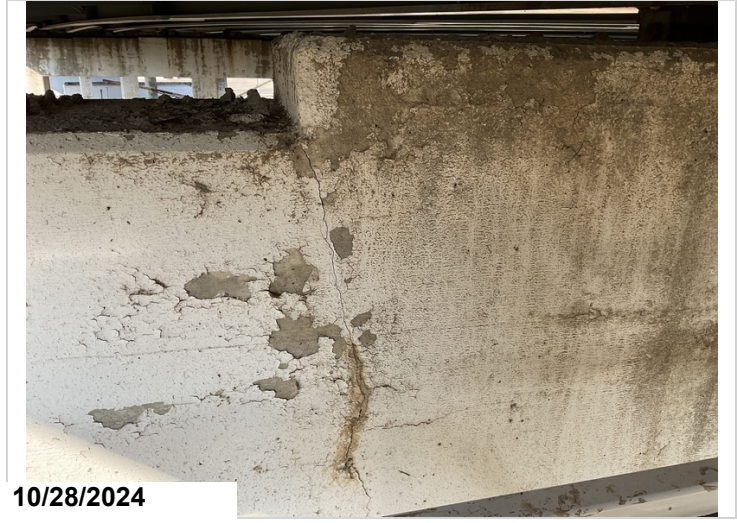
Bent 6 ahead Rt crack CS3
