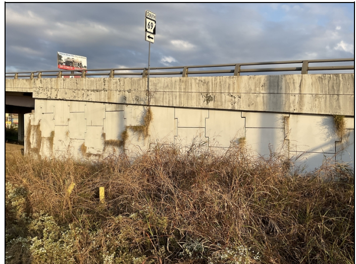
Bent 10 Rt vegetation in mse joints
