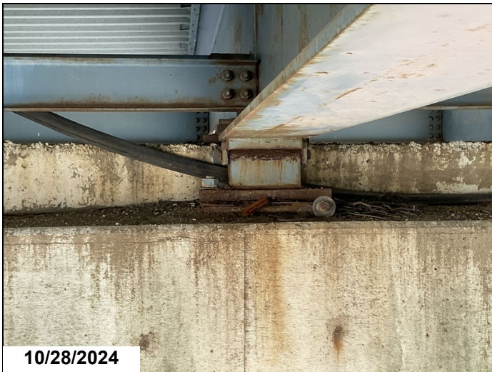
Span 6 bent 7 bearing 4 has 1 anchor bolt sheared off
