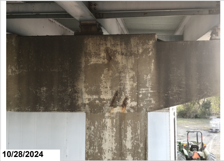
Bent 2 cap has 1' spall with exposed rebar CS2 and 1' cracking CS2
