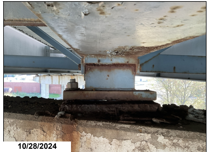
Span 4 bent 5 bearing 6 has 1 anchor bolt sheared off
