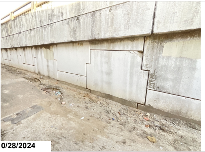
Bent 1 Rt starting 22 units back from 90° cracks and corner spalls
