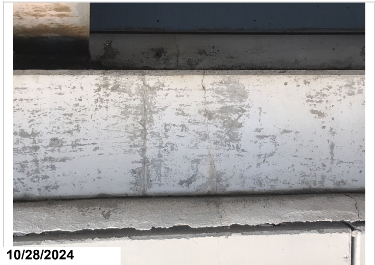
Bent 1 abutment has 15' of cracking CS2
