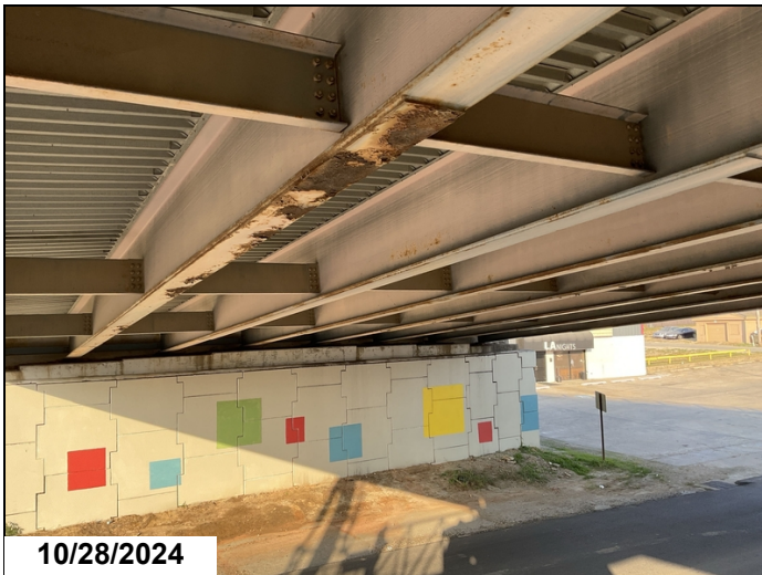
Span 1 girder 7 corrosion with minor section loss CS3
