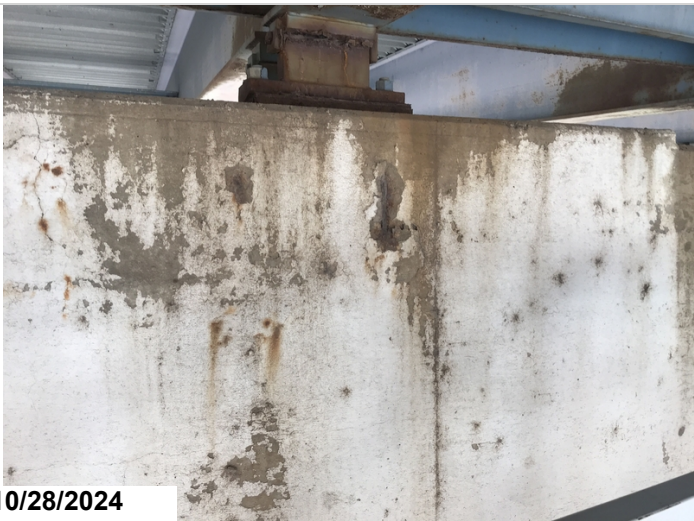
Bent 3 cap has 3' of delamination CS2 and 2' of spall with exposed rebar CS2 and 2' of cracking CS2
