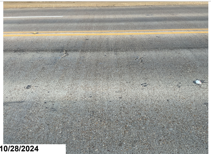
Span 2 East bound delam/shallow spalls
