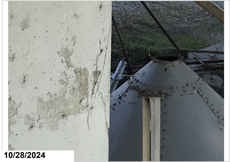
Bent 3 column 2 ahead has a 3' vertical crack under cap CS3
