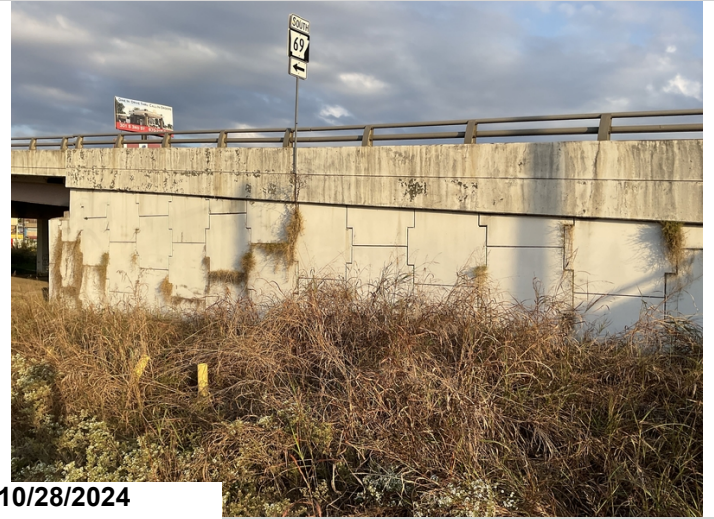
Bent 10 Rt vegetation in mse joints
