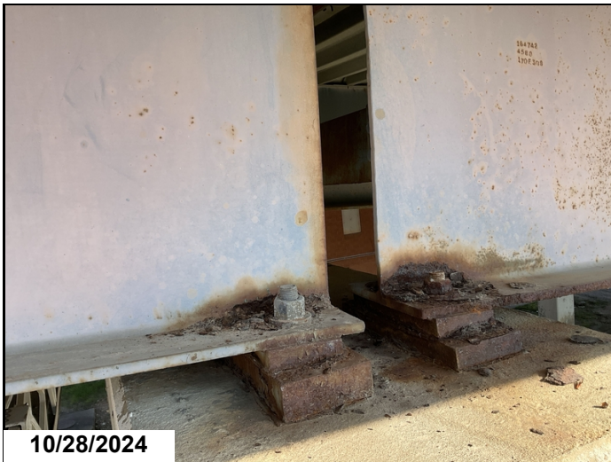
Span 7 bent 8 girder 8 and Span 8 bent 8 girder 8 have 6" areas of 1/8" section loss at bottom of web over bearings. CS3
