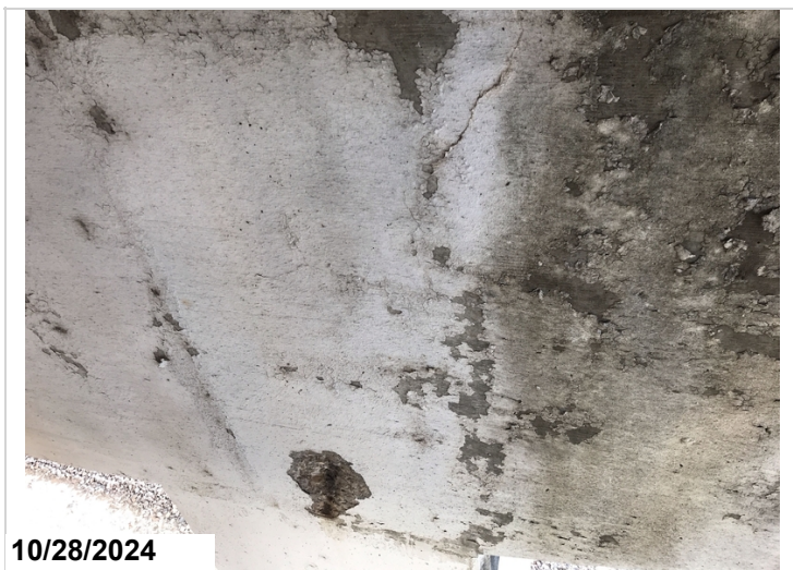
Bent 5 cap has 1' spall with exposed rebar CS2 and 1' of cracking CS2
