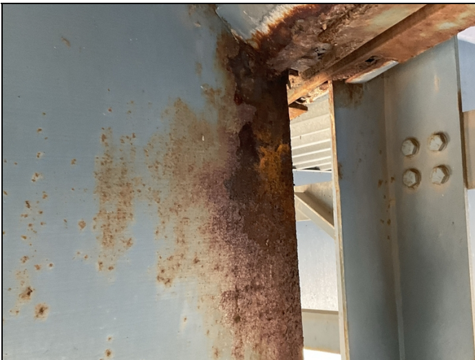
Span 6 bent 6 girder 5 has some minor flaking rust in web below haunch
