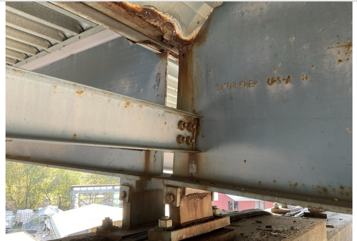
Typ corrosion at ends
