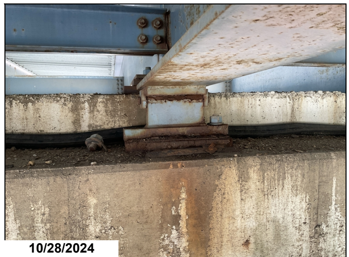
Span 6 bent 7 bearing 6 has 1 anchor bolt sheared off
