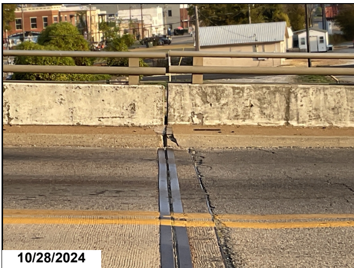
Typical settlement at bents 1 and 10
