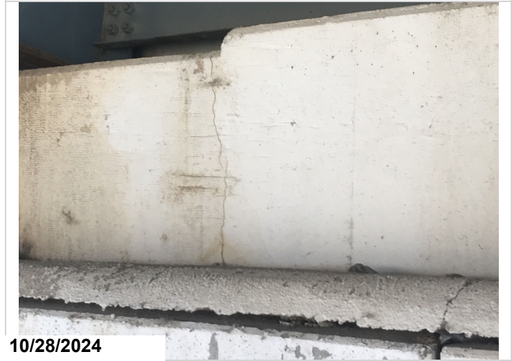
Bent 10 abutment has 16' of cracks CS2
