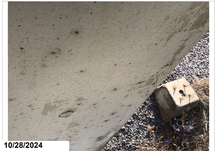
Bent 5 column 3 back has a 2' vertical crack 3' from bottom of cap CS2
