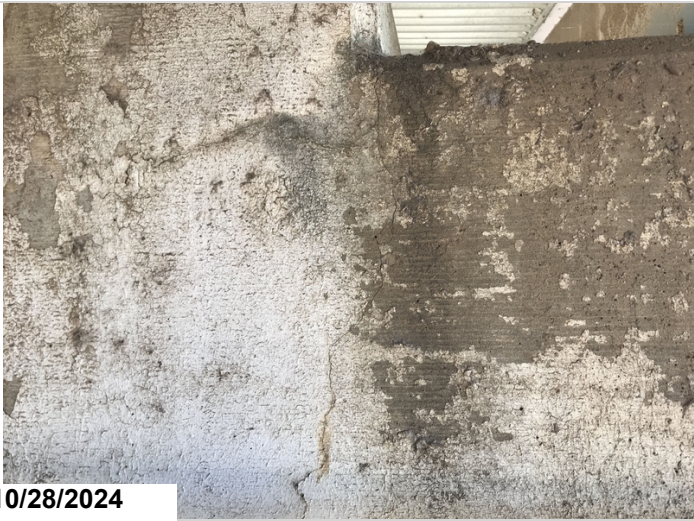
Bent 4 cap has 1' of cracking CS2
