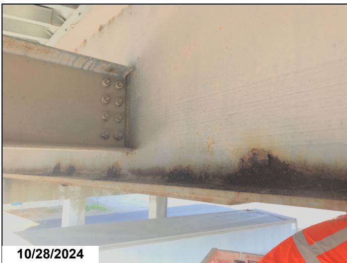
Span 2 girder 7 Rt side corrosion
