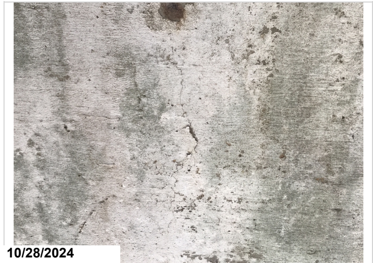
Bent 7 cap has 2' cracking CS2 and 1' delamination CS2
