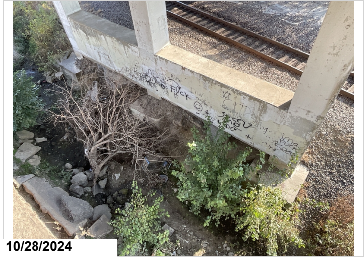
Bent 5 back footings exposed
