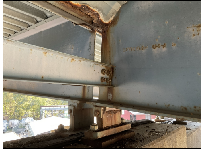
Typ corrosion at ends
