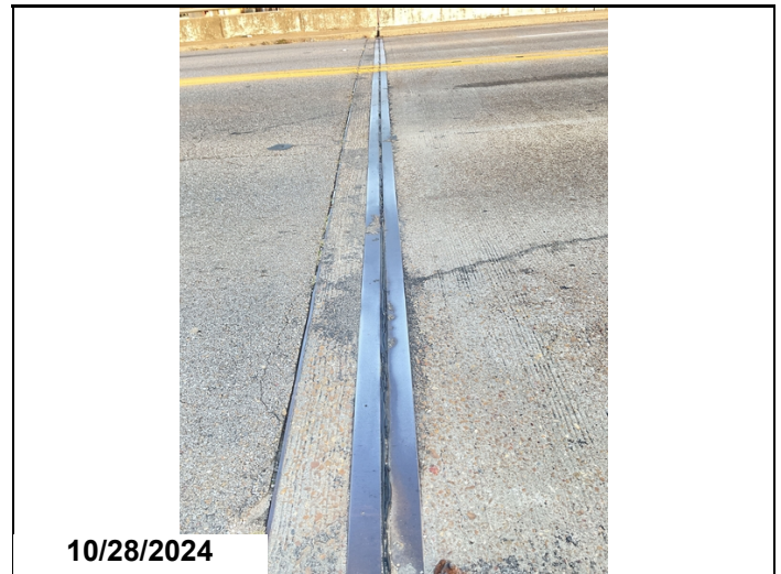
Bent 1, 3, 4, 8, 9, 10 joint torn
