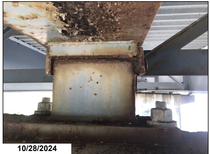
Span 6 bent 6 bearing 5 retainer is bowed from pack rust at cap screw. CS3
