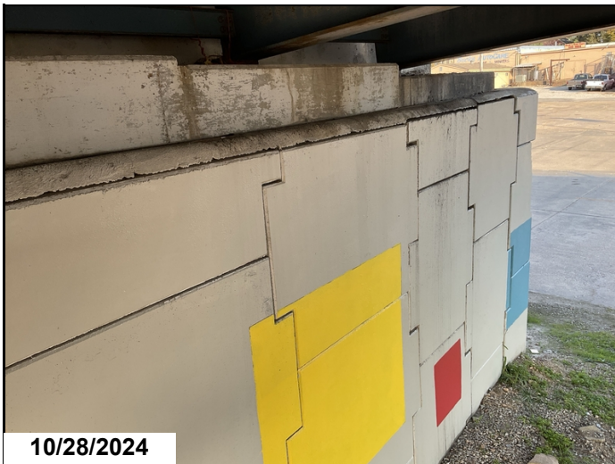
Bent 1 Lt MSE wall settlement at top corner
