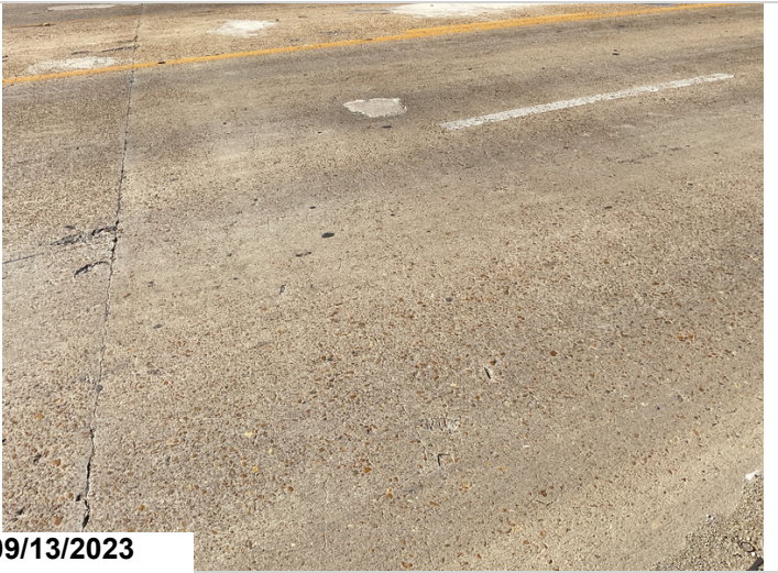
Span 1 cracks
