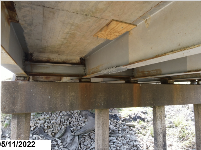
Bent 2 girder repairs
