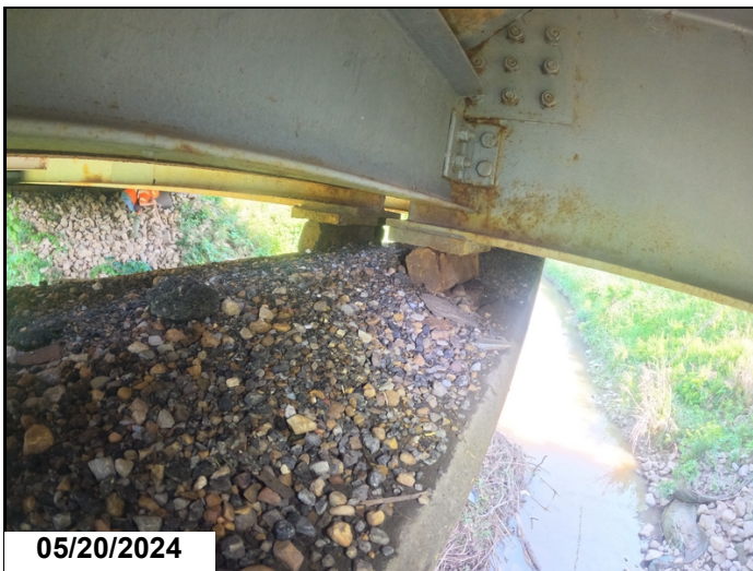
Span 2, Bent 2, Girder 4: bearing rotation
