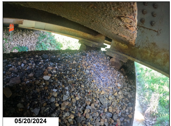
Span 2, Bent 2, Girder 3: bearing rotation
