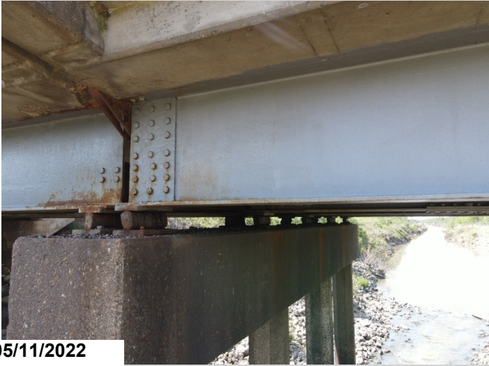
Span 1 bent 2 girder 1 repair
