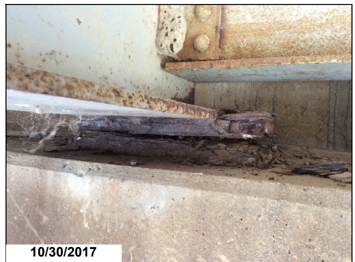
Span 2, Bent 2, Girder 3: bearing rotation
