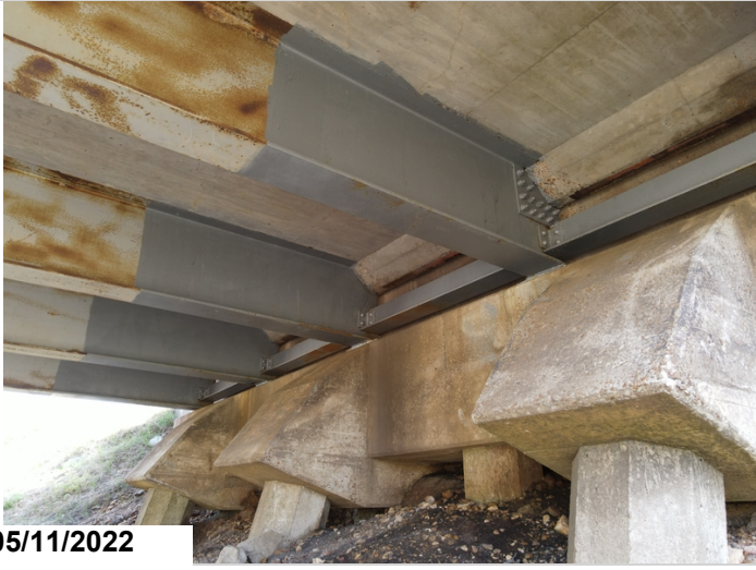
Bent 3 girder repairs
