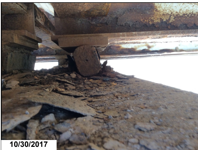
Span 2, Bent 2, Girder 4: bearing rotation
