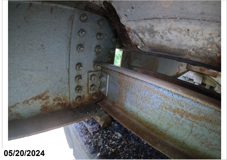
Span 1, Bent 2, Girder 1: bolted web splice
