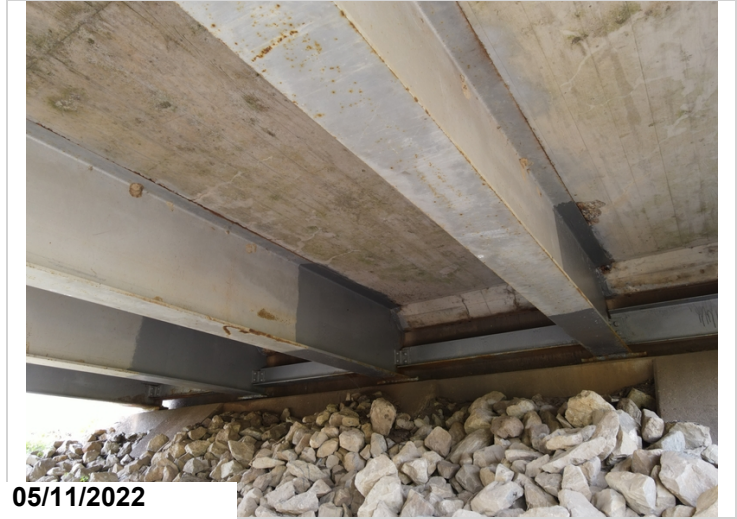
Bent 1 girder repairs
