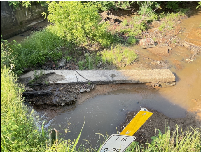
old wing wall footing left in place
