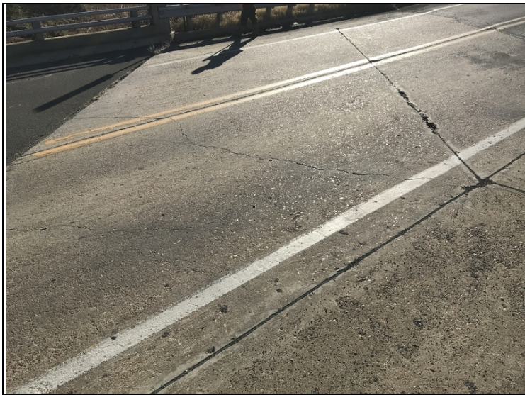
Approach slab cracks
