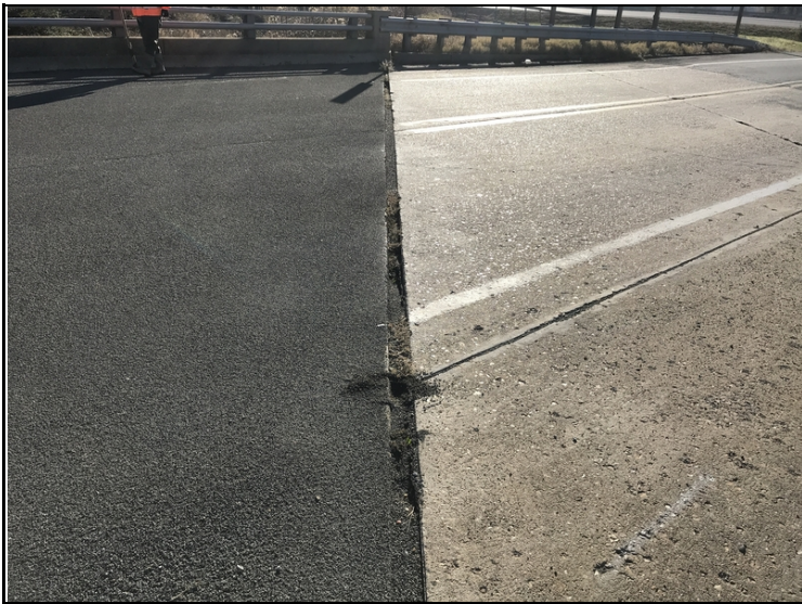
Typ gap at approach slabs
