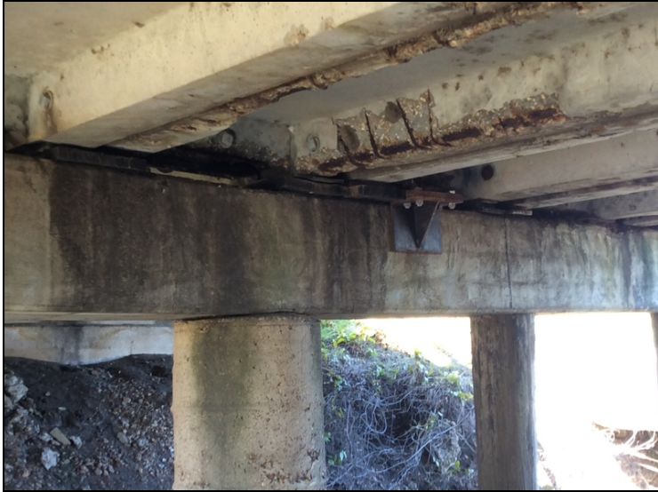
Bent 3 cap repair span 2 side.
