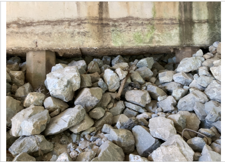
Bent 4 Scour with exposed piles
