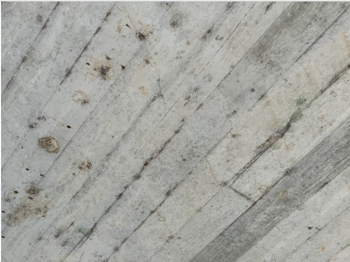
Span 2 Cracking in undersurface
