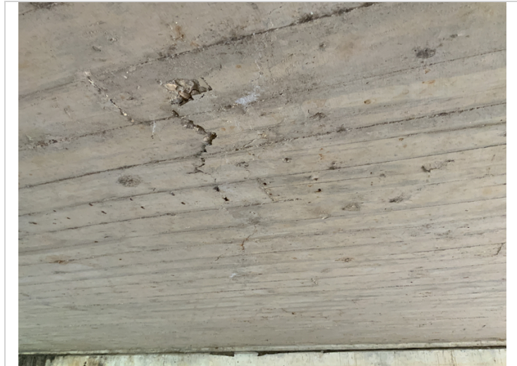
Span 1 Delaminating at mid span
