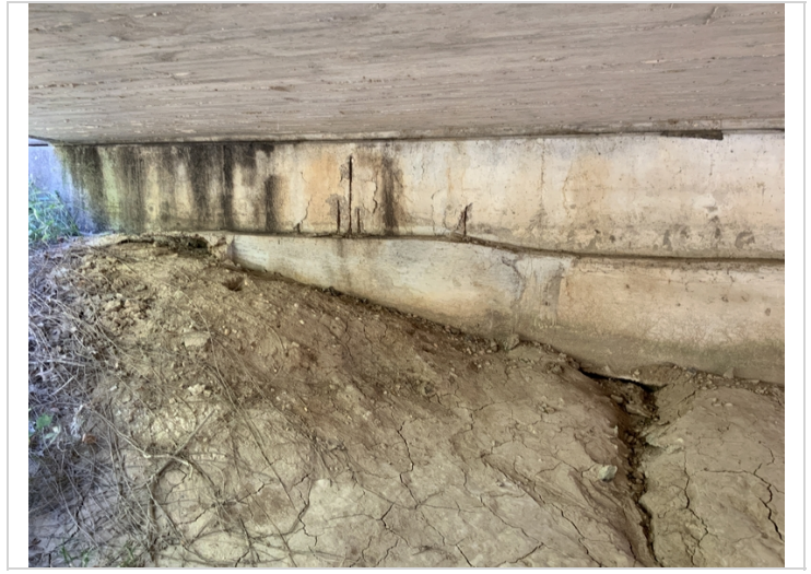
Abutment 1 Spalling with exposed reinforcing steel
