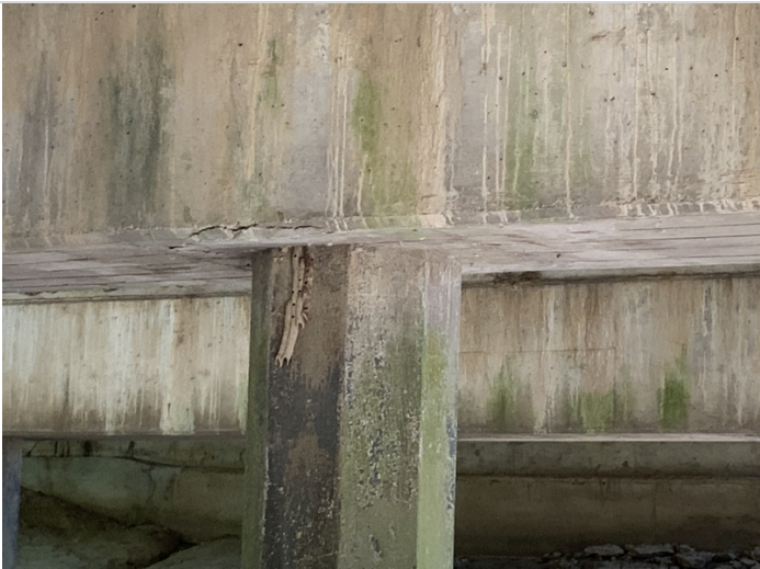
Bent 3 Above column 3 cracking
