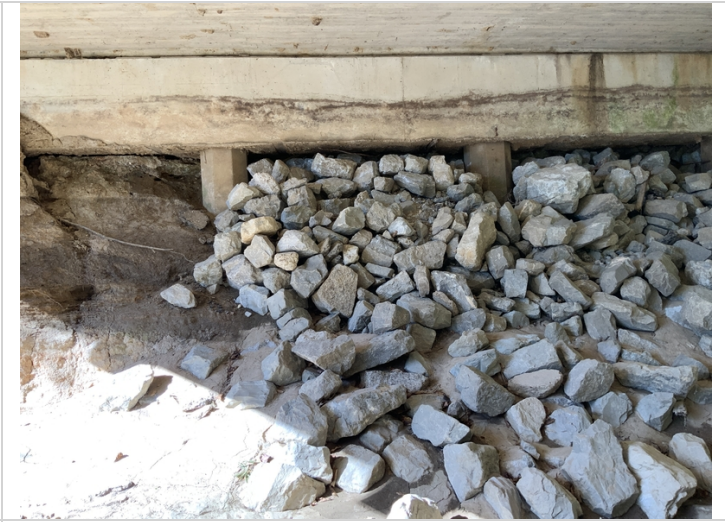
Abutment 2 Scour countermeasures failing
