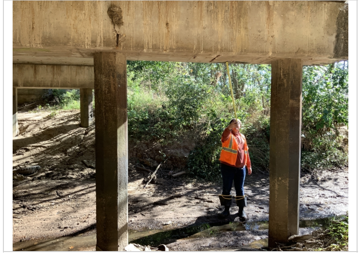
Bent 3 Spalling with exposed reinforcing steel
