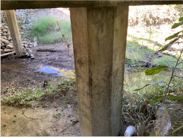
Bent 2 Column 5 Cracking
