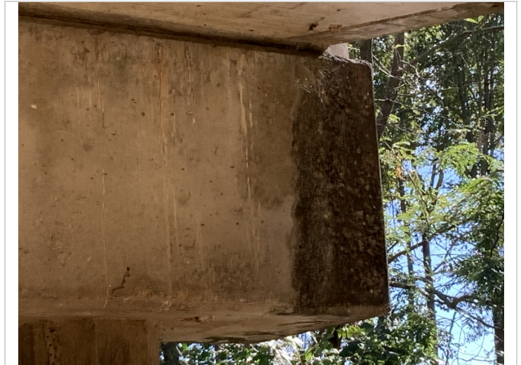
Bent 3 Abrasion on end of caps
