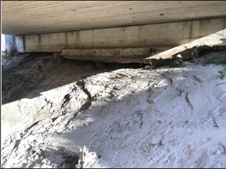
Bent 1 erosion
