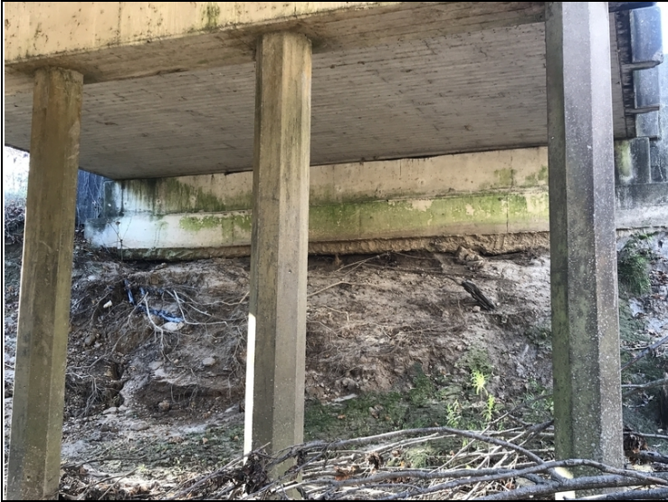
Bent 4 erosion 2020
