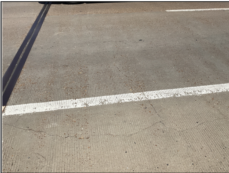
deck cracks
