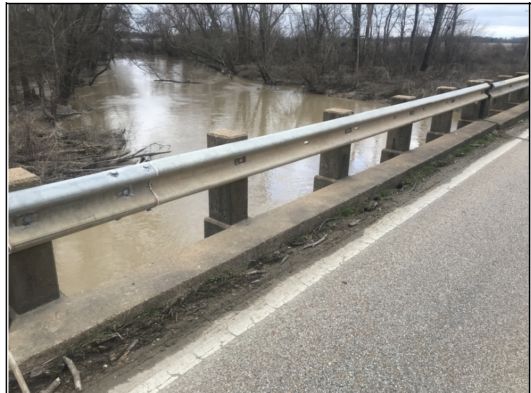
Span 13 rail right repaired
