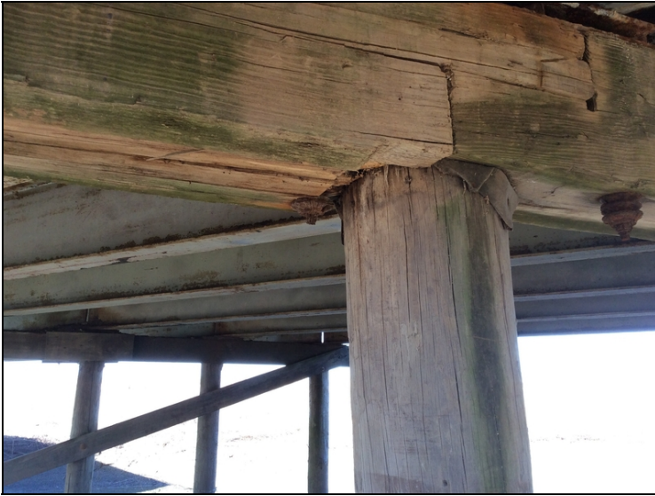
Bent 3 cap at splice over pile 3.
