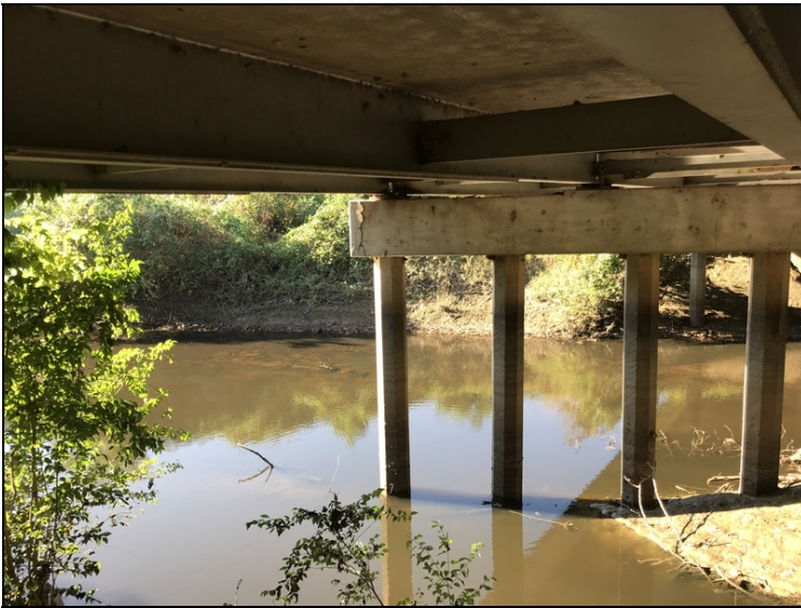
S3 b3 cap delamination and spall
