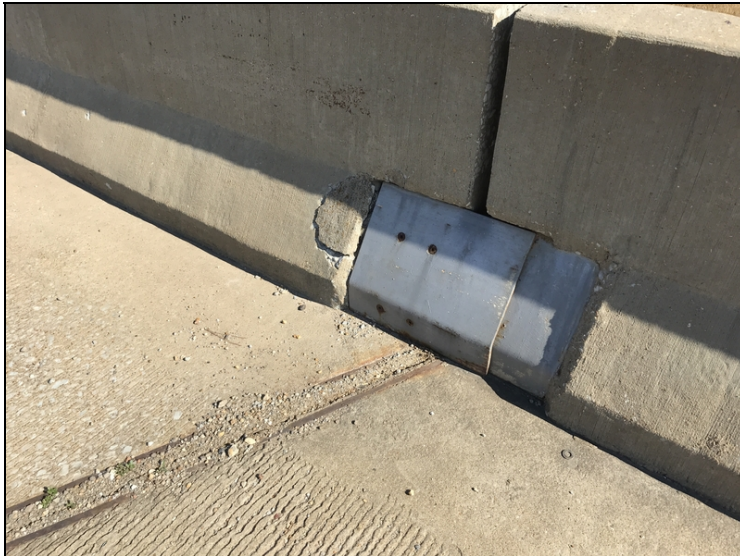
Delamination in rail at bent 4 2019
