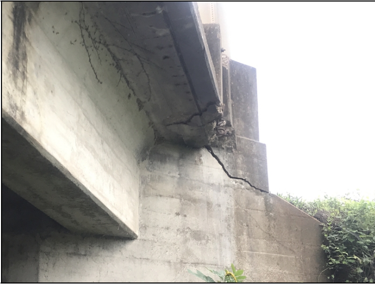
Span 1 right side bent 2 rail & soffit 2019
