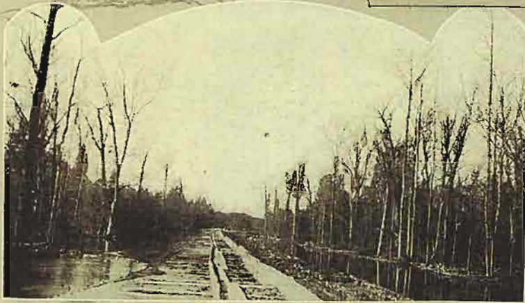
Temporary Relief for Traffic on Route No. 4, in Drew County.
