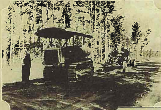
Maintenance equipment at work in Drew County.
