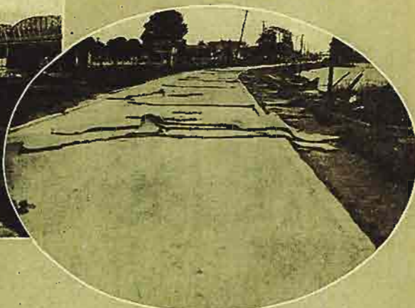
Route No. 65, in Desha County, showing how asphalt was stripped from the concrete base.
