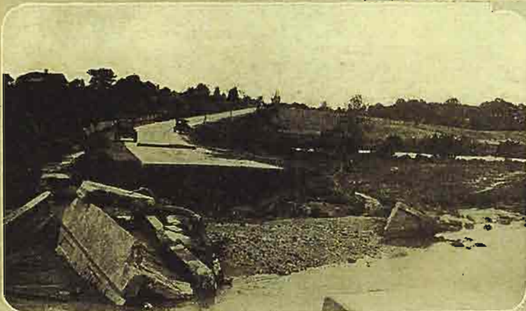
Concrete Bridge washed away on Hot Springs-Little Rock Road, in Saline County.
