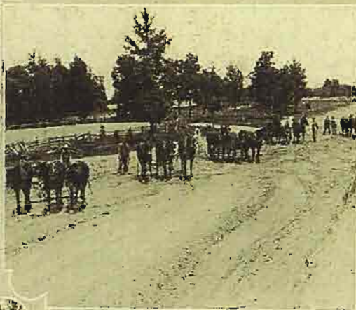
Finishing crew on a grading job on Route 70, in Pike County.
