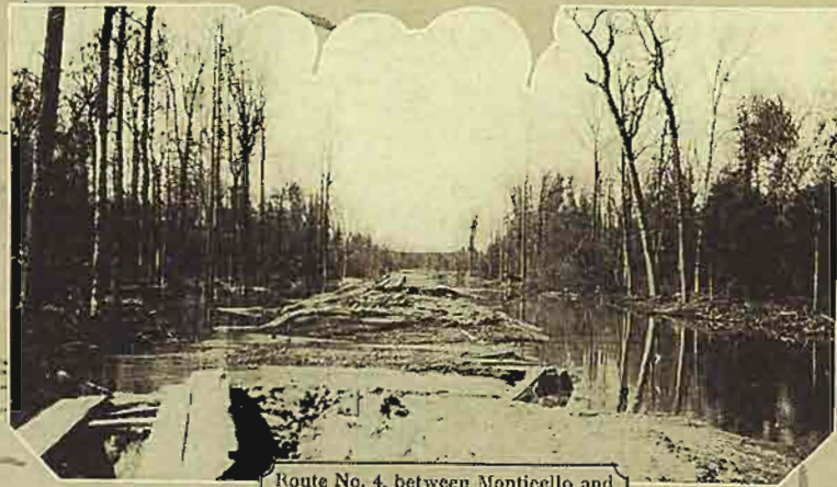
Route No. 4, between Monticello and Tillar, Drew County.
