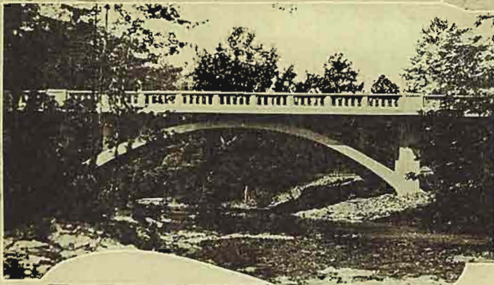
Recently completed bridge across Harp Creek, north of Jasper, in Newton County.
