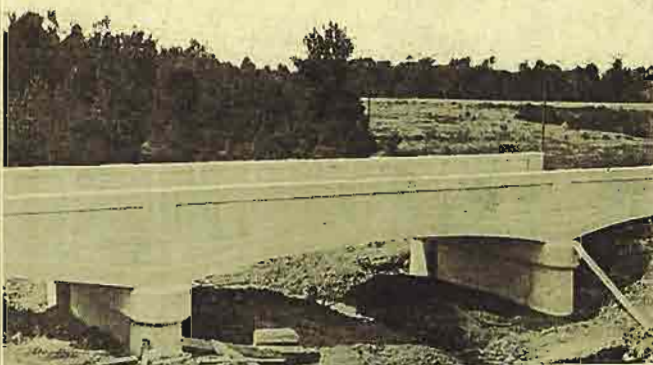
New concrete Bridge across Ditch No. 9, southeast of Marked Tree, in Poinsett County.
