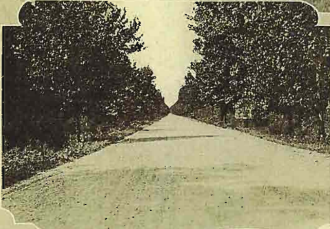
Route 14, between Harrisburg and Marked Tree, in Poinsett County.
