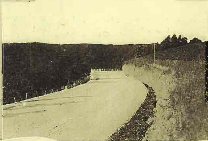
Widened road northeast of Eureka Springs, in Carroll County.
