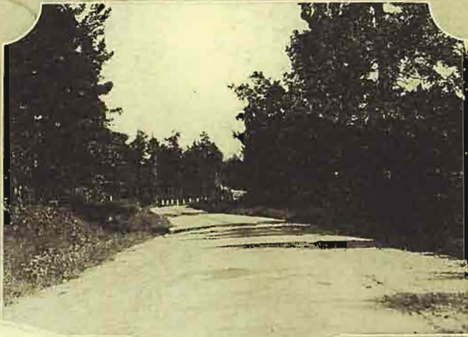
The old Dollarway in Jefferson County. The first improved road built in the State. This road has been relocated and work is now under way on the grading and drainage structures.
