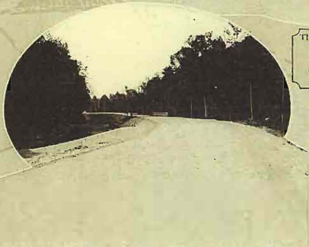
One mile north of Lonoke, on the Lonoke-Beebe Road. A most excellent example of good grading and gravel surfacing.
