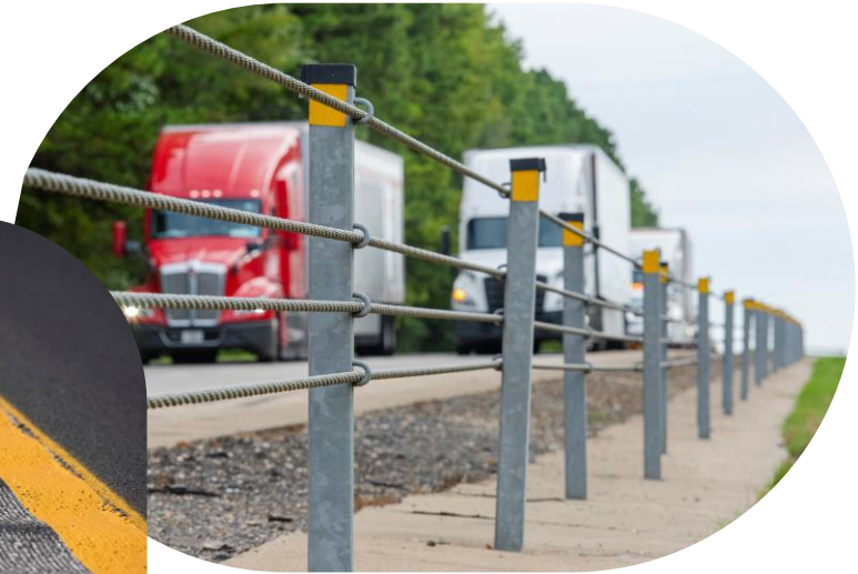
Cable median barriers & centerline rumble strips
