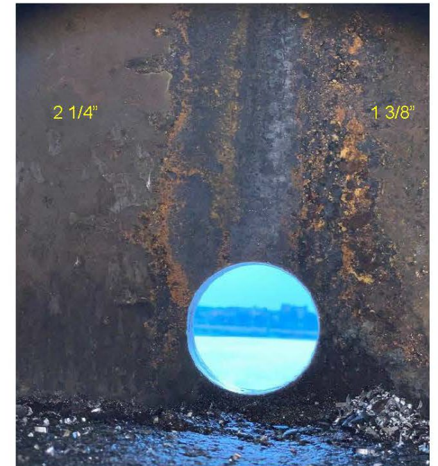
Figure 15. View from inside tie showing core sample removed from groove weld.
