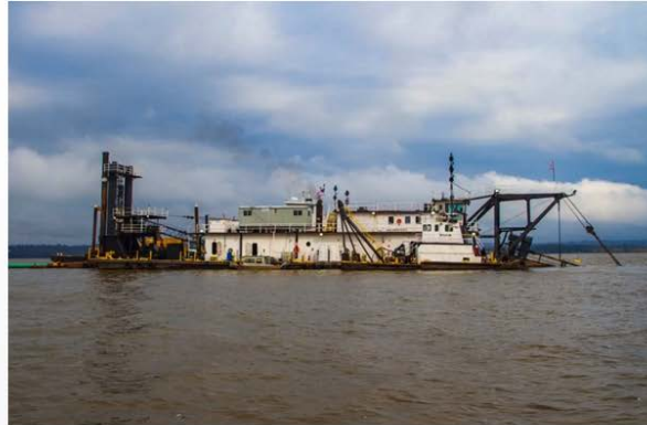
Dredging on Arkansas River in Little Rock District, Mile 222 (2019). Image Source: https://www.dredgingtoday.com/2019/11/11/arkansas-river-busy-with-dredging-operations/
