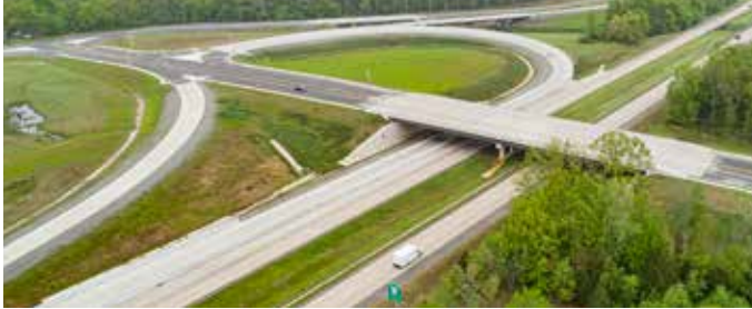
Highway 67 Interchange North of Cabot
