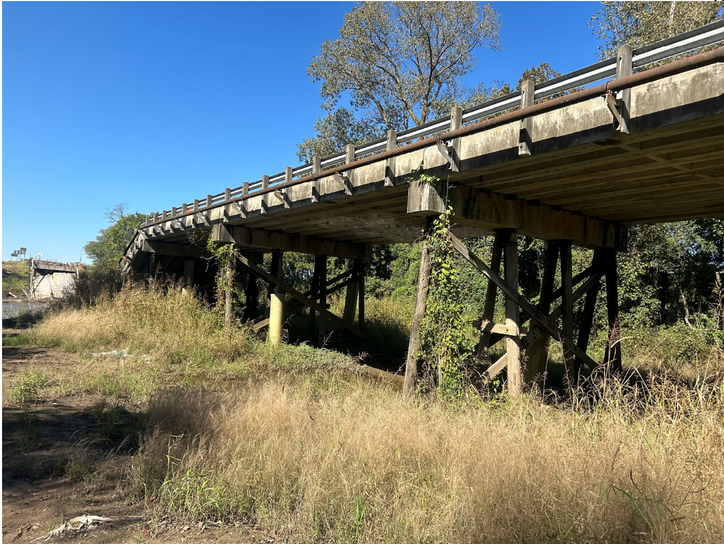
Looking northwest from the east bridge end (Early October 2024 Before Demolition)
