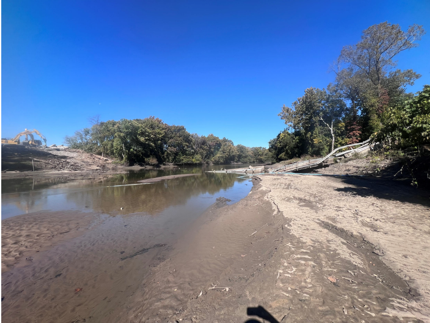
South side of east bridge end looking north (Late October 2024 During Demolition)
