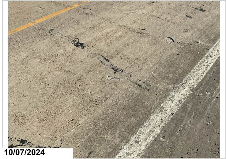
Typical deck crack
