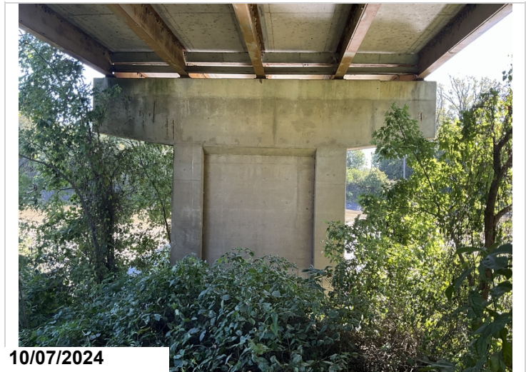
Bent 3, Cap, Back: Six 1' spalls with reinforcing steel exposed above left column and a 1' spall with exposed reinforcing steel on right side. Reinforcing steel has no section loss.
