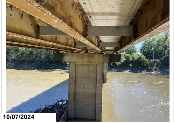
Bent 4, Cap, Back, Under Girder 4: 1' spall with reinforcing steel exposed. Reinforcing steel has minor section loss.
