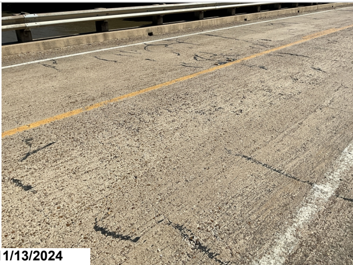
Typical deck abrasion
