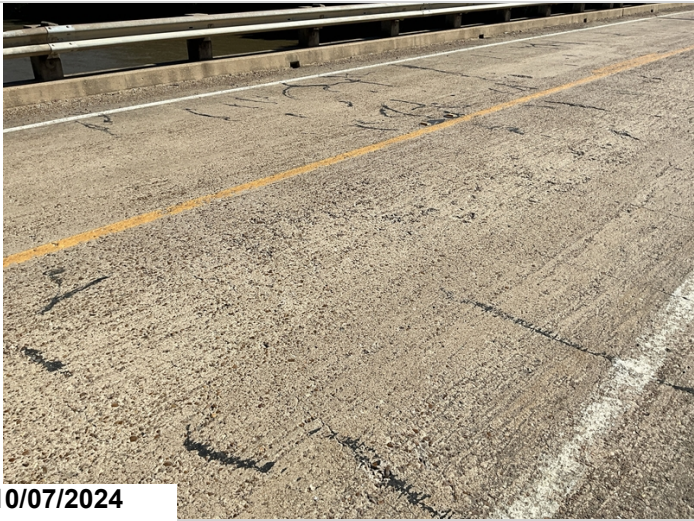
Typical deck abrasion
