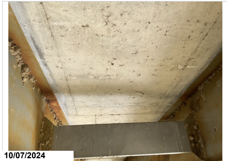
Span 5, Deck Undersurface, Bay 3, 1/4 Span: 1' delamination.
