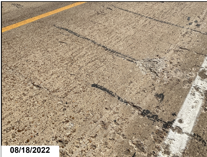
Typical scaling in span #3 deck
