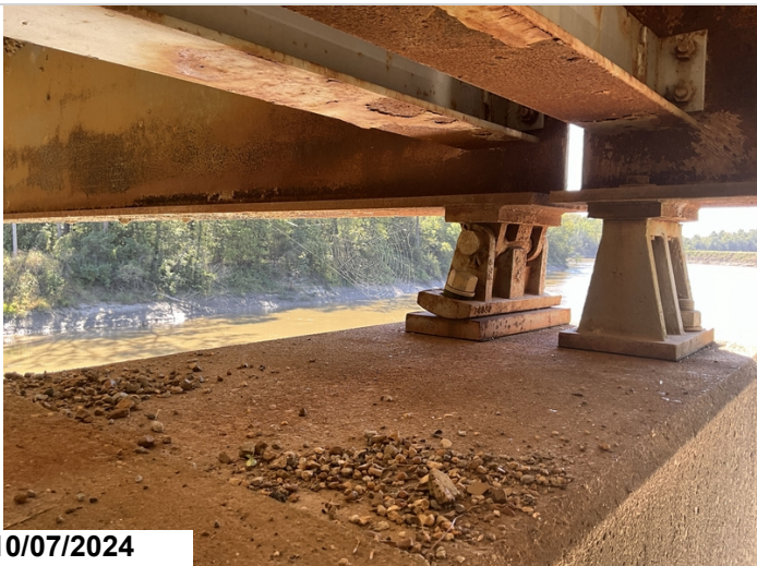
Bent 4, Span 4, Bearing 1: Rocked back 15 degrees.
