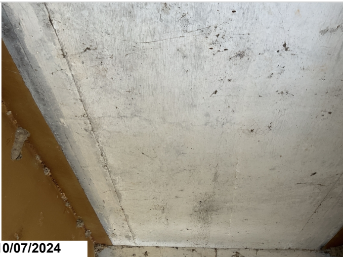
Typical deck undersurface crack
