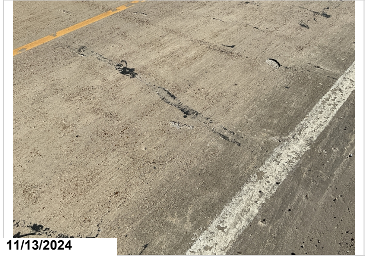
Typical deck crack
