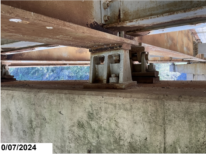
Typical fixed bearing
