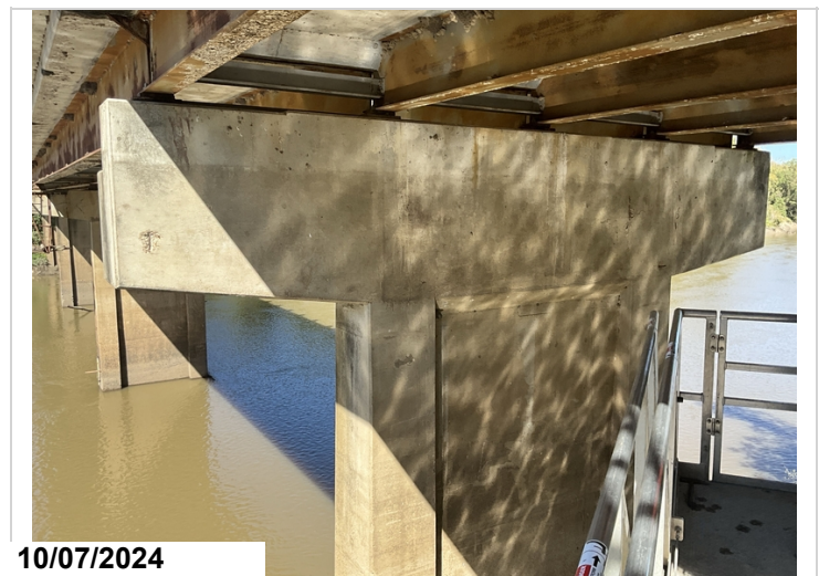
Bent 6, Cap, Ahead: 3' of exposed reinforcing steel due to poor concrete coverage. Reinforcing steel has moderate section loss.
