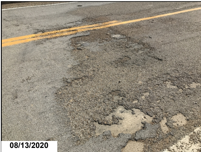
Wearing Surface, Span 7, Near Bent 7: 40 square feet of rough area.
