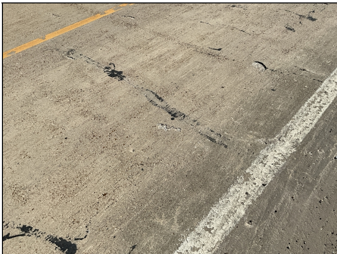
Typical deck crack
