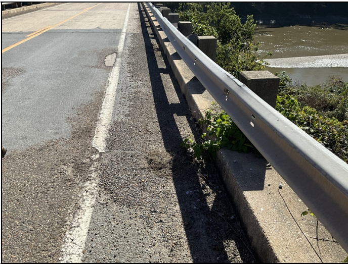
Deck Gutters: Dirt and debris.
