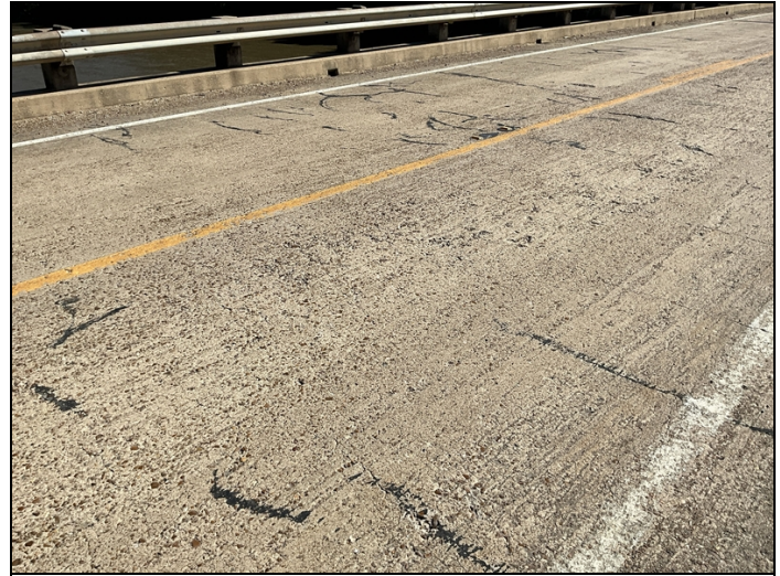
Typical deck abrasion
