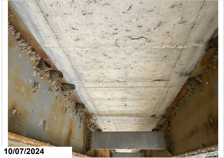
Typical crack with efflorescence span 5
