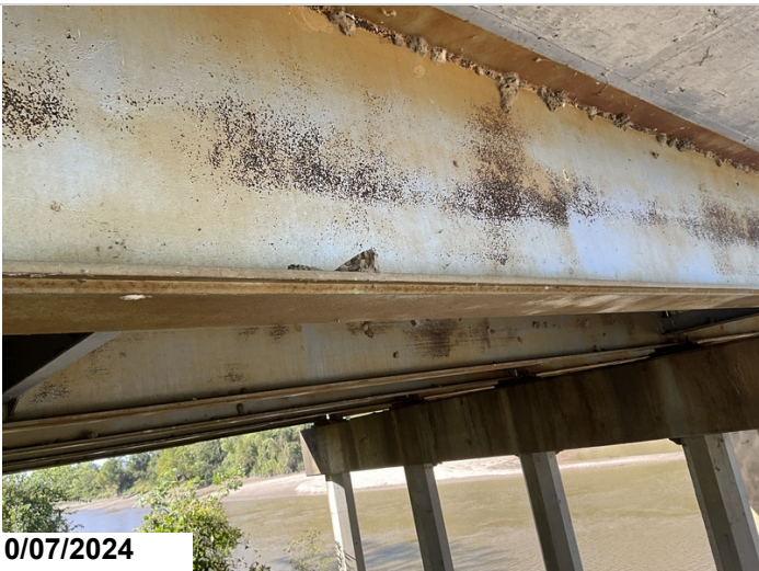
Typical girder condition
