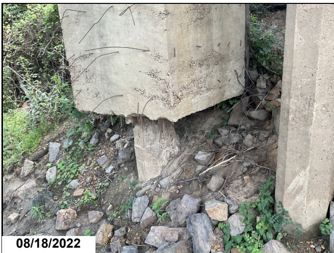
Bent #7 pile #1 repair undermined
