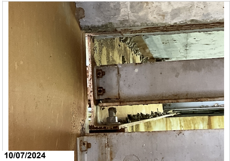
Span 2, Girder 3, Bent 3: Web is bent on end.
