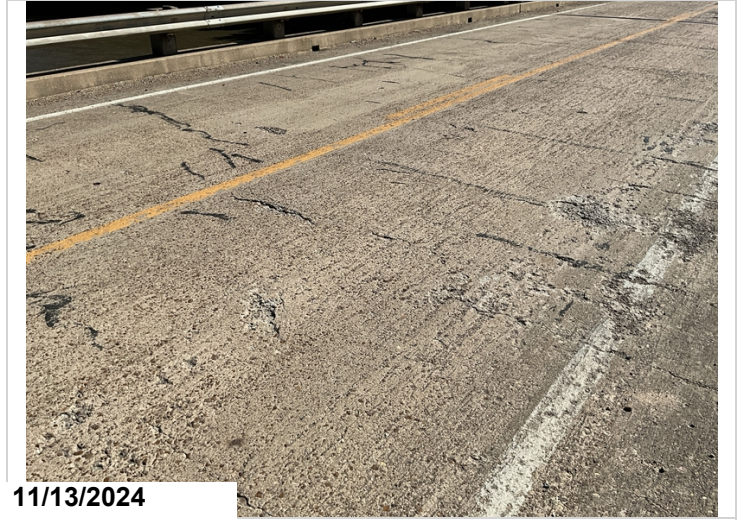
Typical deck spalls
