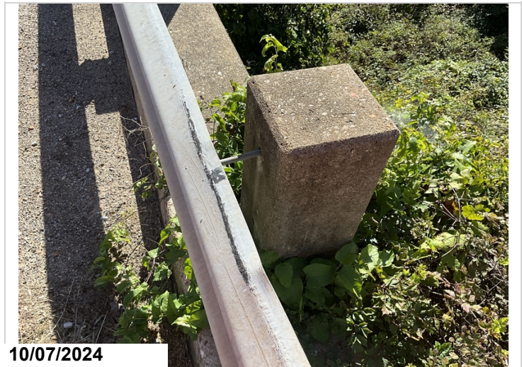
Typical bridge rail block broken missing
