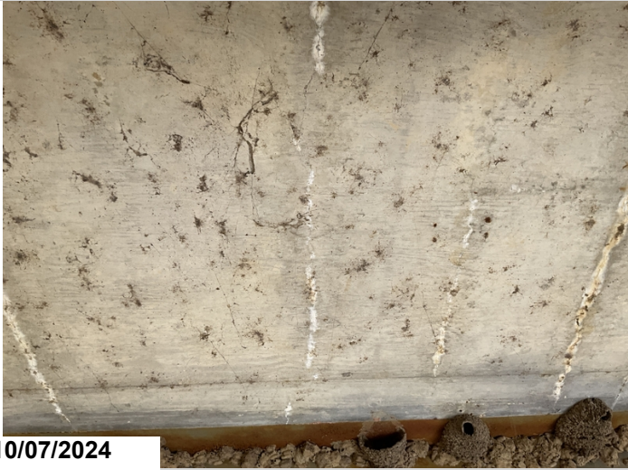
Span 5, Deck Undersurface, Bay 4, 1/4 Span: 1' delamination.
