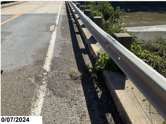
Deck Gutters: Dirt and debris.
