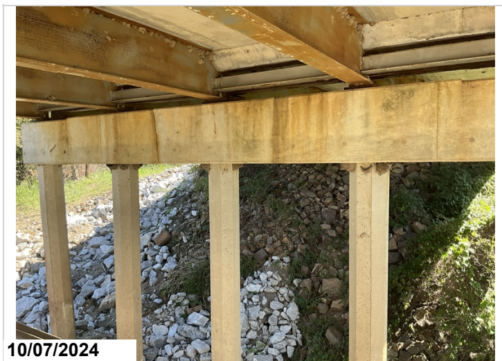
Bent 7, Cap, Back: 1' of exposed reinforcing steel due to poor concrete coverage. Reinforcing steel has moderate section loss.
