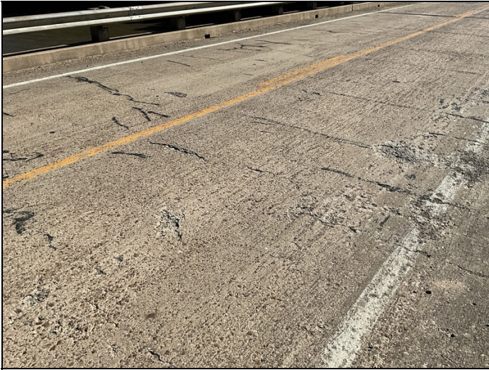
Typical deck spalls
