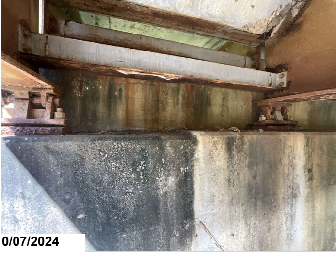
Bent 3, Cap, Ahead: 3' exposed reinforcing steel due to poor concrete coverage. Reinforcing steel has minor section loss. Bent 3, Cap, Ahead: 8' of longitudinal cracking.
