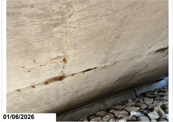
Span 1, near center: typical cracking with rust stains.
