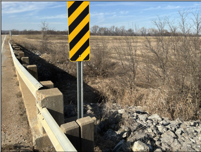
Abutment 2: log mile sign missing.
