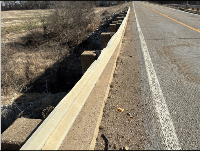
Dirt and debris in gutters.
