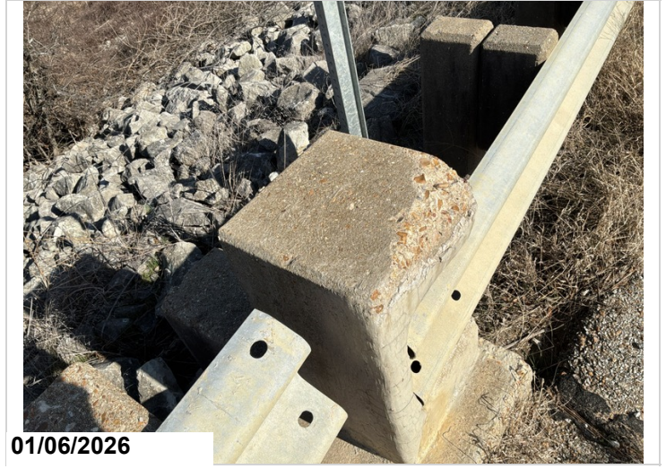
Bridge rail, monument post, abutment 2, left side: spall for 1'.
