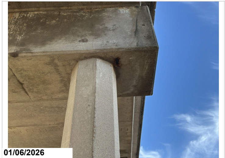
Bent 3, cap, bottom face, left side of pile 1: 6" spall with exposed reinforcing steel.
