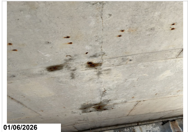
Span 4, center span: typical longitudinal cracks with rust stains.
