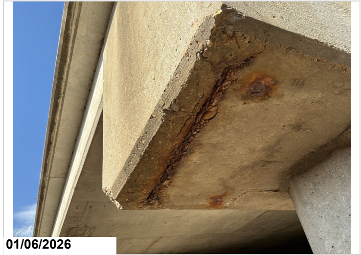
Bent 2, cap, bottom face, right side: 2' spall with exposed reinforcing steel.
