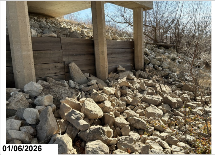
Wood back wall, ahead face of bent 2.
