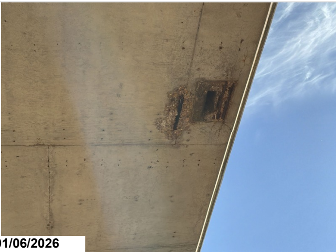
Span 3, right side, by drain: 1' spall with exposed reinforcing steel.
