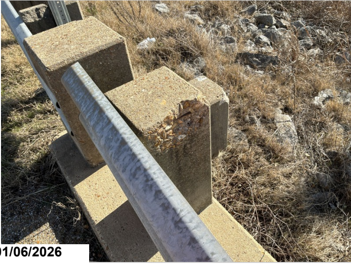
Span 4, right side, rail post 4: 1' spall with exposed reinforcing steel at top.
