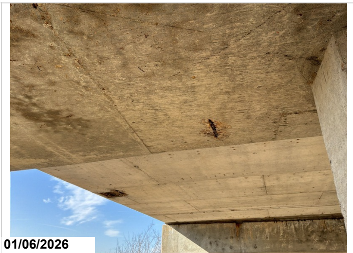
Bent 4, cap, bottom face, on each side of pile 3: delaminated for 6".
