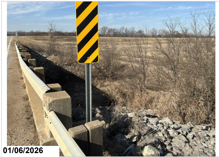
Abutment 2: log mile sign missing.
