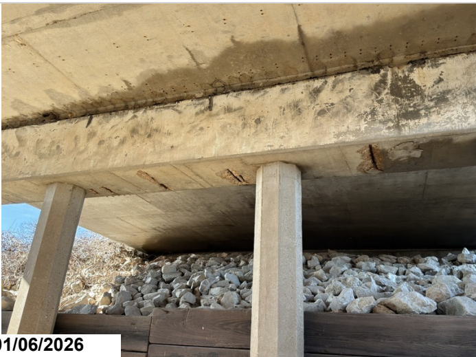
Bent 2, cap, bottom face, between piles 2 and 3: six 1' spalls with exposed reinforcing steel.
