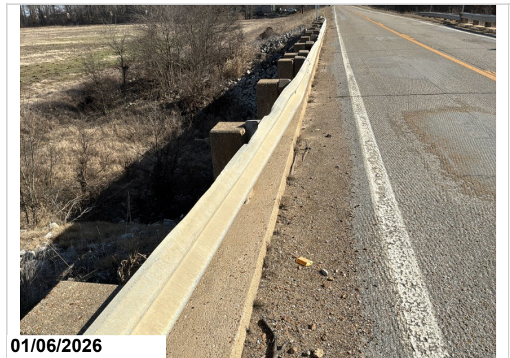
Dirt and debris in gutters.
