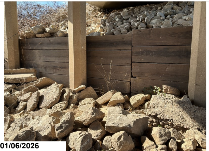
Wood back wall, behind backface of bent 2.
