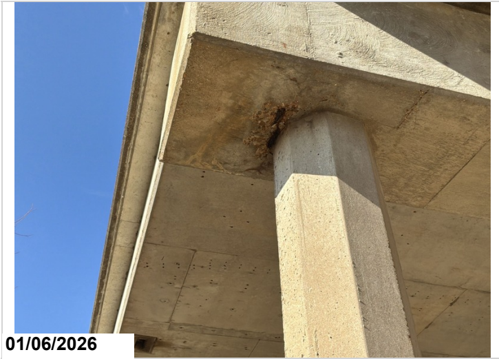
Bent 3, cap, on bottom face, right of pile 4: 1' spall with exposed reinforcing steel.
