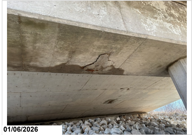
Bent 4, between piles 1 and 2, bottom face: cracked and delaminated for 2'.
