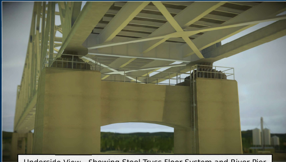
Underside View - Showing Steel Truss Floor System and River Pier
