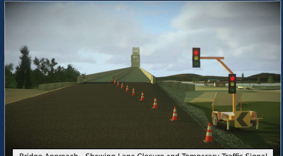
Bridge Approach - Showing Lane Closure and Temporary Traffic Signal
