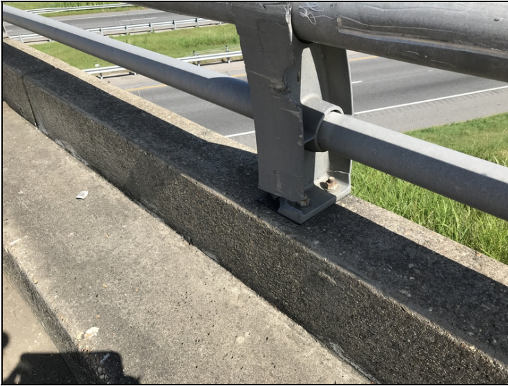
Span #1 right metal second rail post is broken at base.
