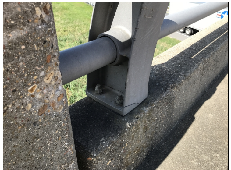
Span #1 left metal first post is cracked at base.
