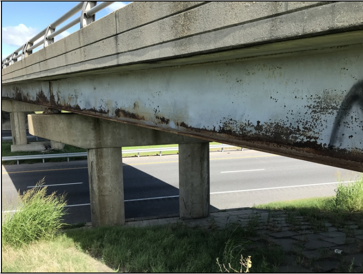
Typical paint condition outside girders.
