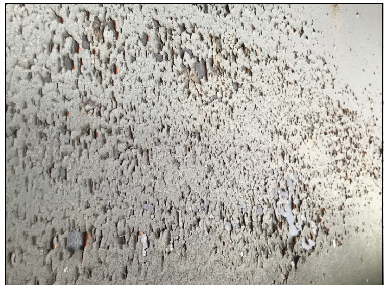
Typical peeling paint on girders.
