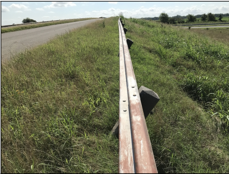
Abutment #2 left approach rail is leaning out.
