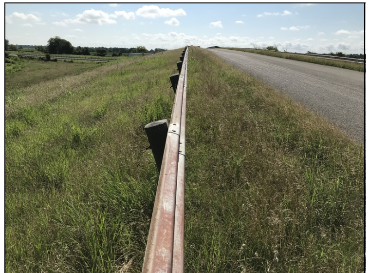
Abutment #2 right approach rail is leaning out.
