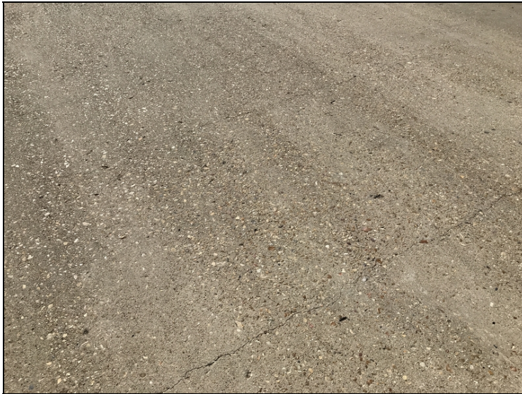
Typical deck cracks.
