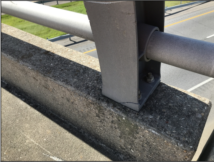
Span #3 left bridge rail ninth metal post is cracked at base.
