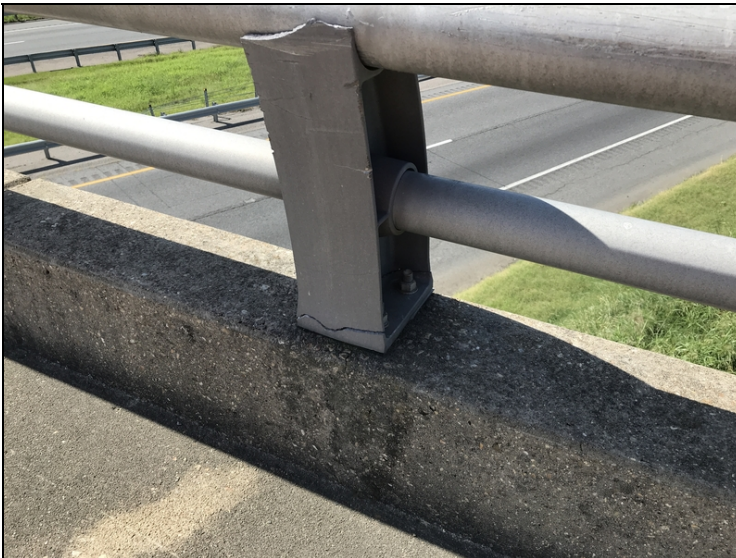
Span #4 left side third metal post is cracked at base.
