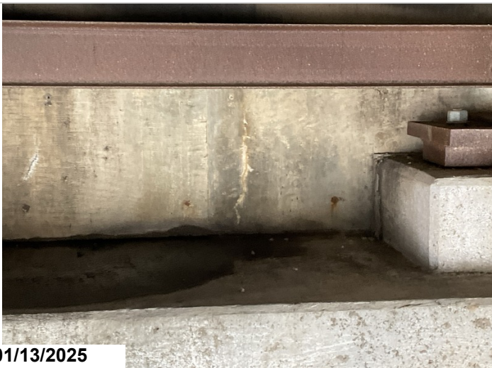
Typical vertical crack in abutment back wall with light efflorescence.
