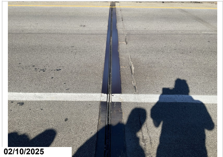
Abutment 2, joint seal: 10' of lost adhesion with minor sagging.
