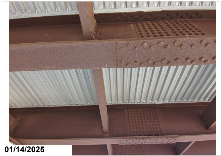
Span 2, girder 4, first bottom splice plate: one bolt missing.
