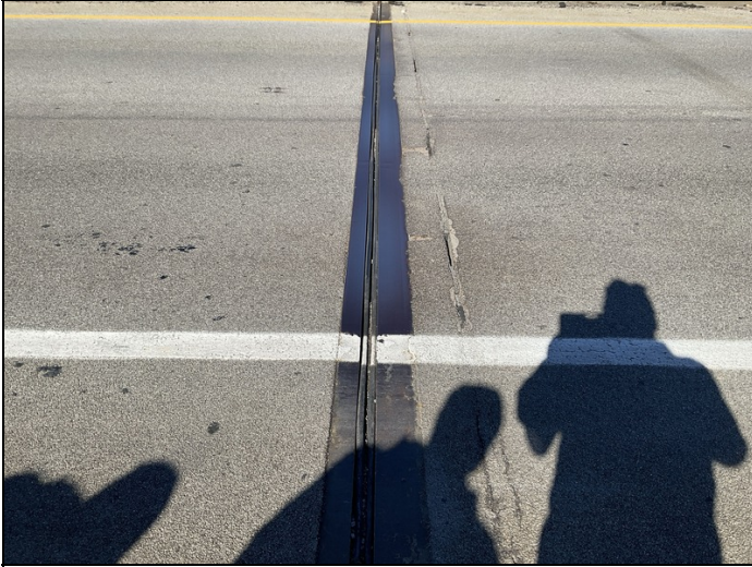
Abutment 2, joint seal: 10' of lost adhesion with minor sagging.
