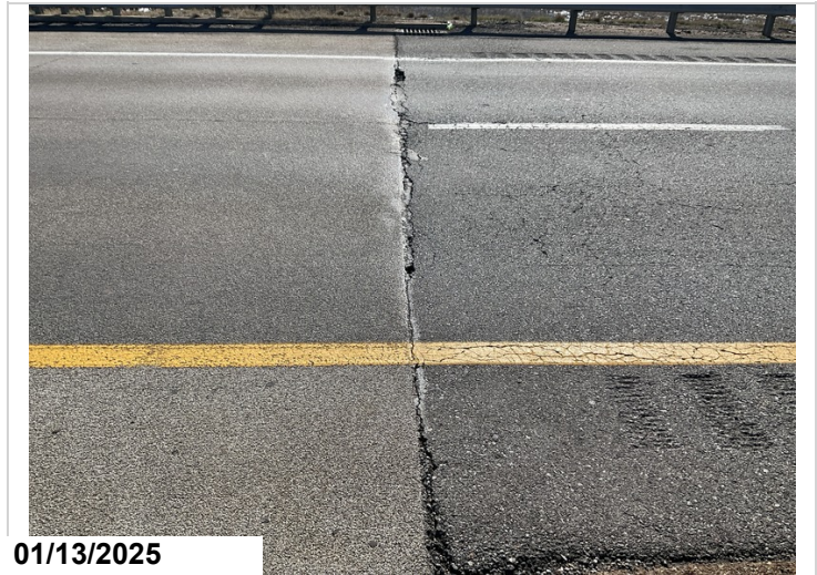
Abutment 1, approach roadway: pavement raveling at joint with approach slab.
