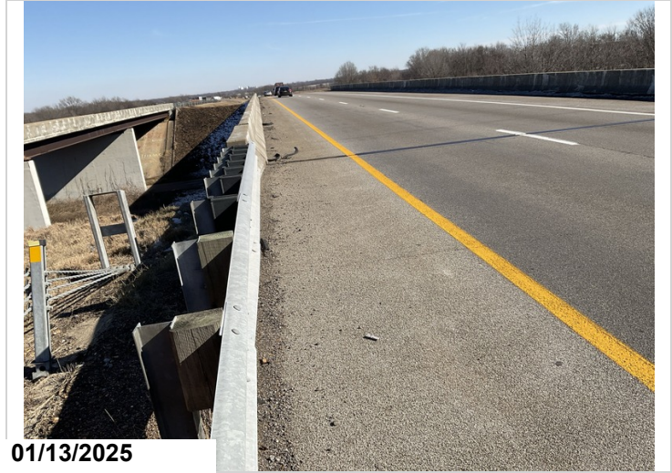
Dirt and debris in gutters.
