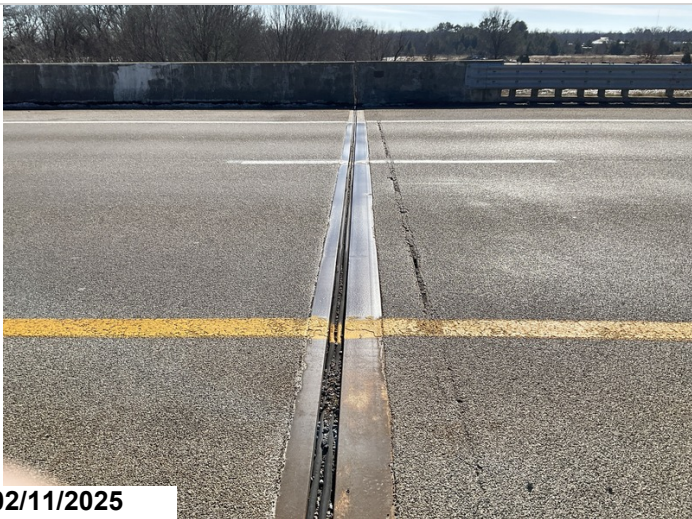
Moderate debris impact in joints along shoulders.
