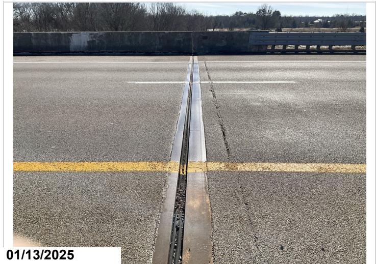
Abutment 1, joint seal: 15' lost adhesion and sagging.
