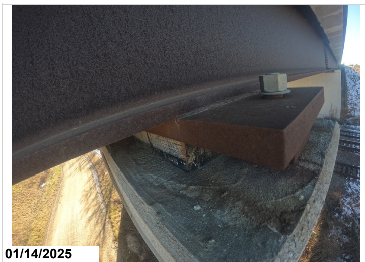
Typical intermediate bearing.
