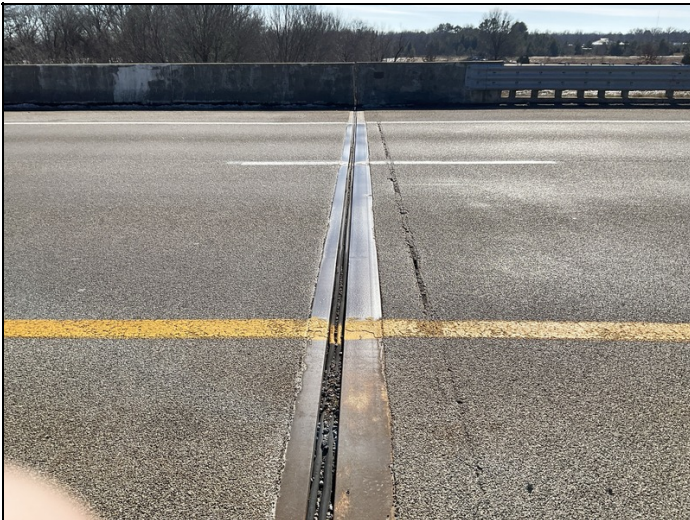
Moderate debris impactation in joints along shoulders.
