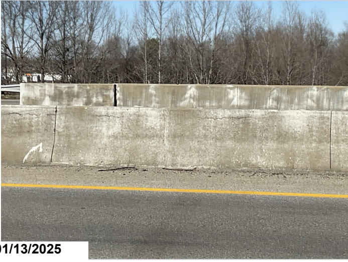
Typical longitudinal cracking in left bridge rail.
