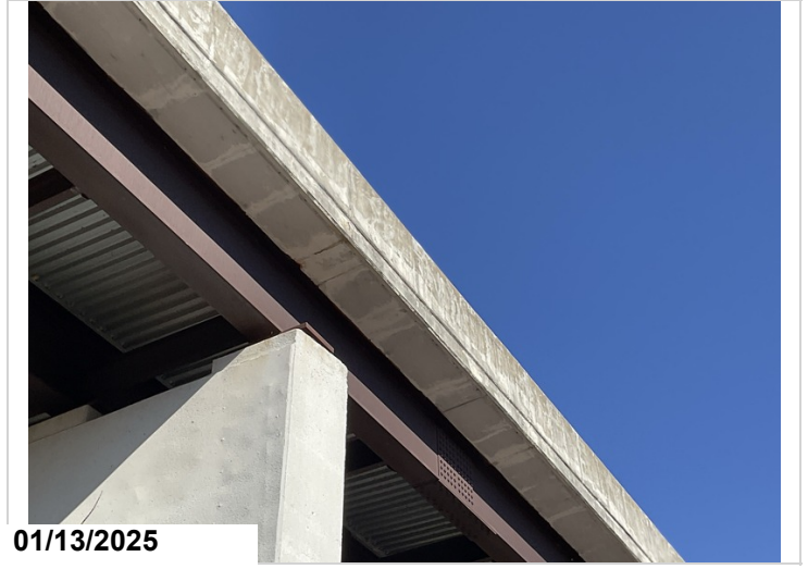
Typical cracking in overhang.
