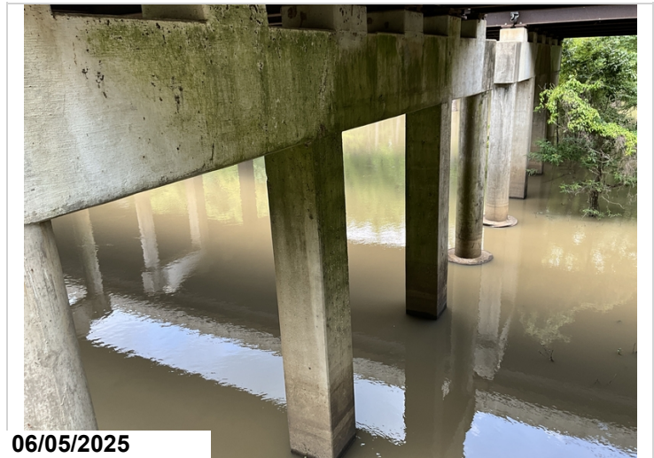
Bent 16, Column 2: Cracks and delaminations.
