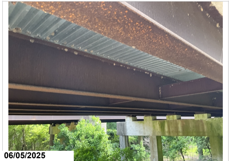
Typical girder condition
