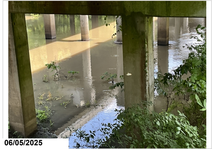
Bent 14, Column 3: Cracks and delaminations.
