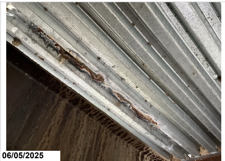
Typical stay in place form corrosion
