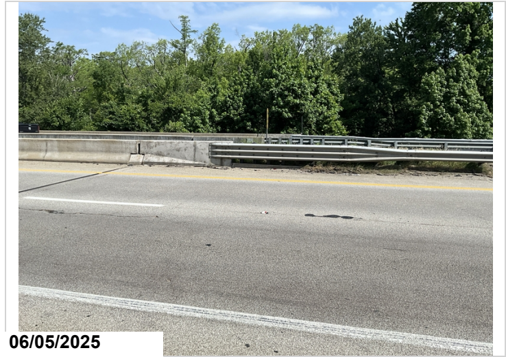
Typical approach rail transition
