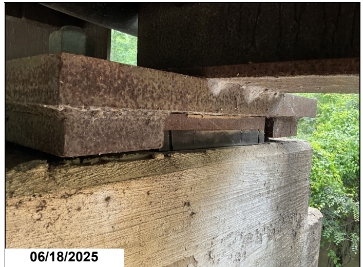
Span 14, Bent 15, Bearing 4: Bearing has twisted and moved back but still under girder plate. Span 15, Bent 16, Bearing 6: Bearing has twisted and moved back but still under girder plate. Span 16, Bent 17, Bearing 4: Bearing has twisted and moved back but still under girder plate.
