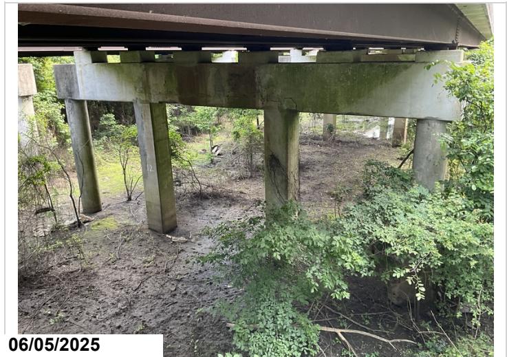
Cap, Bent 12, Bottom, Between Columns 2 & 3: 2' Cracks with delaminations.
