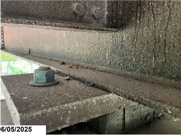
Bent 20, Girder 4, Girder To Soul Plate Weld: Not welded. Bent 20, Girder 5, Girder To Soul Plate Weld: Not welded.
