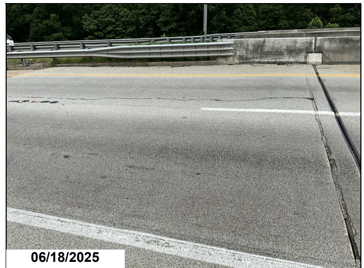
Abutment 1, Approach Slab, Left Lane: Full length longitudinal crack reflecting through overlay.
