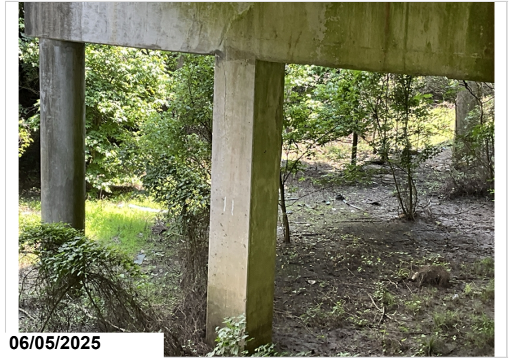
Bent 11, Column 2: Cracks and delaminations.
