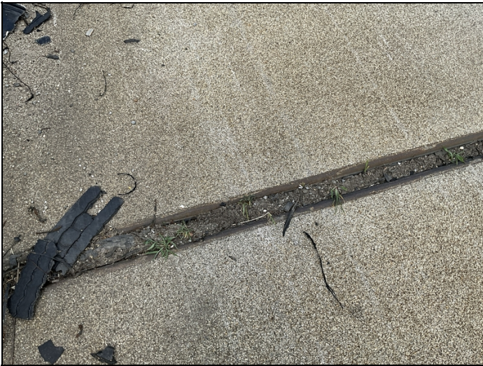
Typical debris in joints
