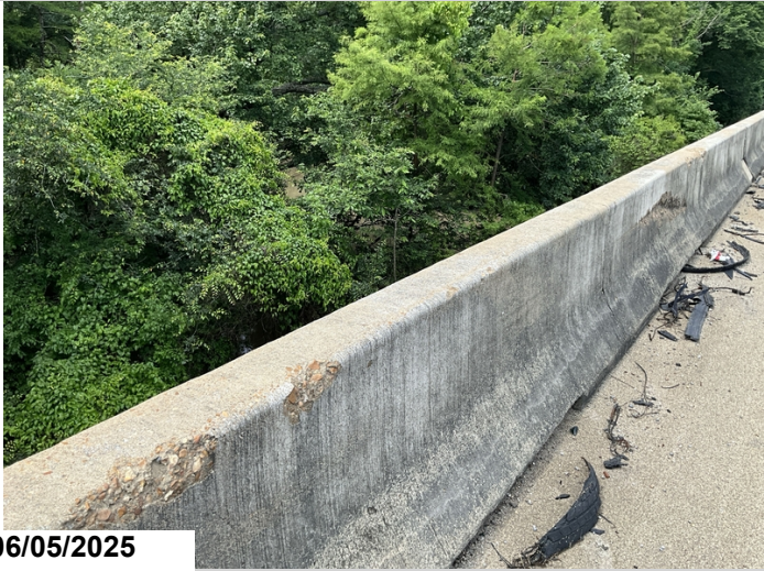
Span 18, Bridge Rail, Right: 4' gouging due to collision damage.
