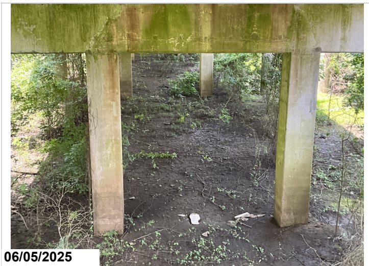
Bent 12, Column 1 & 2: Cracks and delaminations.
