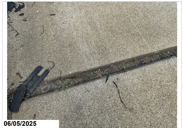
Typical debris in joints
