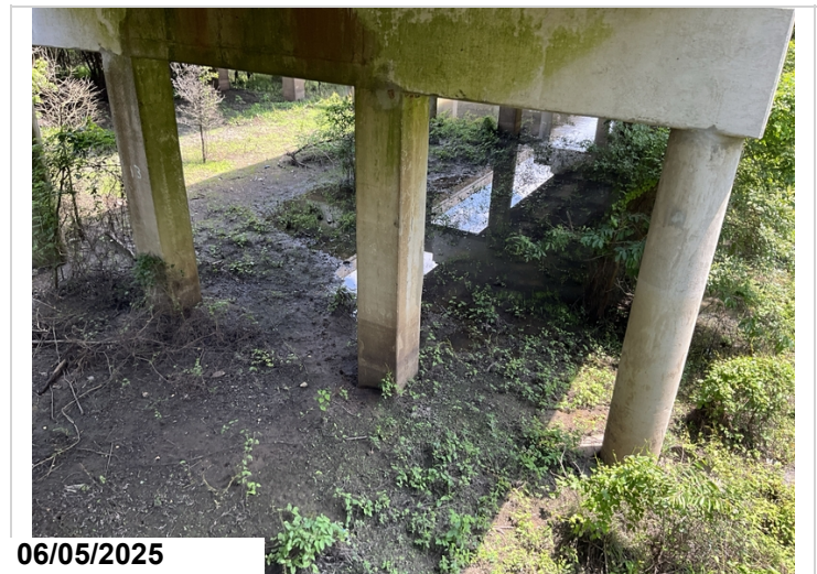
Bent 13, Column 3: Cracks and delaminations.
