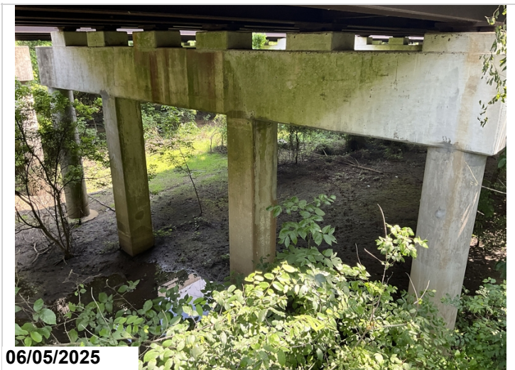
Bent 9, Column 3: Cracks and delaminations.
