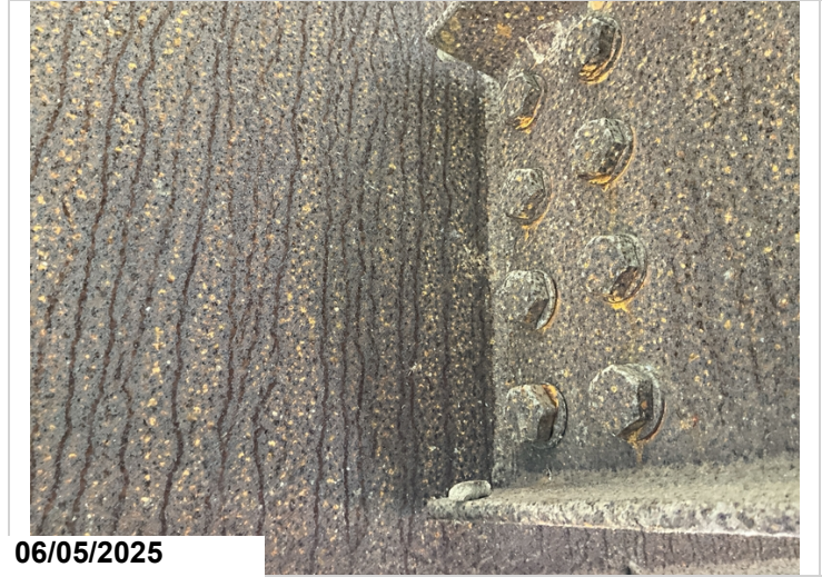
Typical diaphragm bolt loose.
