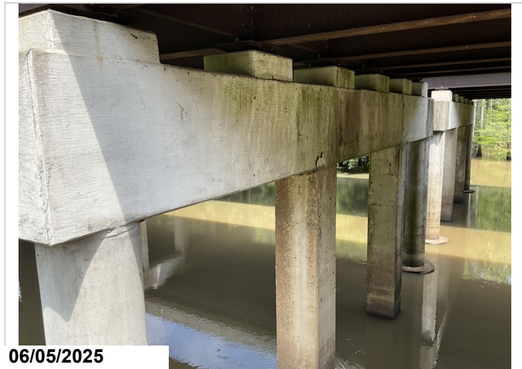
Cap, Bent 6, Ahead, Above Columns 2 & 3: 1' cracks with delaminations each location.
