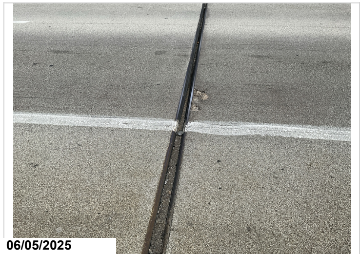
Deck, Span 9, Ahead Of Bent 8 joint: 1' wide spall no exposed reinforcing steel.
