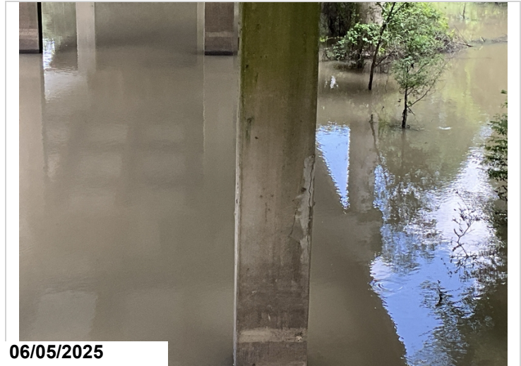
Bent 20, Column 3, Back, Right, Corner: Cracked for 3'.
