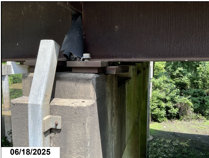
Span 8, Bent 8, Bearing 6: Bearing pad has sild half way out from under girder.
