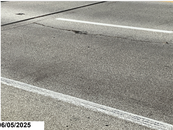
Abutment 2, Approach Slab: Several cracks reflecting through the epoxy coating.
