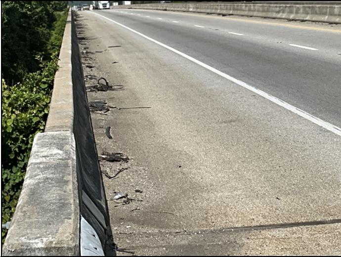
Typical debris in gutters
