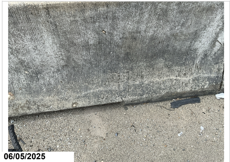
Bridge Rails, Full Length: Vertical cracks spaced 2' apart half with efflorescence and one longitudinal crack full length 3" down from top.
