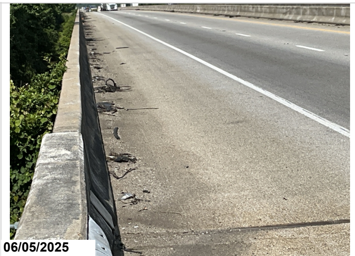
Typical debris in gutters
