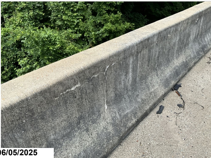
Bridge Rails, Full Length: Vertical cracks spaced 2' apart half with efflorescence and one longitudinal crack full length 3" down from top.
