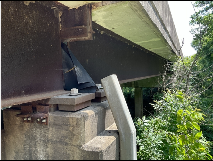
Joint Trough, Bent 8, Right: Last 3' failed.
