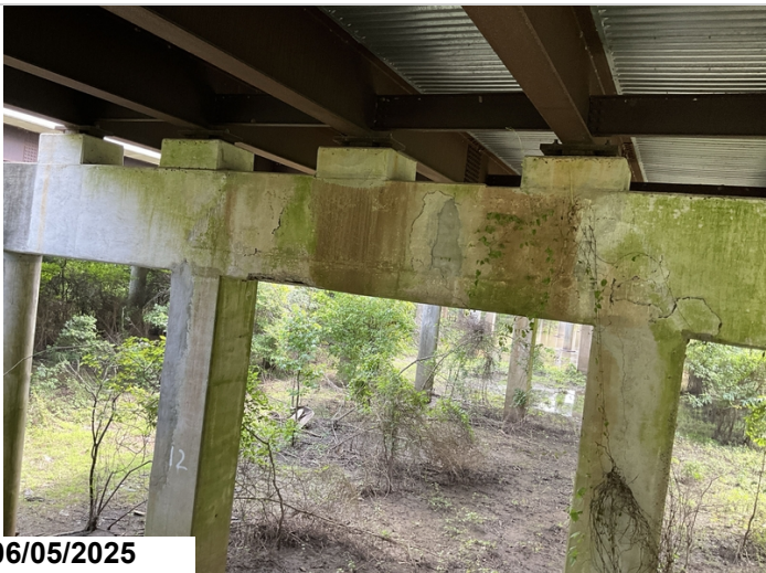
Cap, Bent 12, Bottom, Between Columns 2 & 3: 2' Cracks with delaminations.
