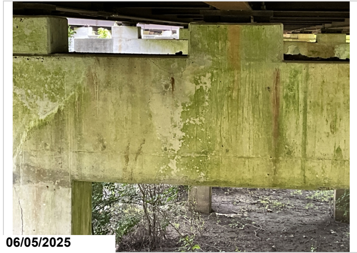
Cap, Bent 11, Back, Under & To Left Of Girder 3: 3' cracks with delaminations.
