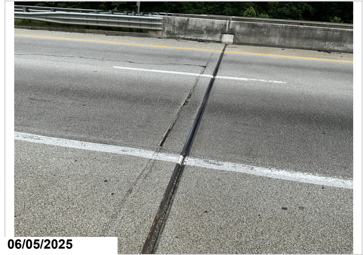
Abutment 1 joint
