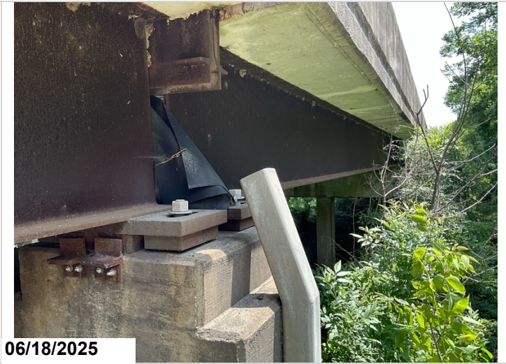
Joint Trough, Bent 8, Right: Last 3' failed.
