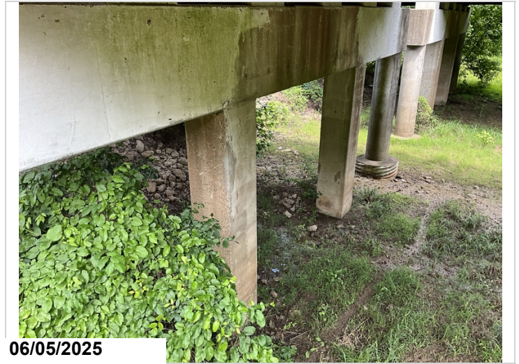
Bent 2, Column 3: Cracks and delaminations.
