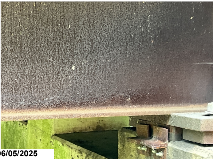
Typical active corrosion on girders.
