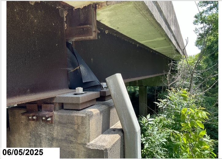
Joint Trough, Bent 8, Right: Last 3' failed.
