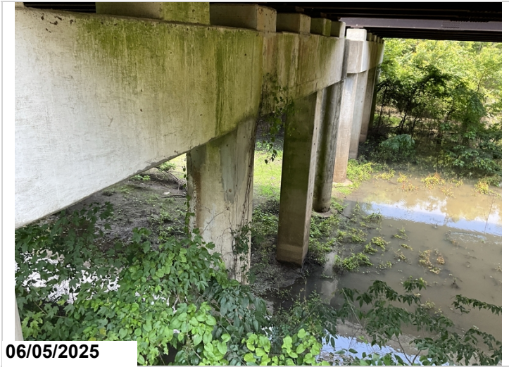
Bent 14, Column 2 & 3: Cracks and delaminations.
