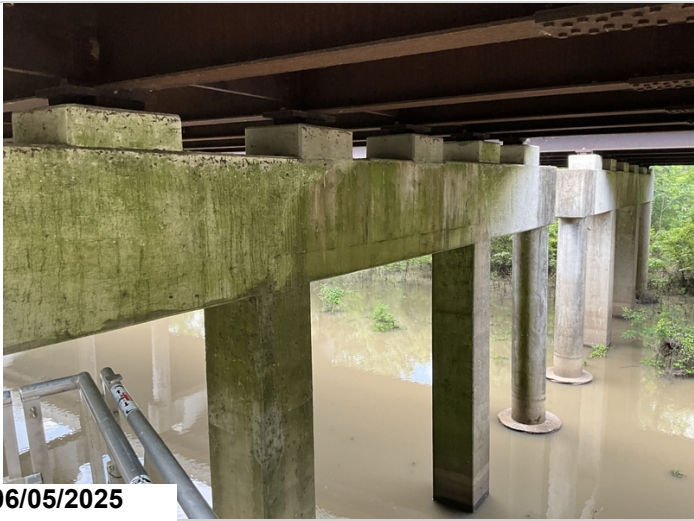
Cap, Bent 19, Ahead, Above Column 2: 1' cracks with delamination.
