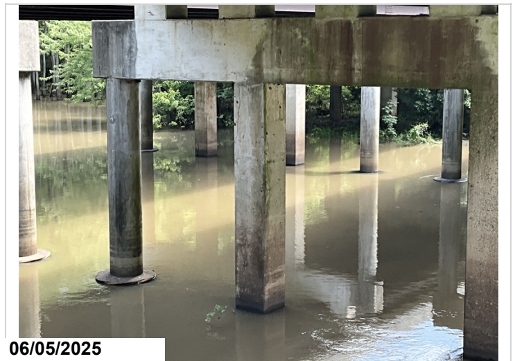
Bent 6, Column 2: Cracks and delaminations.
