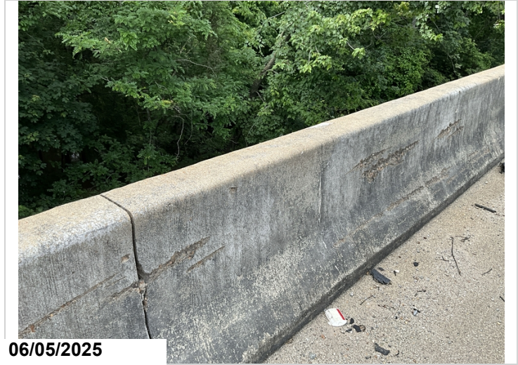
Span 16, Bridge Rail, Right: 10' long area of impact damage.
