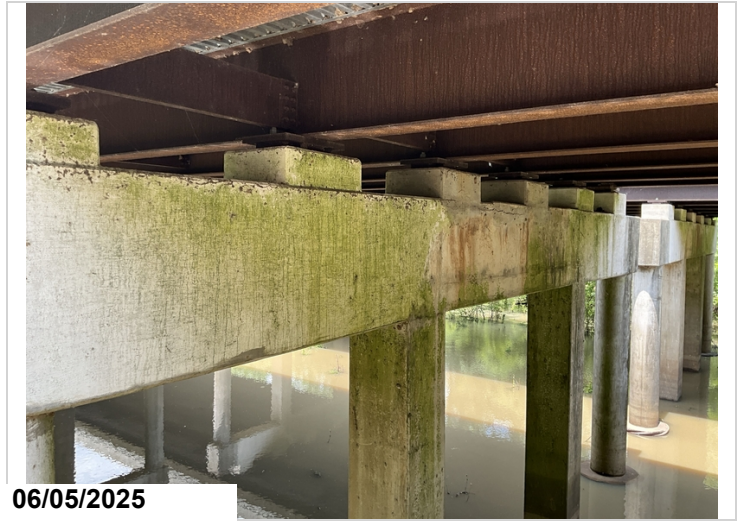
Cap, Bent 18, Ahead, Top, Between Girders 3 & 4: 4' cracks with delamination, and a 5' long crack.
