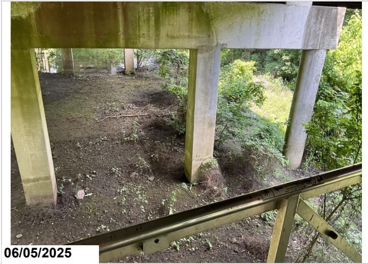
Bent 10, Column 2: Cracks and delaminations.
