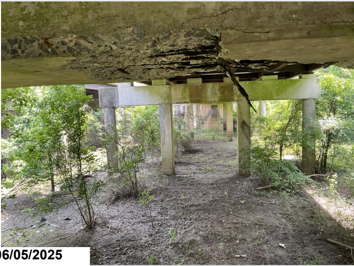
Cap, Bent 11, Bottom, Between Columns 2 & 3: 5' of spalls exposed reinforcing steel with moderate to heavy section loss.
