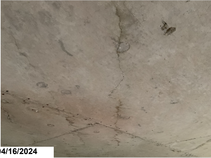
Typical soffit / undersurface of deck crack with rust stains
