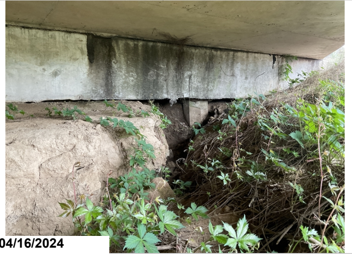
Abutment 1, cap: slope eroded at pile 2 for 4' up to 2' deep, exposing pile 2.
