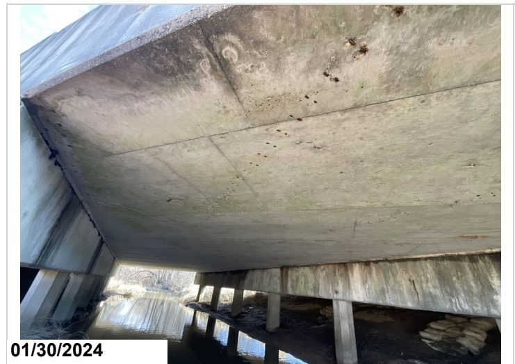
Span #2 soffit / underside of deck
