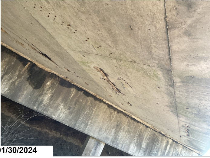
Span #2 soffit left side spalled with exposed rebar
