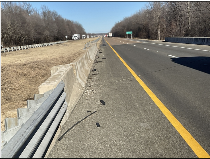
Dirt and debris in gutters
