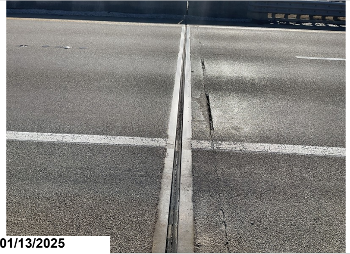
Abutment 1, joint: seal has lost adhesion for 10' with minor sagging.
