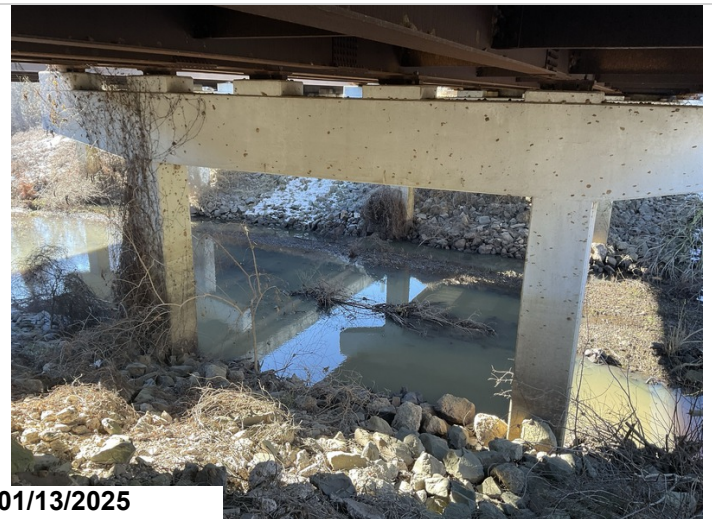
Vegetation growing on bent 3 and beside and under bridge.
