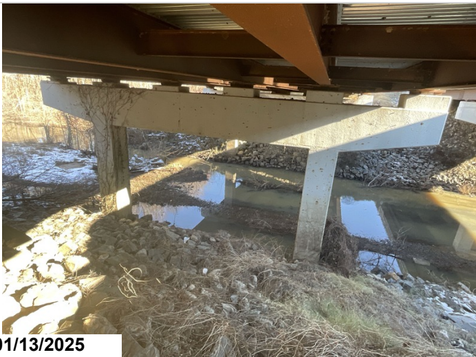
Vegetation growing on bent 2 and beside and under bridge.
