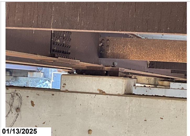
Bent 3, Girder 4, anchor bolt: loose nut.
